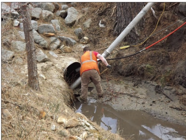
Fig. 2-1. Crews clean a culvert.
