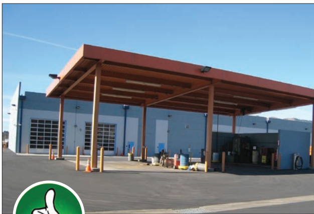
Fig. 3-13. Whenever feasible, wash rack areas and fuel points should be covered.
