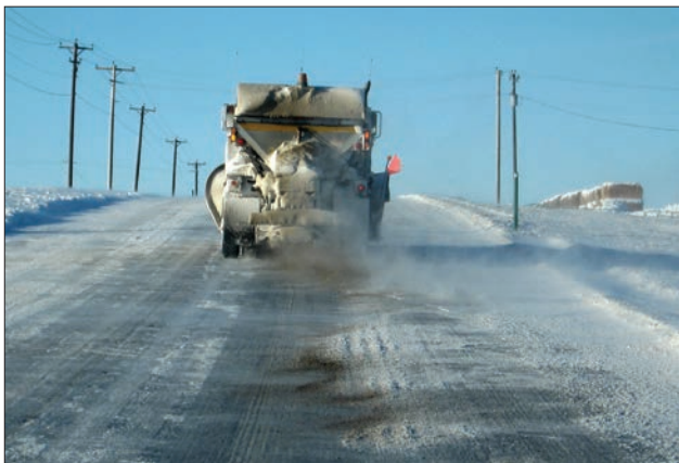
Fig. 2-10. Snow removal helps maintain a clear vehicular path of travel. Sand and salt applied to the roadway can be transported offsite and impact stormwater quality. Source: Idaho Transportation Department
