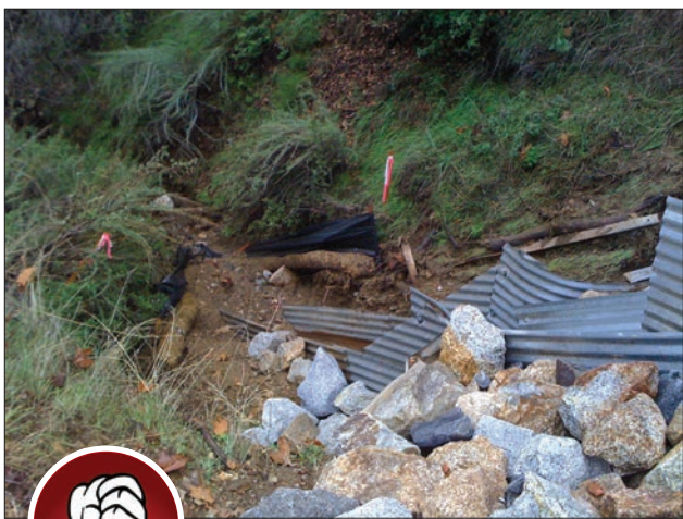
Fig. 2-2. Failure to provide routine maintenance at pipe outfalls can lead to larger failures.
