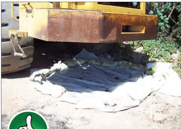
Fig. 3-9. The gravel bags and tarp being used here offer effective containment of possible leaks.
