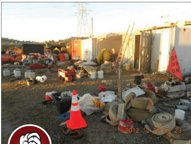
Fig. 3-2. Stored materials should be organized and placed within containment areas when not in use.
