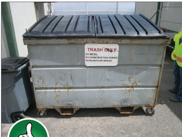
Fig. 3-5. Providing lids on trash bins is an easy way to prevent wind dispersal and contact with stormwater. Signs are advisable to limit contents.
