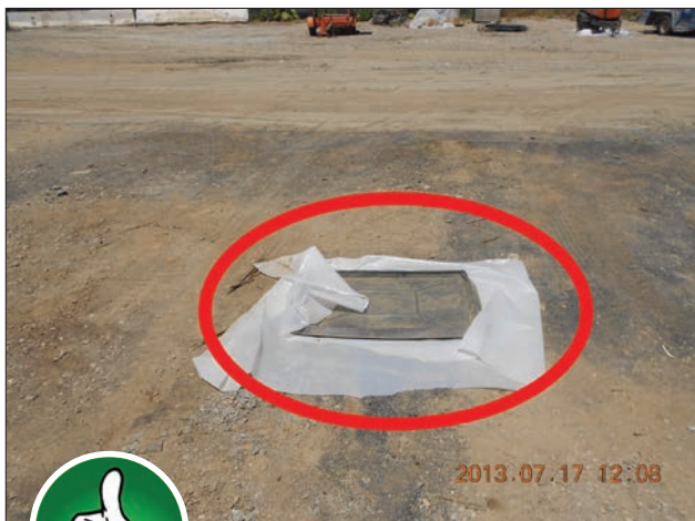
Fig. 3-7. A basic drip pan is shown here for use in collecting drip leaks.
