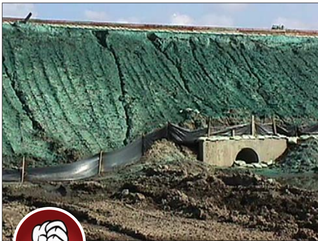
Fig. 2-7. The binder used in this situation requires a greater application rate, as visibly evident by signs of rill erosion.
