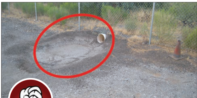
Fig. 5-25. Conditions near this outfall will create a condition of standing water and a potential for mosquito breeding. Source: RBF Consulting
