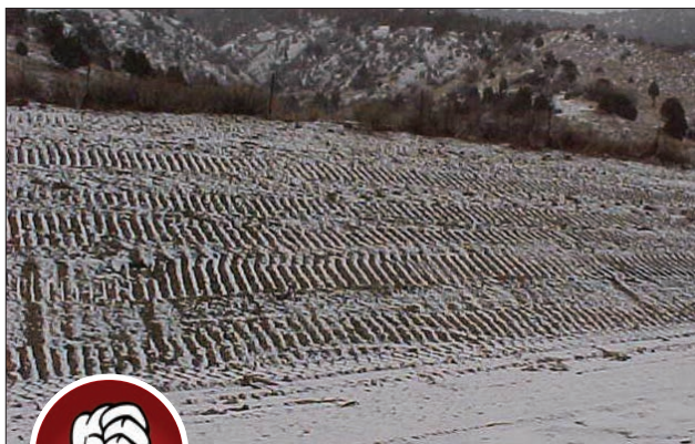
Fig. 4-2. Track walking in the wrong direction increases rilling and erosion.
