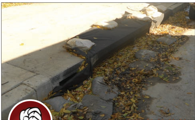
Fig. 5-11. Gravel bags shown here are crushed, allowing leaves and other debris to build up. The filter fabric should not be used in this application.
