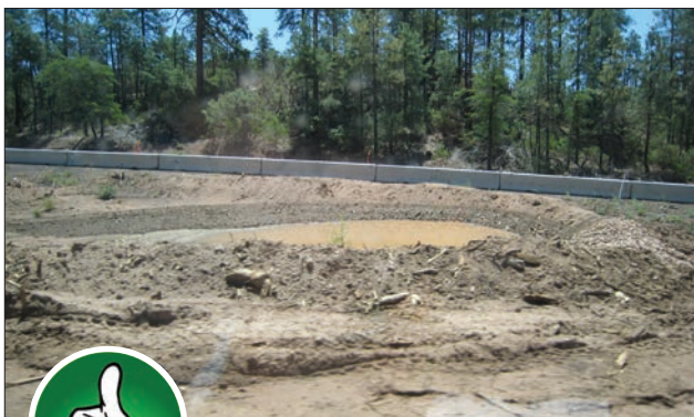
Fig. 3-19. A typical installation of sediment trap is shown. Notice there are no signs of overflow, spot failures, or scour.
