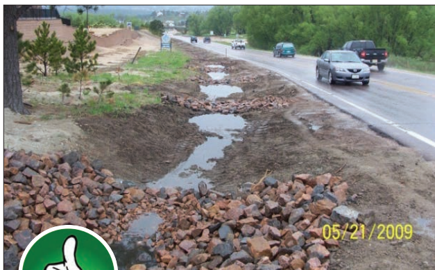
Fig. 5-20. This shows effective containment of water behind check dam and controlled spillover through the middle. Source: Colorado DOT
