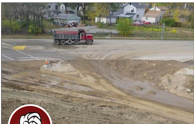
Fig. 3-11. A stabilized construction entrance is needed to prevent tracking of sediment offsite. Source: Ohio DOT
