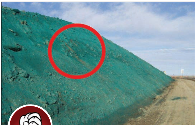
Fig. 4-12. This is a poor example of a spray-on mulch. There is uneven coverage and holes/uncovered areas. Source: Colorado DOT
