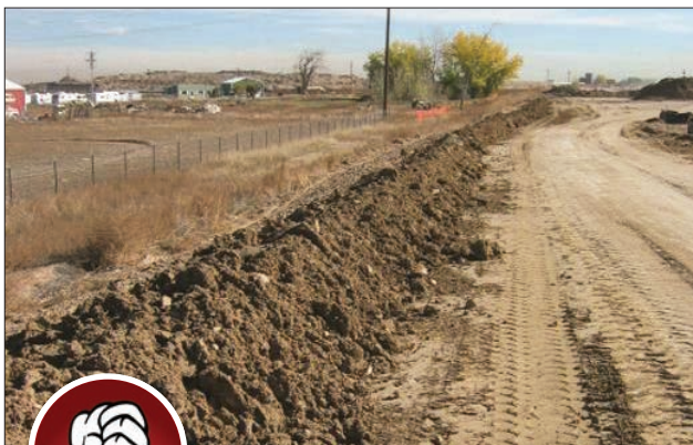
Fig. 5-7. This berm is not compacted.
