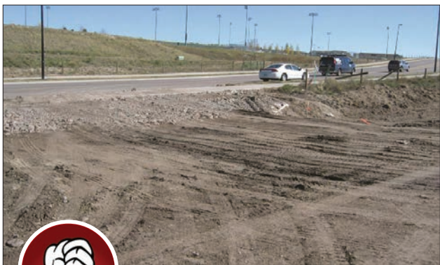
Fig. 3-6. This is a poor installation of a construction entrance. It lacks perimeter controls.
