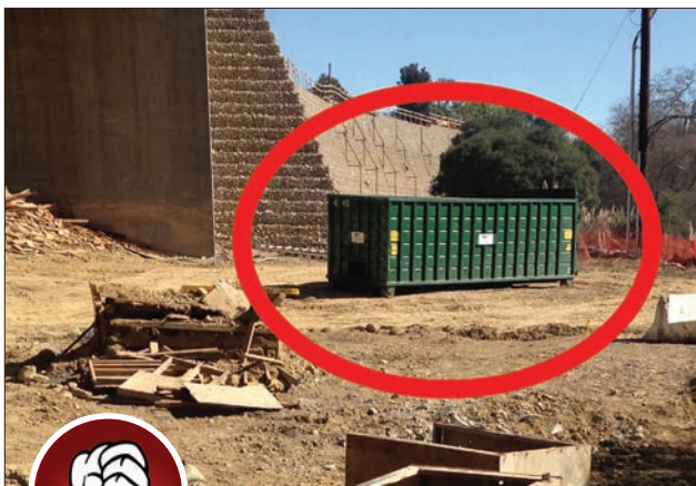
Fig. 2-5. Leaving trash dumpsters uncovered is among the most typical mistakes on construction sites.
