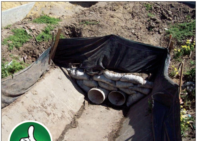
Fig. 5-2. A BMP configuration of silt fence and gravel bags helps stabilize this temporary drainage crossing.
