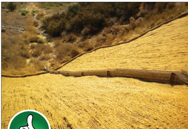
Fig. 5-17. This is an excellent example of a slope drain being used as an effective erosion control.
