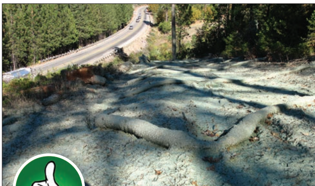
Fig. 4-9. Hydroseeding of large slopes is always more effective when done in combination with sediment control measures such as the fiber rolls shown here. Source: RBF Consulting
