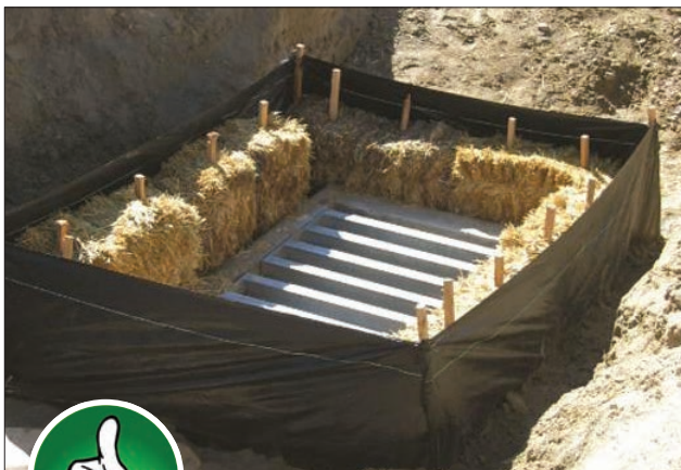
Fig. 5-12. This is a good installation of inlet protection using silt fence and straw bales.
