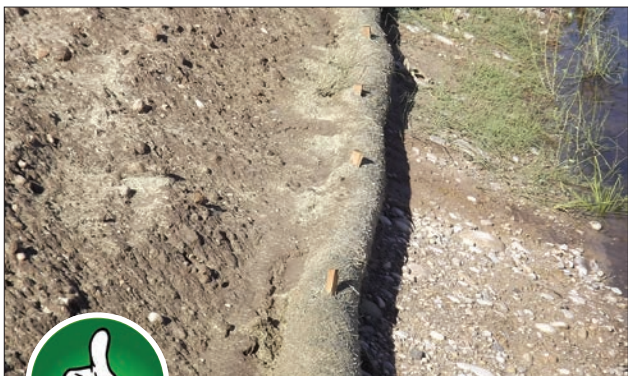
Fig. 3-9. This wattle is clearly trapping sediment, although removal of trapped sediment is required to maintain effectiveness.
