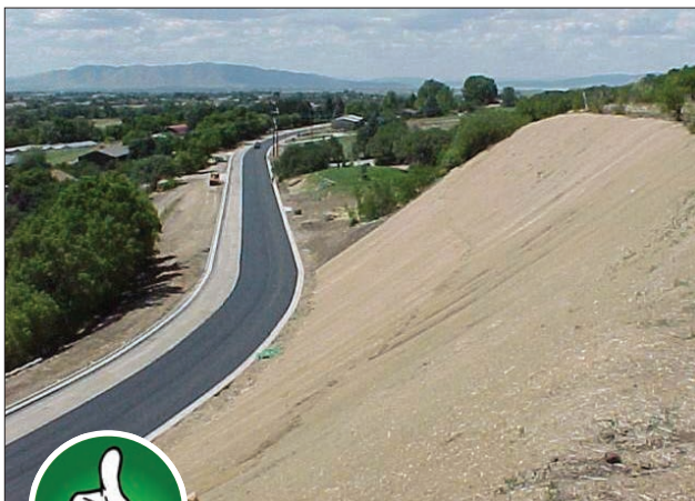
Fig. 4-15. RECPs are an effective way to provide immediate stabilization to steep slopes.
