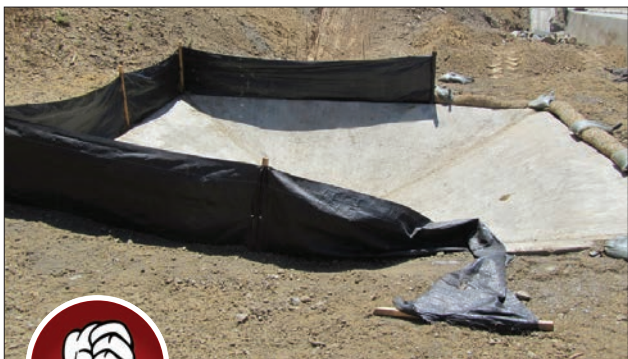
Fig. 5-10. Proper installation of stakes is critical to the performance of inlet protection measures such as silt fence. Also silt fence should not be placed in the path of concentrated flow, as shown here.
