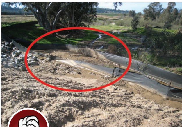
Fig. 1-10. Establishing responsibility for regular inspection and maintenance of stormwater BMPs is an important part of work and communication management key to preventing failures as show here. Source: RBF Consulting
