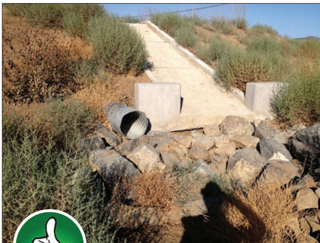
Fig. 5-24. A typical application is shown using riprap for erosion protection at a storm drain outlet. Source: RBF Consulting
