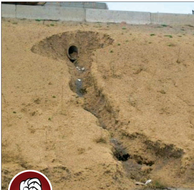
Fig. 5-16. The slope has eroded. This could have been prevented with the use of a slope drain.
