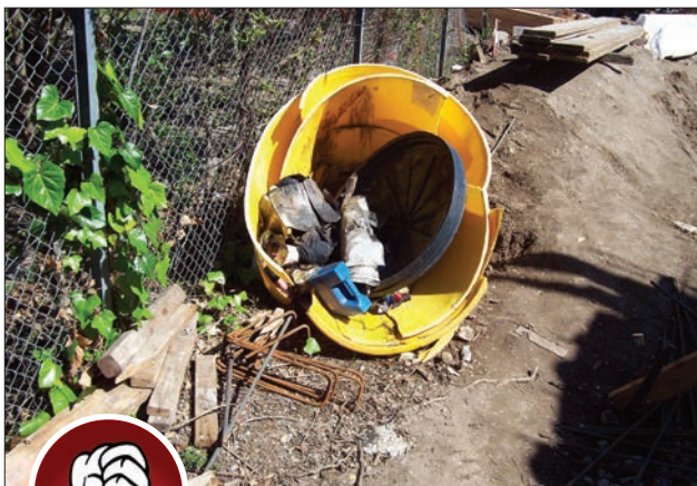
Fig. 2-12. Workers overlook placement of small amounts of waste material such as this in proper disposal areas.
