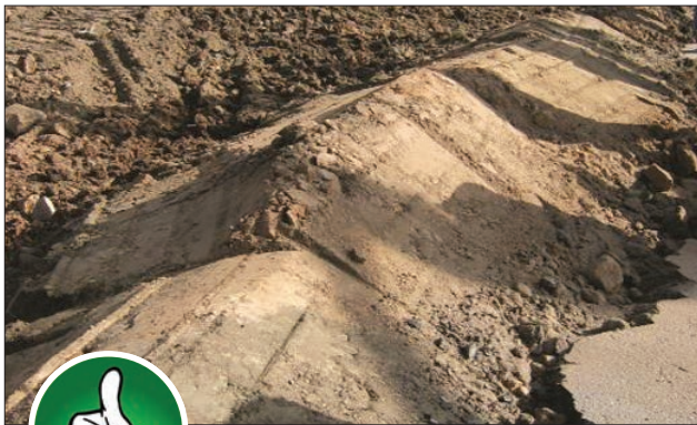
Fig. 5-6. This is an excellent berm. There are no breaks in the berm and the soil is compacted.
