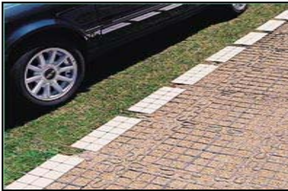
Figure 6.4.17 – Permeable pavement. Source: Connecticut, 2004.
