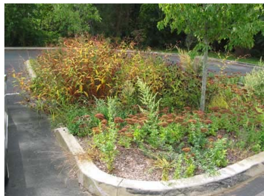
Figure 6.4.15 – Bioretention in use as a parking lot island in Branford, CT. Source: Connecticut Department of Environmental Protection.
