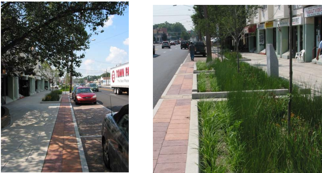
Figure 6.3.12 – Permeable pavement (left photograph) and rain garden/bioretenion (right photograph) retrofits along North Main Street in Bridgeport, CT.
