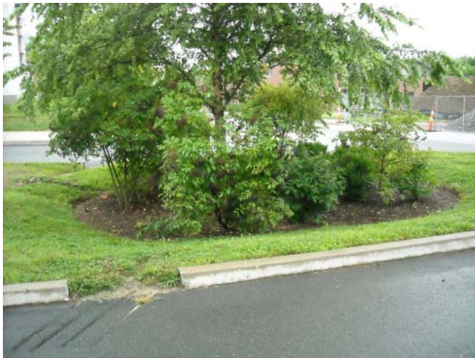
Figure 6.4.28 – Bioretention at University of Connecticut Storrs Campus –Mansfield, CT. Source: Connecticut Department of Environmental Protection.
