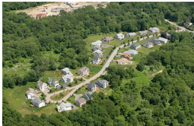
Figure 6.4.8 – Alternative roadway design in Waterford, CT. Source: Tom Walsh, Shoreline Aerial Photography
