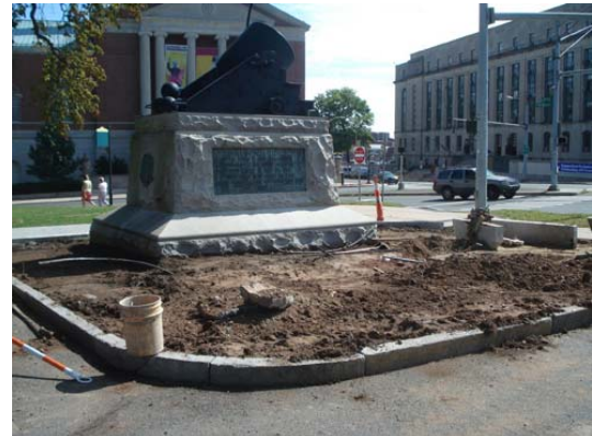
Figure 6.3.14 – Construction of a rain garden at Hartford Green Capitols Project. Source: Camp Dresser & McKee.
