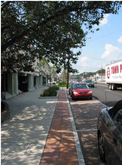
Figure 3.12 – Permeable pavement (left photograph) and rain garden/bioretention (right photograph) retrofits along North Main Street in Bridgeport, CT.
