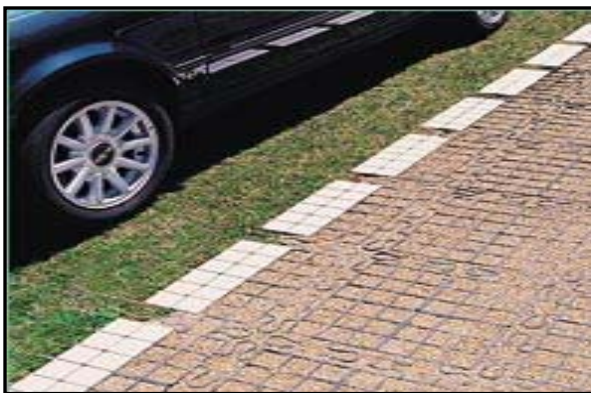
Figure 4.15 – Permeable pavement. Source: Connecticut, 2004.
