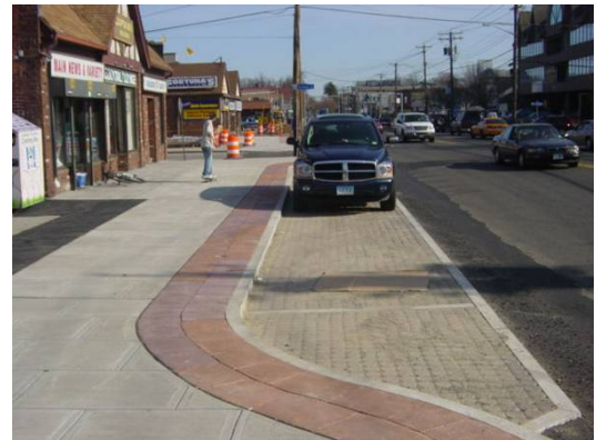
Roads are narrowed and permeable pavement is installed along roadways to provide additional parking and treat runoff.
