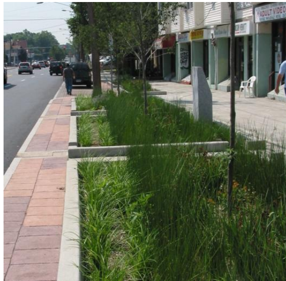
Figure 3.12 – Permeable pavement (left photograph) and rain garden/bioretention (right photograph) retrofits along North Main Street in Bridgeport, CT.
