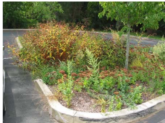
Figure 4.13 – Bioretention in use as a parking lot island in Branford, CT. Source: Connecticut Department of Environmental Protection.
