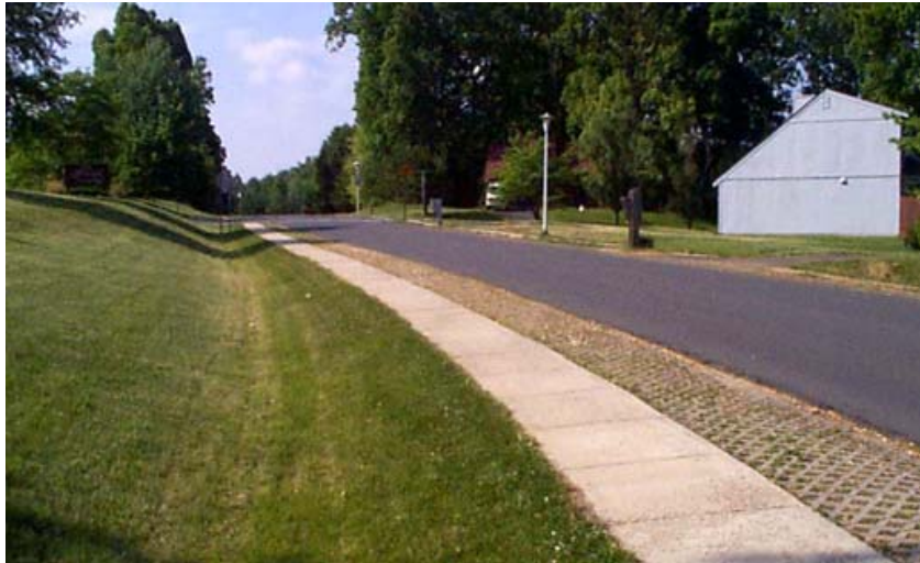
Figure 3.5 - Narrow low-volume road section with sidewalks, shallow swale and porous pavement shoulders.
