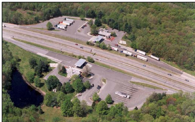
Example of inadequate truck parking along I-395 in Plainfield
