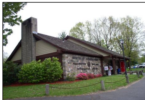
Rest area in Danbury, CT
