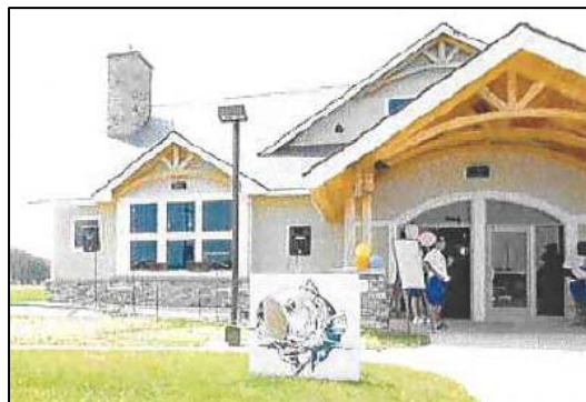
This rest area along I-371 SB in Brainerd Lakes, MN, constructed in 2005, features interpretive monuments and regionally inspired statues
