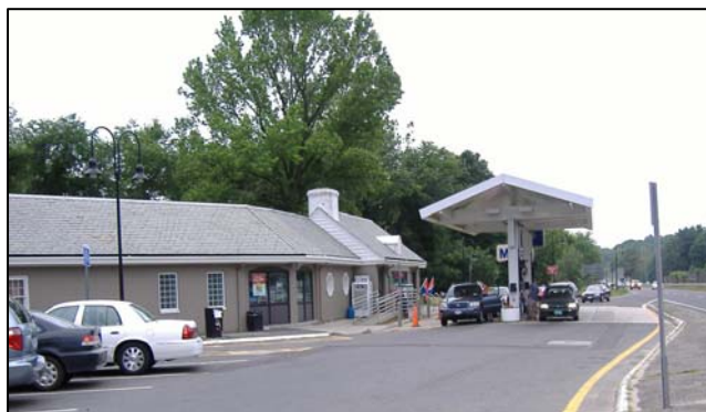
Service plaza along Merritt Parkway (Route 15)
