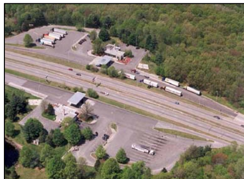
Truck parking on service plaza ramps along I-395 in Plainfield
