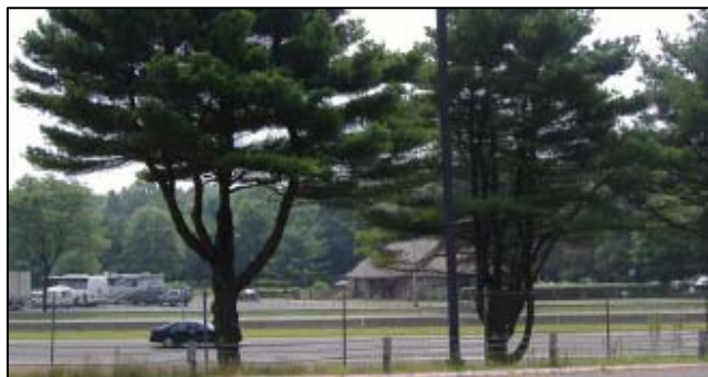
Rest area along I-84 EB in Willington
