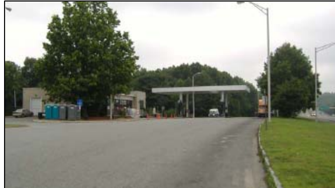
Service plaza along I-395 SB in Plainfield
