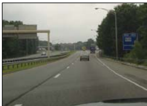
Lighter traffic volumes observed along I-395 (SB) approaching Plainfield service plaza
