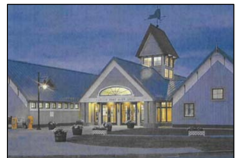
This Rest Area along I-87 NB in Clifton Park, NY was expanded and improved in 1997
