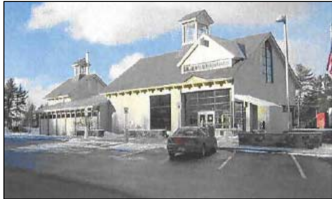
This information center on I-89 NB in Williston, VT, was reconstructed in 2002 and served nearly 382,000 visitors in 2005.
