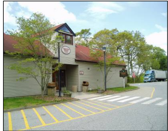
Welcome Center along I-95 NB in Westbrook, CT
