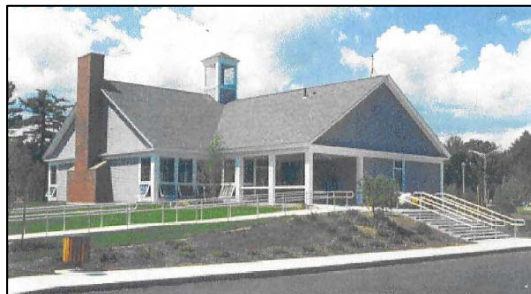
Welcome Center along I-95 in Seabrook, NH
