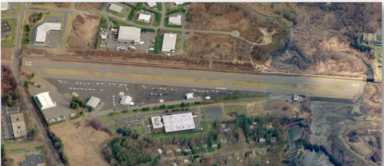
Figure 7-13. Aerial Photograph of Robertson Airport
