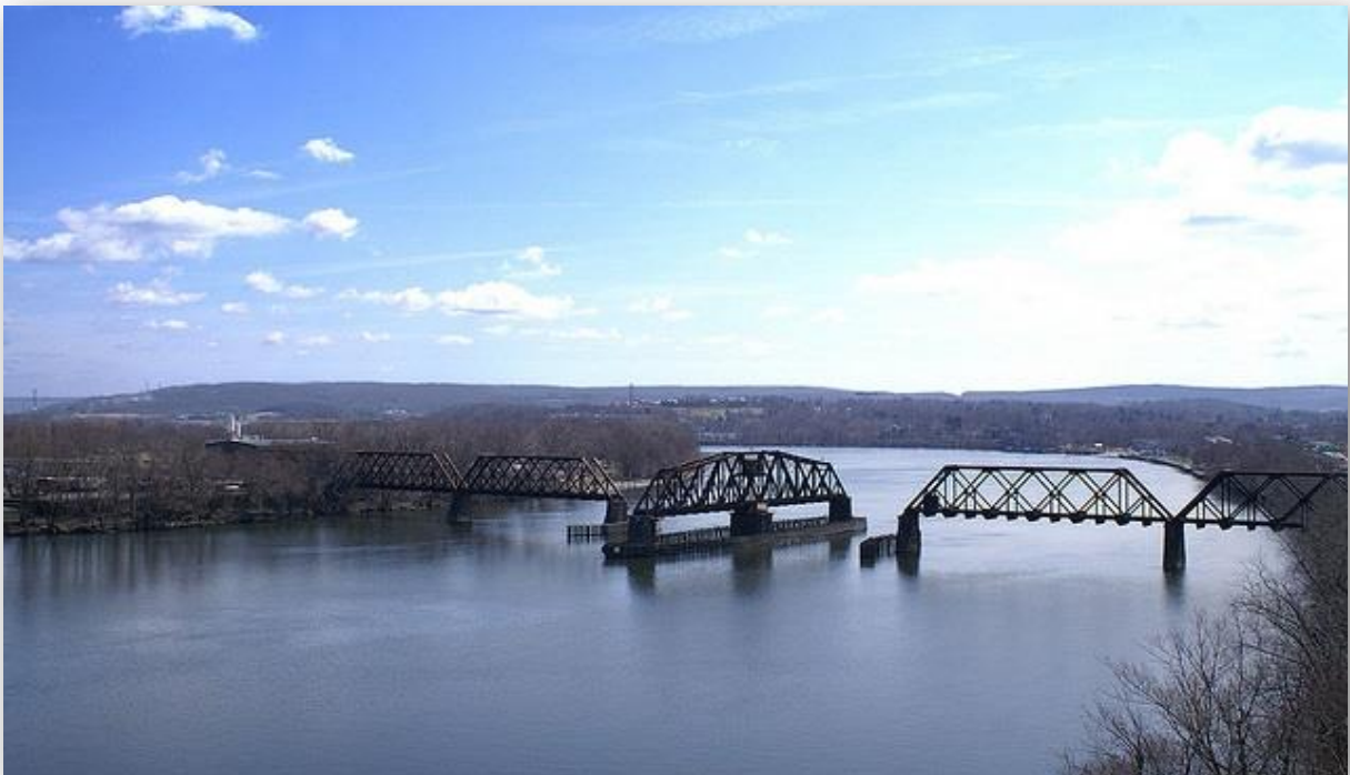
Figure 5-14. Railroad Swing Truss Bridge, Middletown CT
