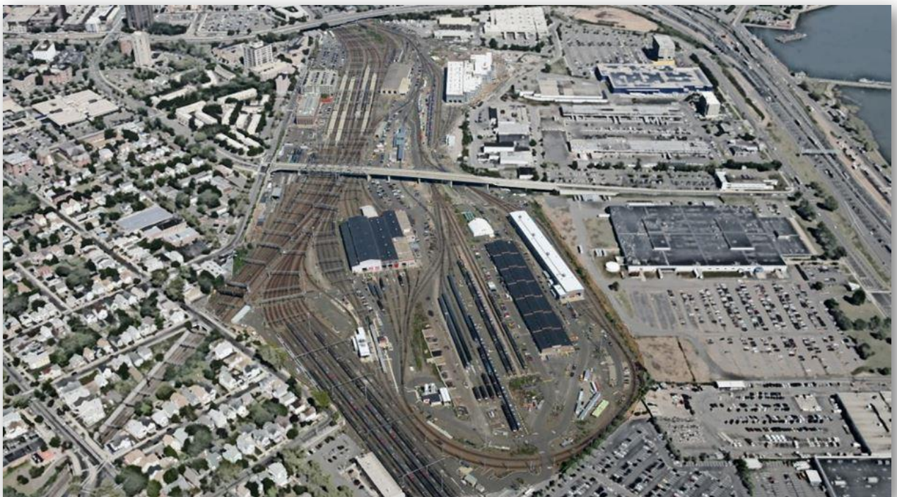
Figure 5-10. Union Station and New Haven Rail Yard, New Haven, Connecticut
