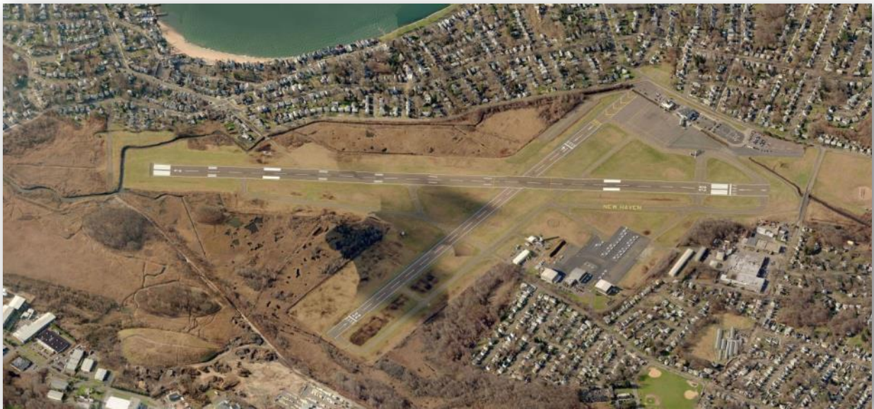
Figure 7-11. Aerial Photograph of Tweed-New Haven Airport
