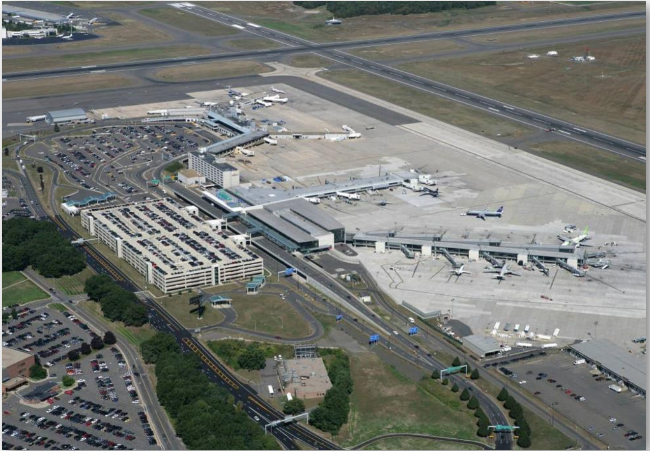
Figure 7-2. Aerial Photograph of Bradley International Airport
