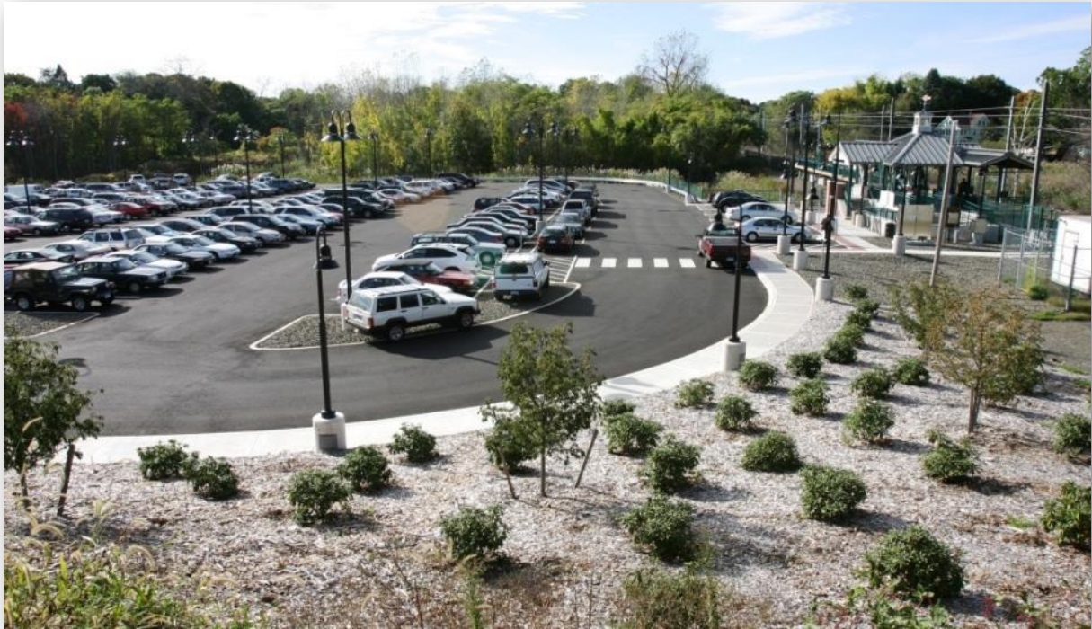
Figure 5.3. Parking Facility at Railroad Station in Branford, Connecticut
