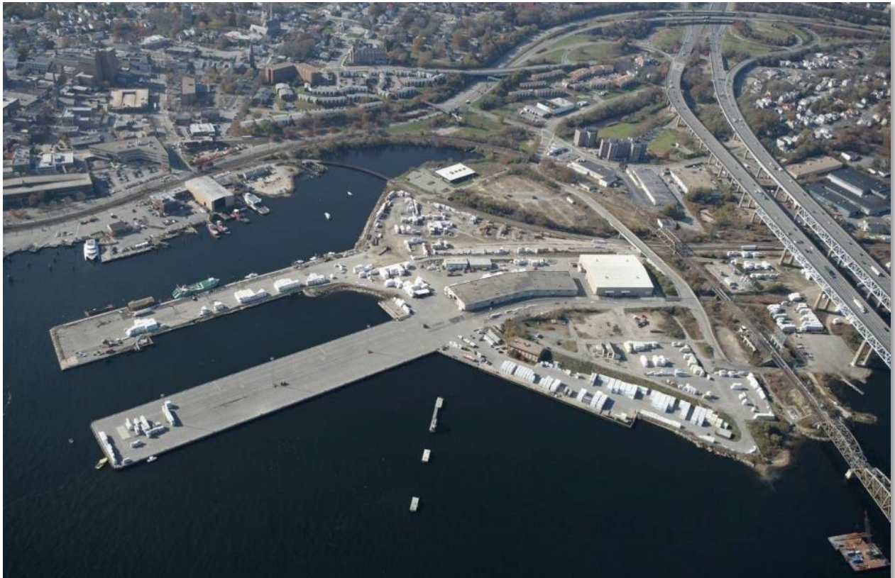
Figure 6-4. Aerial View of the State Port Complex, New London
