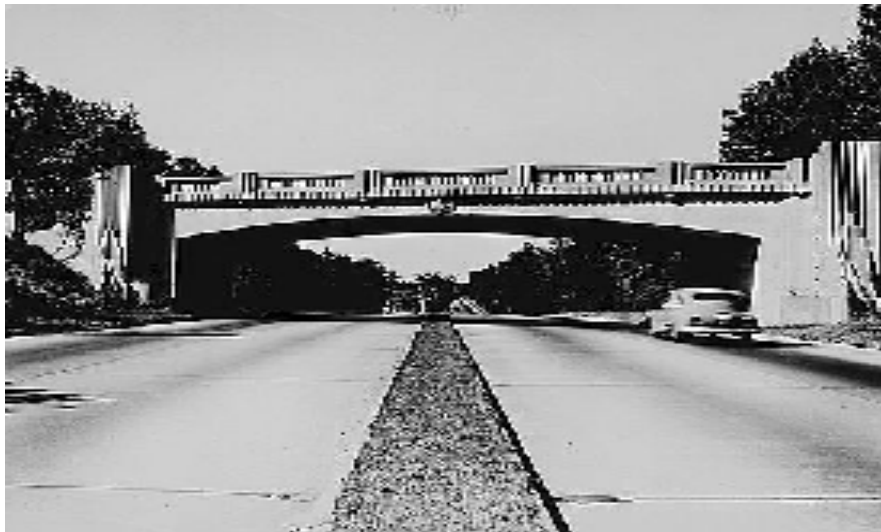
East Rocks Road over Merritt Parkway in Norwalk, CT ( www.nycroads.com/roads/merritt/ )
