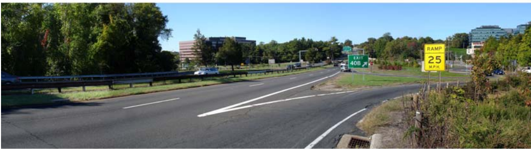
Figure 2: View Along Merritt Parkway Looking West
