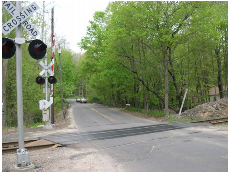
Figure 6: Seeley Road At Grade Crossing Looking West Toward Route 7
