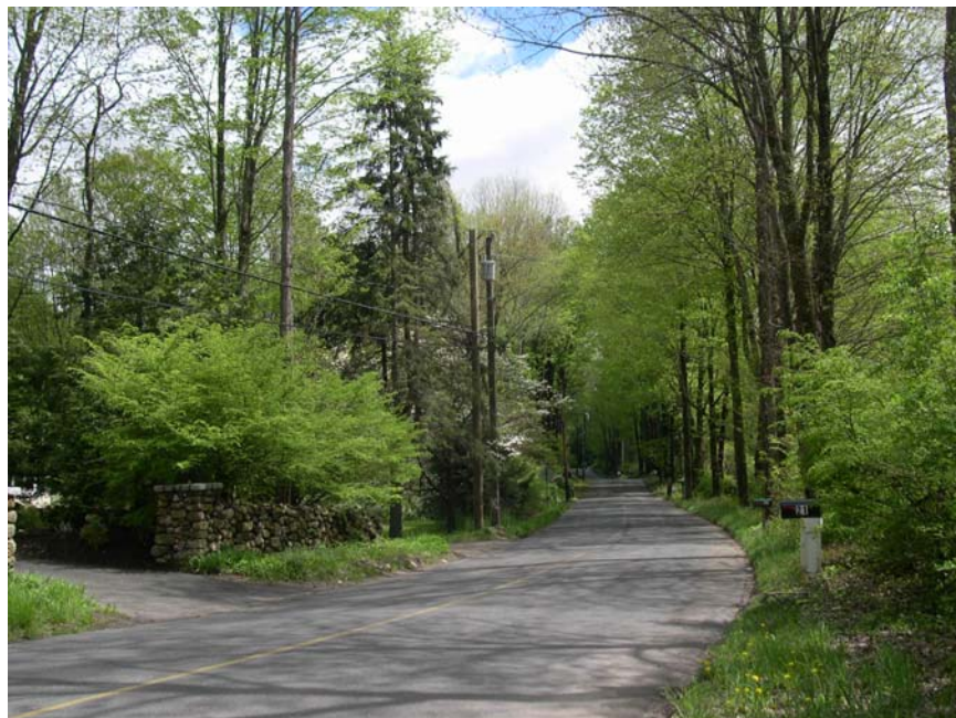
Figure 11: View Along Side Cut Road Looking North
