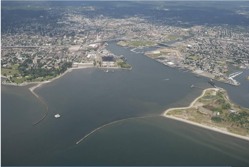
Figure 34. Port of Bridgeport – Bridgeport Harbor Photograph
