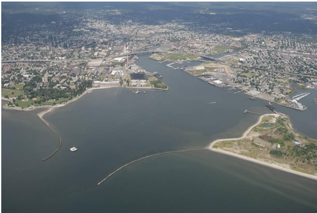
Figure 34. Port of Bridgeport – Bridgeport Harbor Photograph
