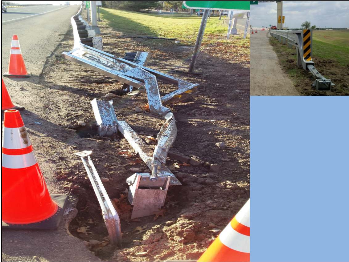
- Crash results of SoftStop Trial Installation
