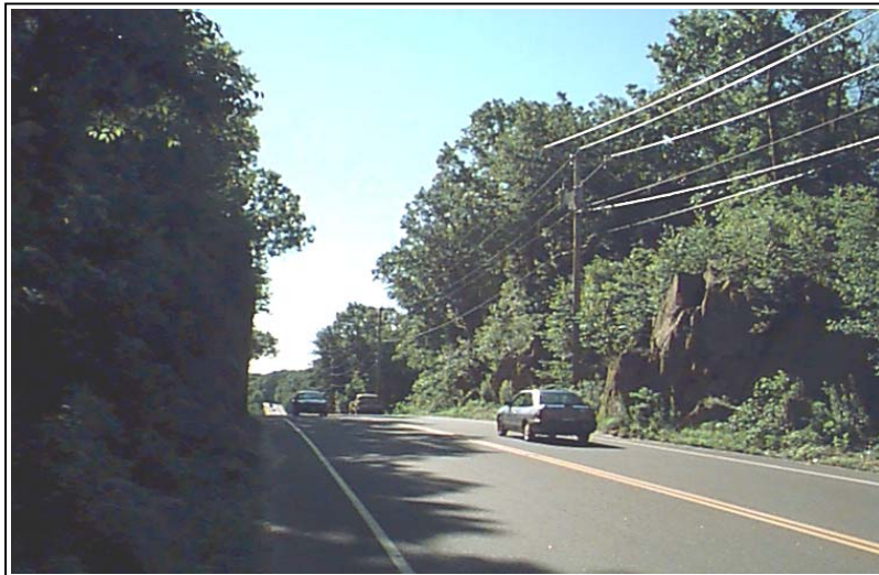
View of Route 64 with limited sight distance and rock ledge on both sides of the roadway
