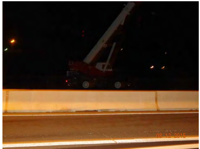
I-84 EB: The Contractor's crane stored on the side of the highway behind T.P.C.B.Cs.
