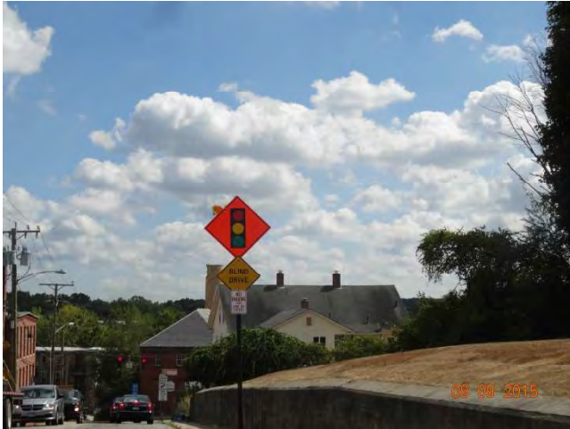
Church Street SB: Approaching the intersection with Pomfret Street (Route 44), a construction sign with a warning light is mounted on an existing advisory sign pole. It depicts a temporary signal ahead.
