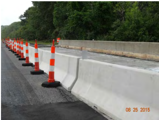
Route 11 SB: The bridge structure behind TPCBC and traffic cones.
