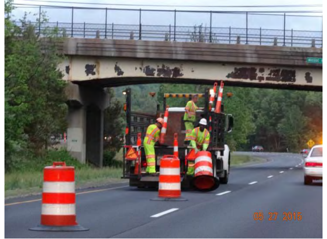
EB: A crew working setting up the traffic pattern
