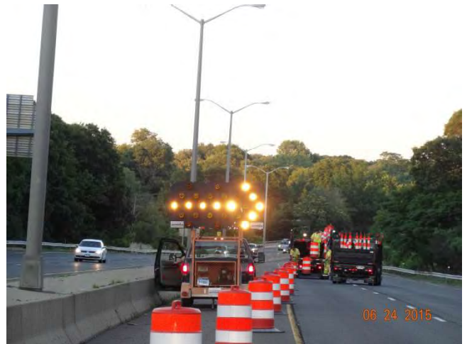
I-95 NB: A portable advance flashing arrow within the taper
