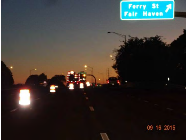
I-91 SB: The taper delineates across the closed lane to allow motorists to exit I-91 at Exit 7.
