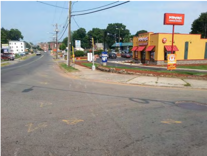
West Main Street EB: Existing sidewalk ramp on the north side of road.
