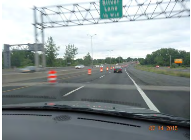
Route 15 NB: Traffic drums composing the taper.
