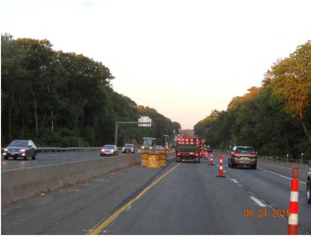
I-95 NB: A Type B Attenuation System with delineator on front
