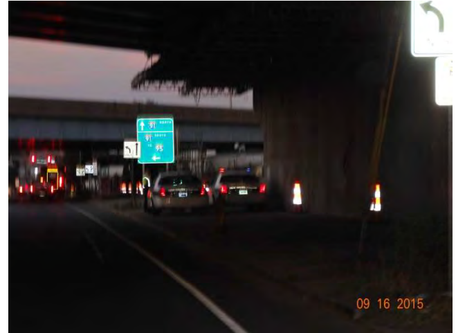
State Street (Route 5): Local police parked near the work area on State Street.
