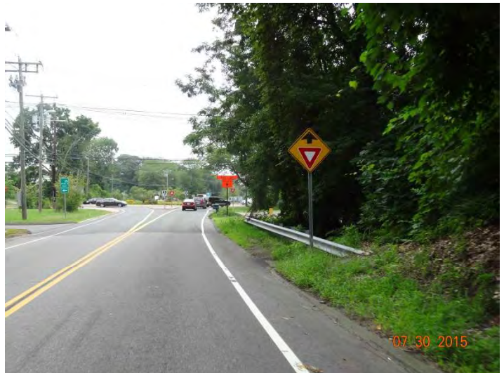
Route 80 EB: A Route 148 detour sign at entrance of roundabout.
