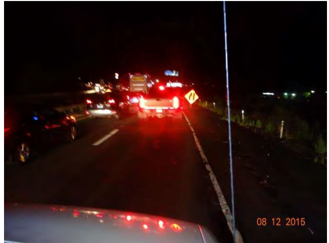
I-84 EB: A merge right construction sign.
