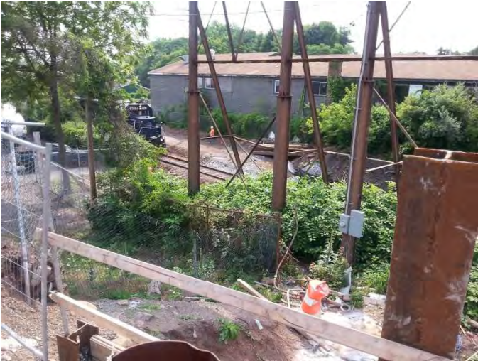
Burritt Street: The commercial train coming through the project site.
