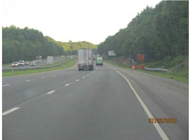
I-84 WB: A better view of the proximity of the CMS to the highway.
