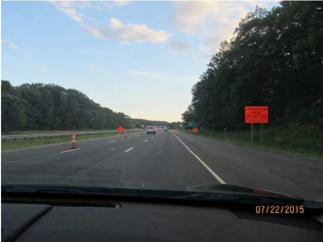
I-84 WB: A Legal Series 16 sign posted after the work zone began.
