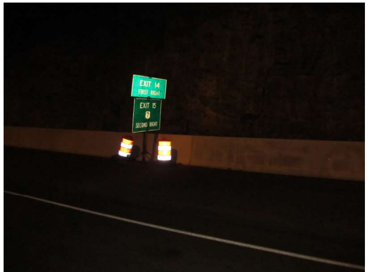
I-95 NB: Temporary exit sign for Exits 14 & 15 on a 7-foot sign post anchored/protected by two traffic drums.
