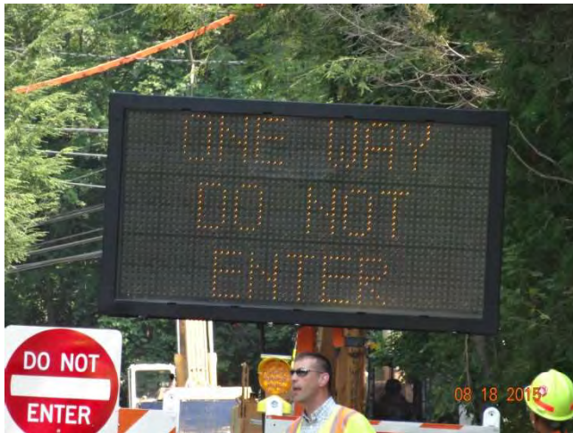
Old Mill Road NB: The second frame stating ONE WAY, DO NOT ENTER.
