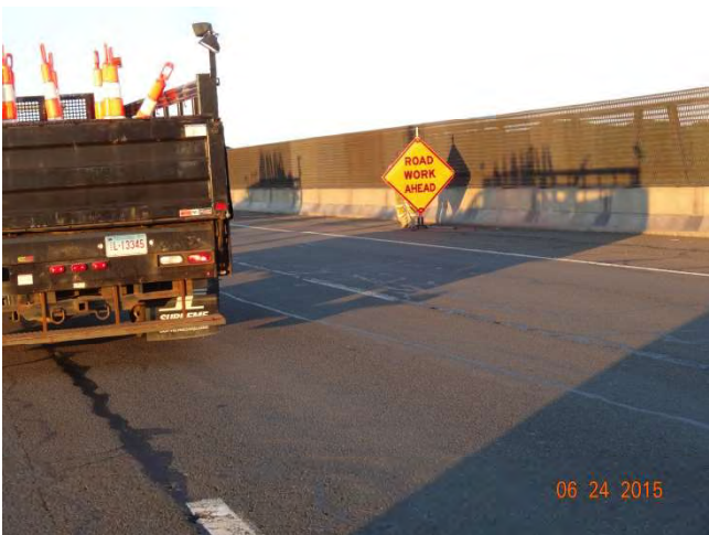
I-95 NB: "Road Work Ahead" sign
