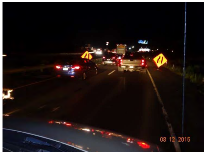
I-84 EB: Traffic bypassing two merge right construction signs on both sides of the road.
