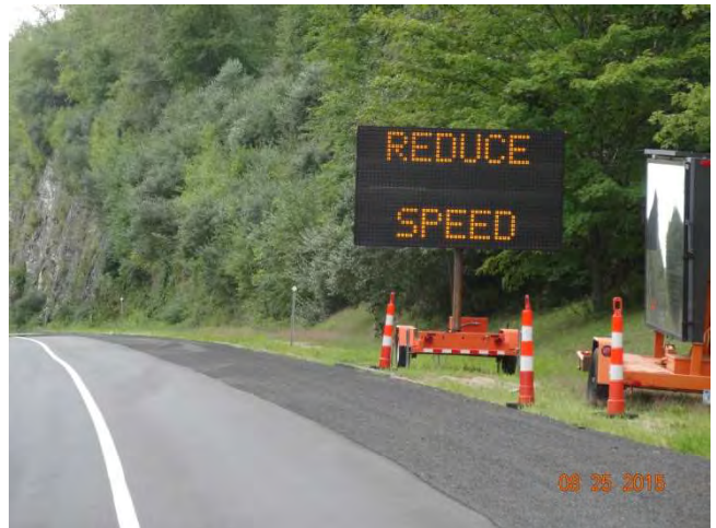
Route 11 SB: The CMS stating REDUCE SPEED on its second frame.
