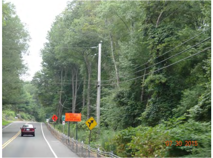
Route 79 SB: A sign saying ROUTE 148 CLOSED DETOUR AHEAD which is for this project and a behind it a signal light sign with warning light for the adjacent project.
