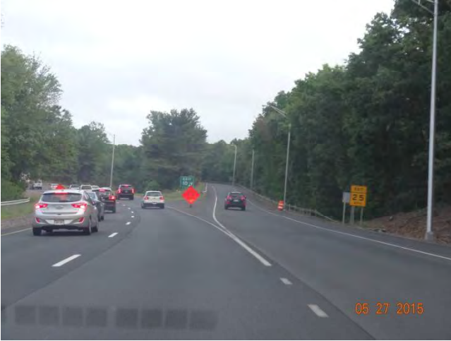
EB: The queue on the eastbound side while the traffic pattern is being set up
