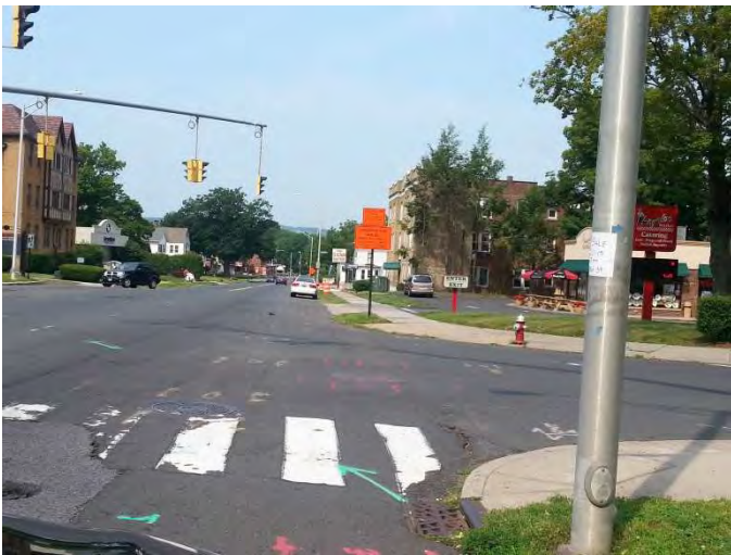
West Main Street EB: The Legal Series signs for Road Use Restricted and Sidewalk Use Restricted. The Road Use Restricted sign is a 16-M and should be a 16-H since it's on a state road.
