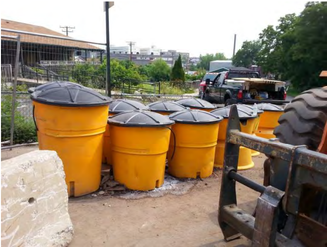
West Main Street: The Impact Attenuation System Type "A" at the west side of the bridge.
