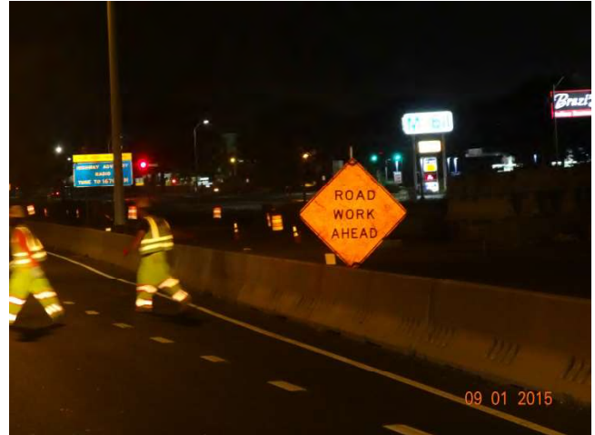
I-95 SB: The workers installed a temporary ROAD WORK AHEAD sign.
