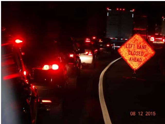
I-84 EB: A LEFT LANE CLOSED AHEAD construction sign. The sign reflectivity is marginal. Signs should be cleaned before placement to prevent motorists from not being able to see them or understand them.
