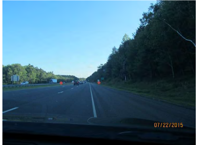
I-84 WB: Advance warning signs on both sides of highway.
