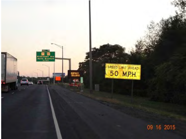
I-91 SB: A Changeable Message Sign (CMS) stating on its first frame EXPECT DELAYS placed behind the guide cables right before Exit 8.
