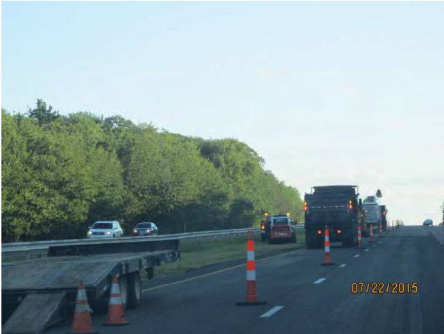
I-84 WB: The work crew paving in the closed left lane.
