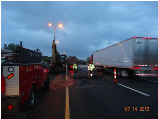
Route 15 NB: The inspection team looking at an open bridge joint.
