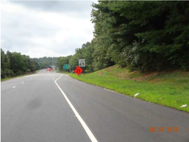
Route 11 SB: A temporary merge left sign with a warning light.
