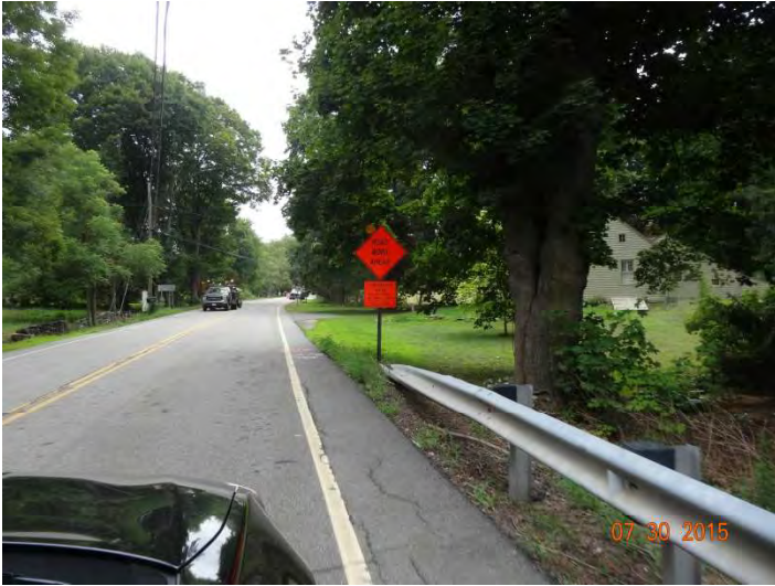
Route 148 EB: A ROAD WORK AHEAD sign with a low-intensity warning light attached and a legal series ROAD USE RESTRICTED sign.
