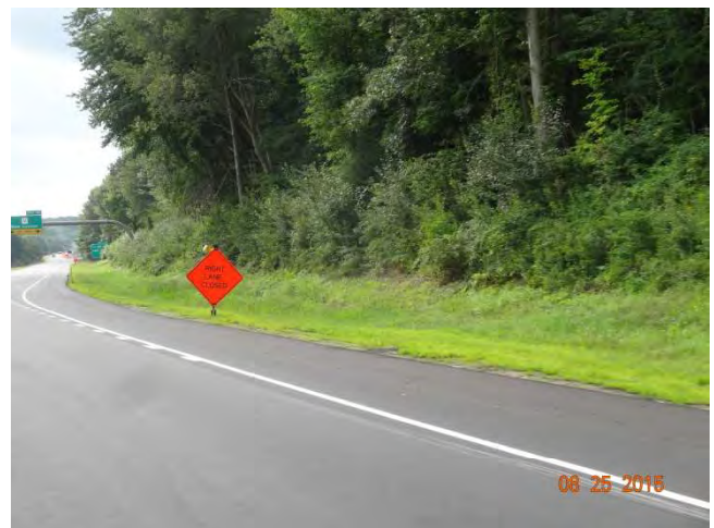
Route 11 SB: A temporary RIGHT LANE CLOSED sign with a warning light attached.
