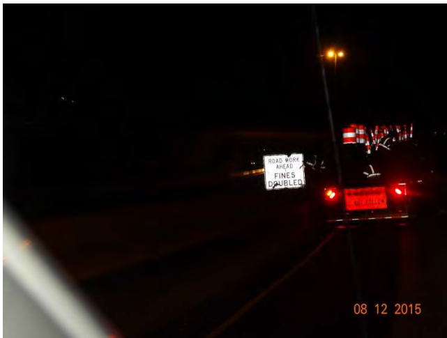
I-84 EB: The sign crew setting up a ROAD WORK AHEAD FINES DOUBLED sign on the left side of the road.
