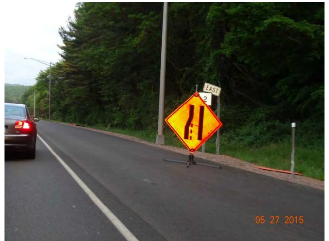
EB: More advance warning for the traffic queue
