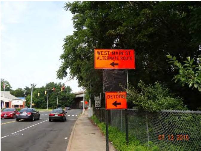
West Main Street EB: Signs advising motorists of the alternate route that can be used instead of traveling through the work zone. A DETOUR Sign is also being used to emphasize the alternate route but the signage can be confusing. The DETOUR sign should be covered up until the detour is being used.
