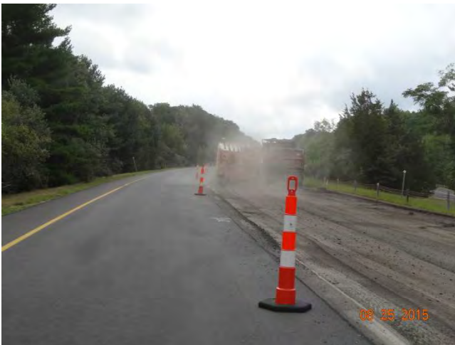
Route 11 SB: A sweeper cleaning the milled surface in the right lane.
