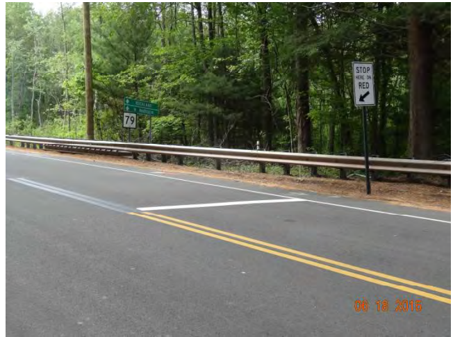
Route 79 SB: The stop bar with stop bar sign. The stop bar was moved back to accommodate the temporary signal being hard wired. Black out tape was used to cover over the existing pavement markings.
