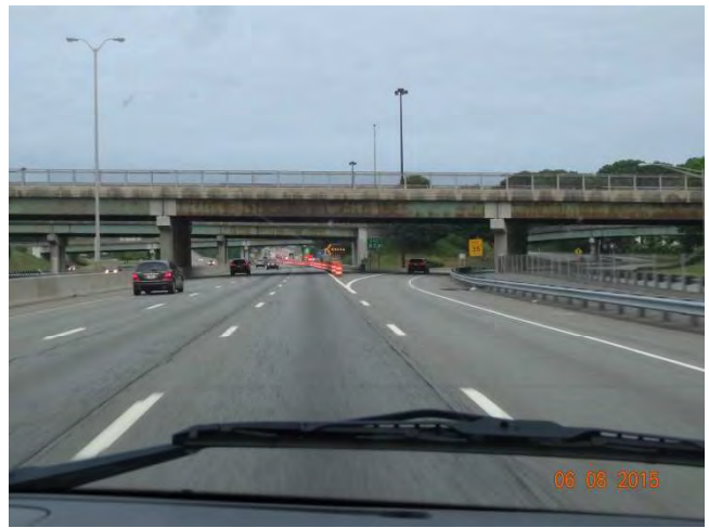
I-95 NB: Traffic pattern taper beginning at Exit 83 with a portable flashing arrow inside the pattern
