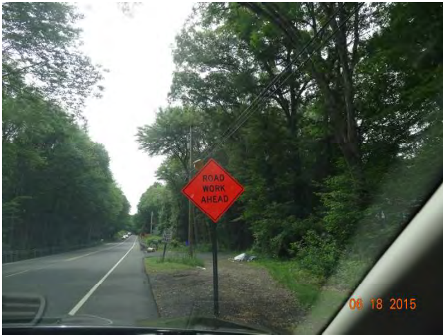
Route 79 SB: A post-mounted "Road Work Zone Ahead" sign with a high-intensity warning light attached
