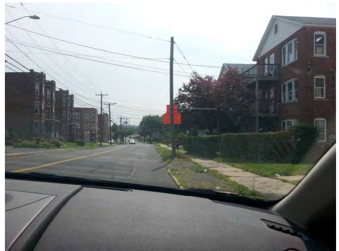
West Main Street WB: The Legal Series signs were placed just behind the utility pole. Despite placing the sign at the proposed location according to the plans, a good judgement would to place them in front of the pole to be more visible to the motorists.
