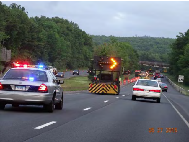
EB: The state police officer, TMAs with flashing arrows, and portable flashing arrow all working to move traffic into the appropriate lane while the pattern is being set up
