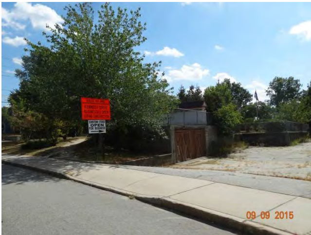
Providence Street (Route 171) SB: A construction sign informing motorists that ROUTE 44 AND KENNEDY DRIVE BUSINESSES ARE OPEN DURING CONSTRUCTION. The sign beneath it put up by the Town says DOWNTOWN STORES OPEN FOR BUSINESS.
