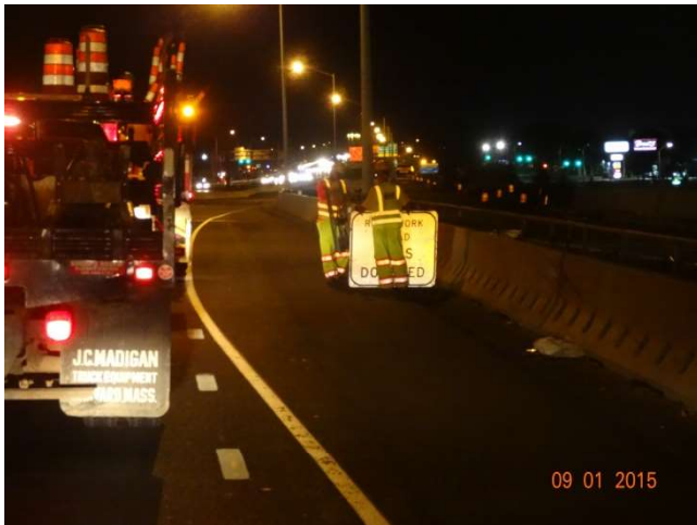
I-95 SB: The sign pattern crew setting up a FINES DOUBLED sign on the right side of the highway.
