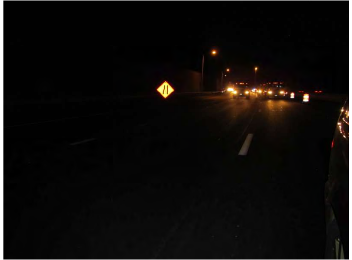
I-95 NB: The Contractor's work truck behind the work crew setting up the traffic pattern. To the side is the merge right sign that will be used later in the night when the second lane is taken.
