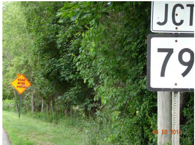
Route 148 WB: The regulatory sign stating the upcoming junction for Route 79 along with a post-mounted “Road Work Ahead” sign with warning light behind it. The construction sign is one of the extra signs the project staff added on this route.
