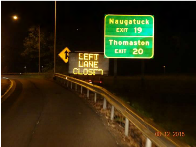
I-84 EB: The CMS near Exit 18 stating LEFT LANE CLOSED on its second frame.
