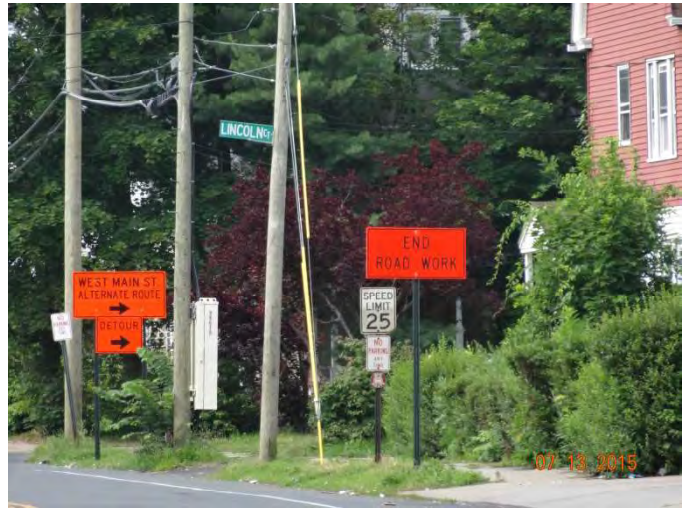
Lincoln Street: The alternate route site with DETOUR sign and an END ROAD WORK sign.
