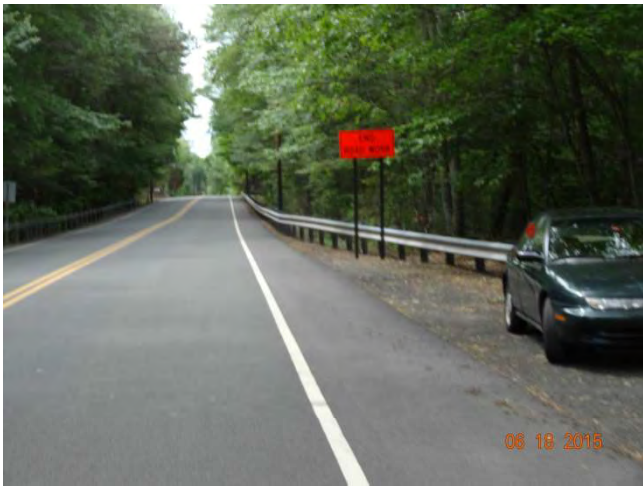
Route 79 SB: A post-mounted "End Road Work" sign
