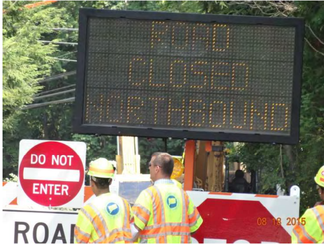
Old Mill Road NB: The first frame of the CMS stating ROAD CLOSED NORTHBOUND.
