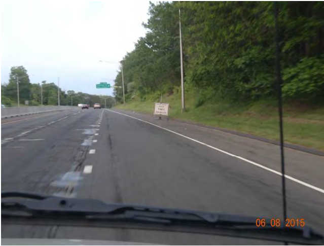
I-95 NB: Fines Doubled sign while approaching work zone
