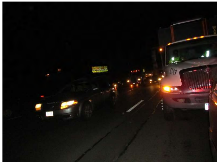
I-95 NB: The traffic bypassing the work zone after release of the rolling road block.
