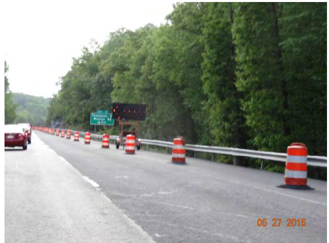
WB: A portable flashing arrow within the taper is signaling for motorists to move over
