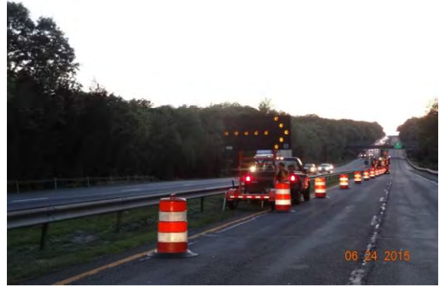
I-95 SB: A portable advanced flashing arrow within the taper
