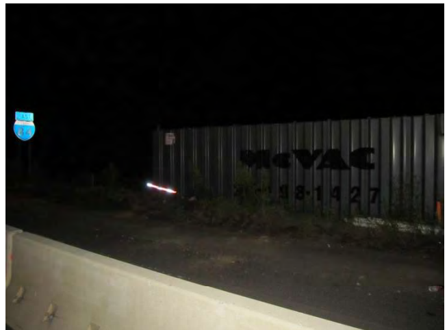
I-84 EB: The Contractor's storage container stored behind barrier on the right side of the current eastbound lanes.
