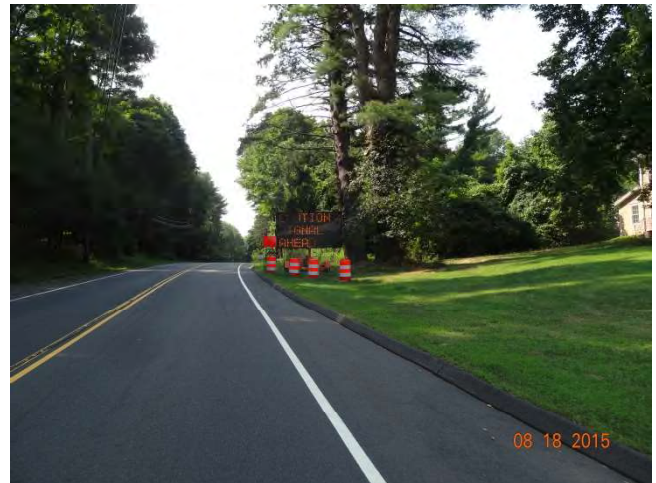
Route 53 SB: A Changeable Message sign with one frame notifying motorists CAUTION SIGNAL AHEAD. The CMS is behind traffic drums but should be positively protected.
