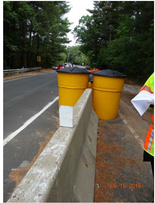
Route 79 NB: The white side of the delineator facing the northbound traffic is correct to be on their right side.
