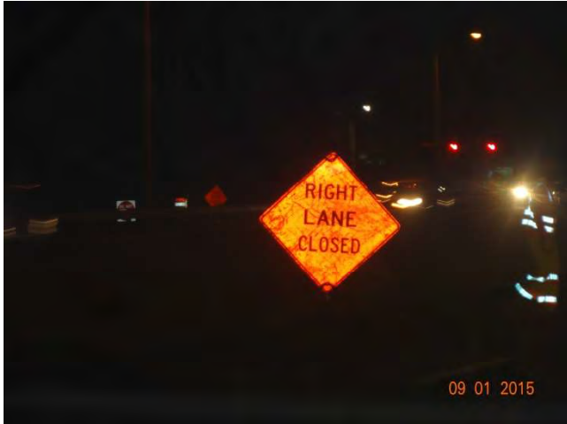
I-95 SB: The reflectivity of the RIGHT LANE CLOSED is seen here. The sign is reflective but the dirt on it does affect its effectiveness.
