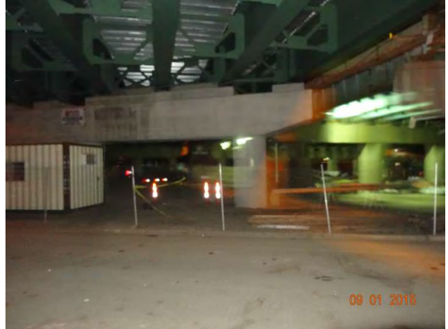
Kimberly Avenue: The other laydown yard under the I-95 overpass on Kimberly Avenue.
