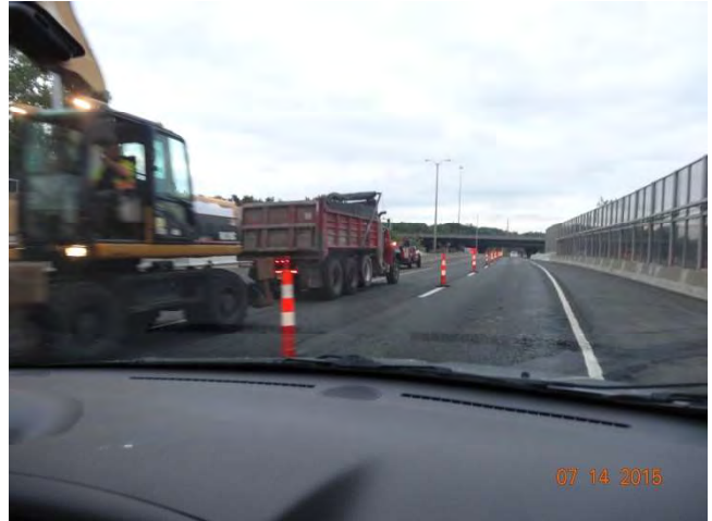
Route 15 NB: The equipment within the work area.
