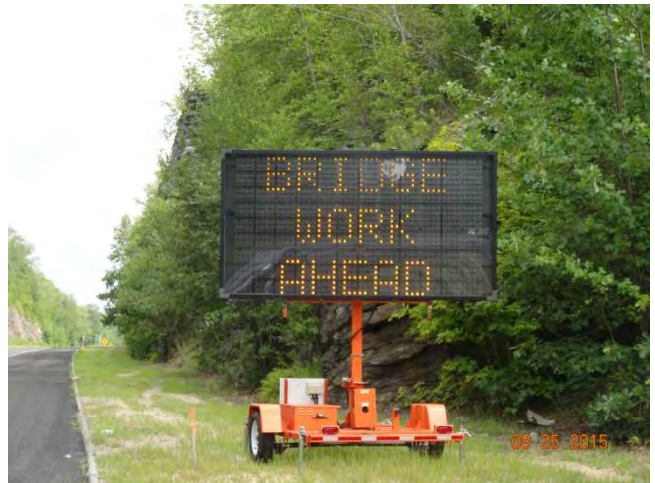
Route 11 NB: The CMS stating BRIDGE WORK AHEAD on this third frame.
