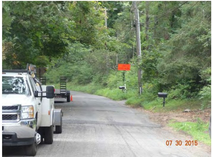
Blue Hills Road: An END OF WORK sign.
