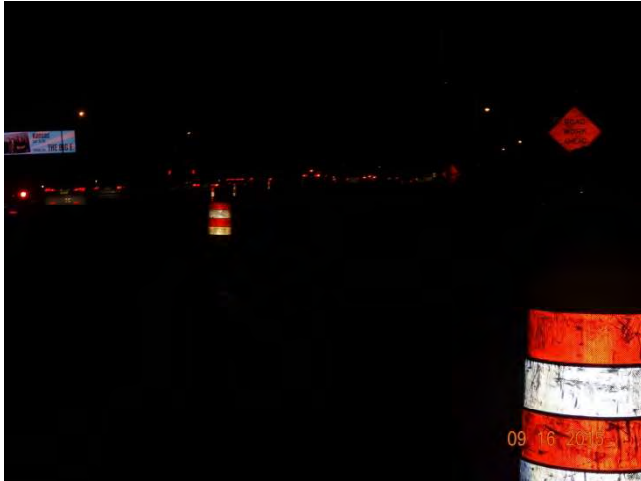
I-91 SB: The condition of the traffic drums shows that they either need to be cleaned or if scuffed, replaced.
