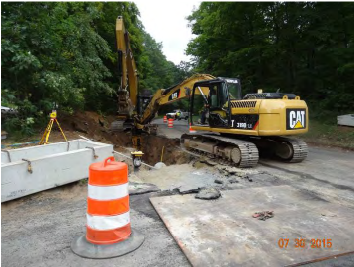
Route 148 WB: A work crew working on the drainage.
