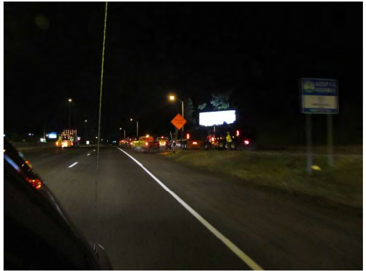
I-95 NB: A post-mounted sign saying SHOULDER CLOSED and dump trucks loaded with asphalt lined up for the paving operation.
