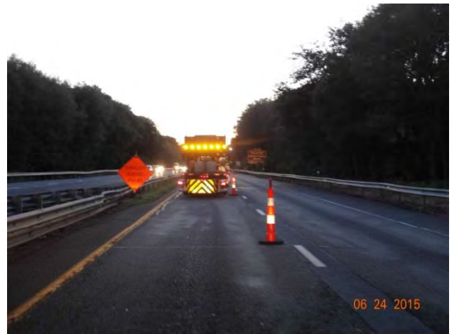
I-95 SB: A crash truck with a flashing arrow within the traffic pattern
