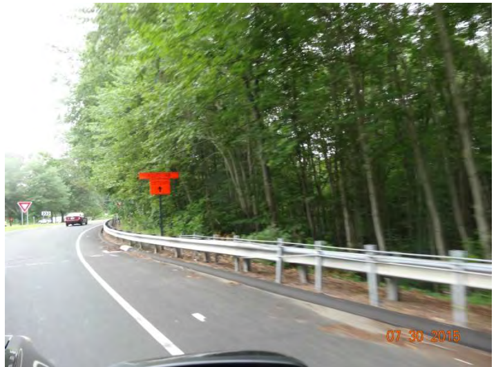
Route 79 SB: A detour sign for Route 148 right before entering the roundabout.
