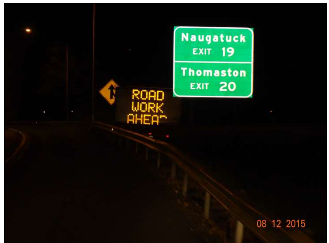
I-84 EB: A CMS near the Exit 18 (Chase Parkway) on ramp stating the ROAD WORK AHEAD on its first frame. The CMS is rather low behind the guiderail and could be difficult for motorists to see.
