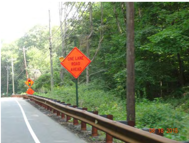
Route 53 NB: A post-mounted ROAD WORK AHEAD sign with a high-intensity barricade warning light.
