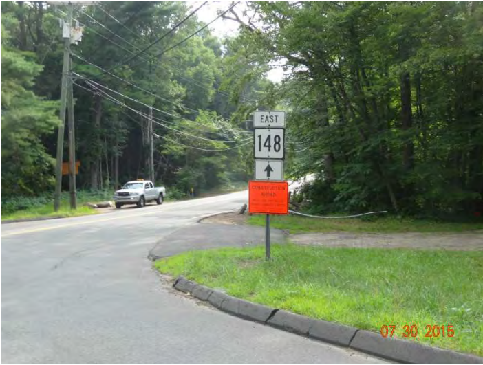
Route 148 EB: A legal series sign for an adjacent project within the detour.
