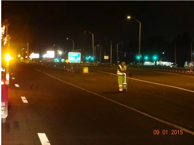
I-95 SB: A worker setting up another temporary construction sign support.
