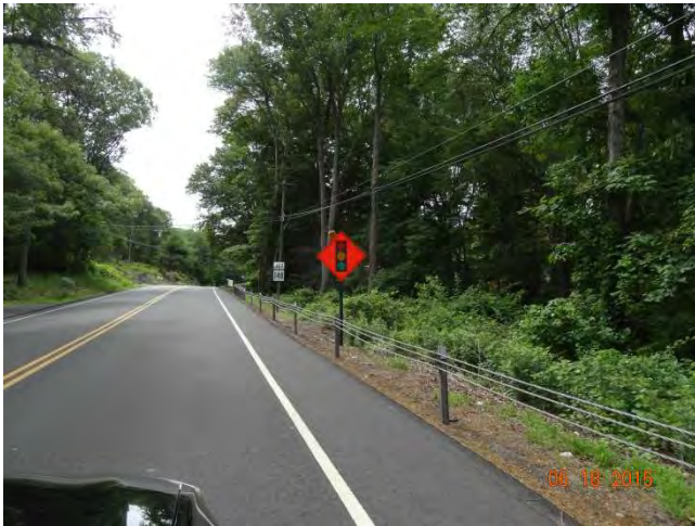
Route 79 SB: A post-mounted Signal Ahead sign with a high-intensity warning light
