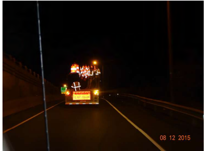
I-84 EB: The sign crew heading out onto I-84 to set up the traffic pattern.
