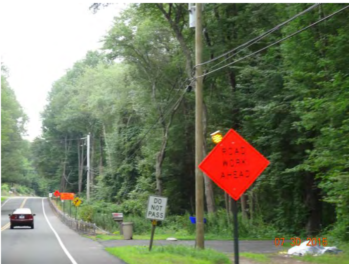
Route 79 SB: A ROAD WORK AHEAD sign with a high-intensity warning light.
