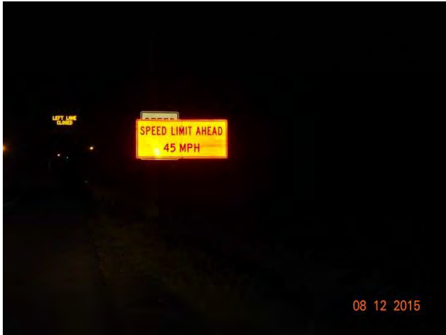
I-84 EB: A SPEED LIMIT AHEAD 45 MPH construction sign informing the motorists that the speed limit for this section of I-84 has been legally reduced to 45 mph.
