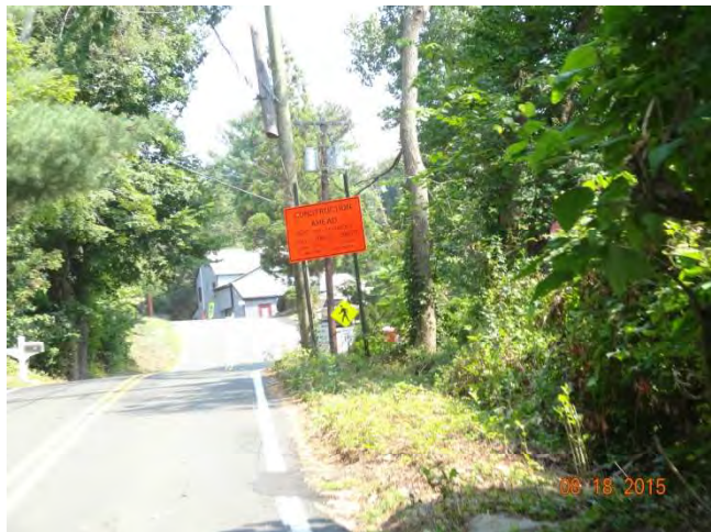
Old Mill Road NB: A post-mounted legal series sign on 7-foot posts.
