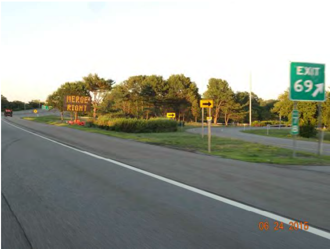
I-95 NB: The Changeable Message Sign in the Exit 69 gore area.
