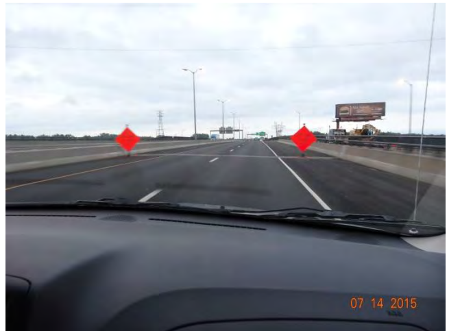
Route 15 NB: Signs on both sides of highway stating LEFT LANE CLOSED.
