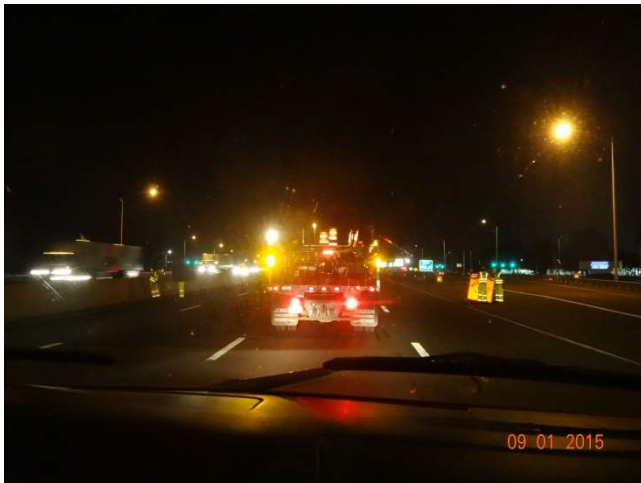
I-95 SB: Two workers installing a temporary RIGHT LANE CLOSED.
