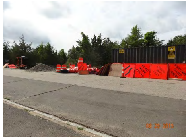
Route 11 NB: The stockpiled materials in the laydown yard.
