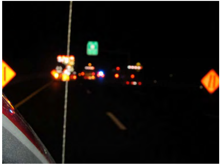
I-95 NB: The advance warning signs on the both sides of the highway.
