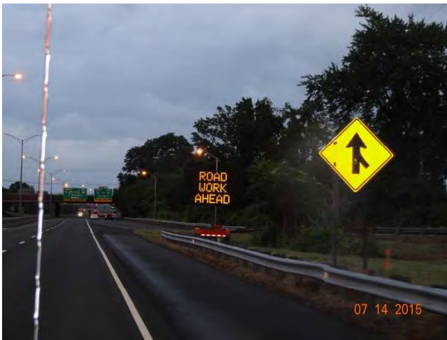
Route 15 NB: A Changeable Message Sign at the Exit 88 on ramp.
