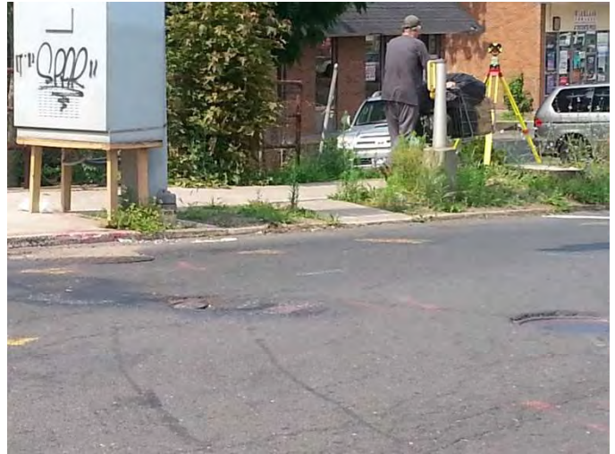
West Main Street EB: Existing sidewalk ramp on the south side of road.
