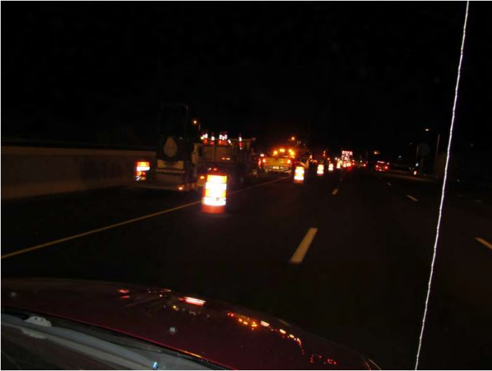
I-95 NB: The taper extending into a full lane closure of the left lane with the work crew on the inside of the pattern.
