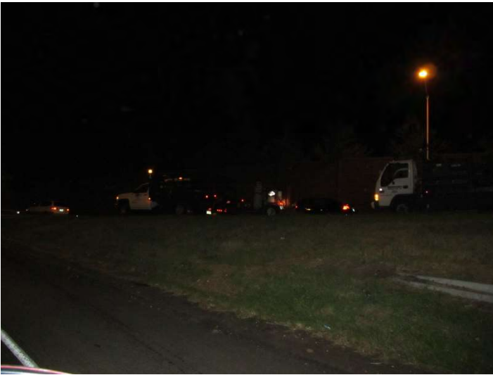
I-95 NB: More of the Contractor's crew coming onto the highway.
