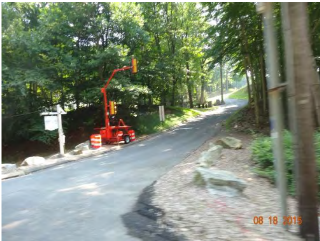
Route 53 NB: The temporary signal at the entrance to the Weston Racquet Club.
