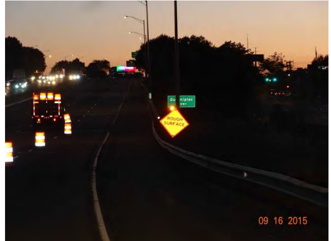
I-91 SB: The ROUGH SURFACE sign shown previously but now with its high-intensity barricade warning light flashing since the sun set.
