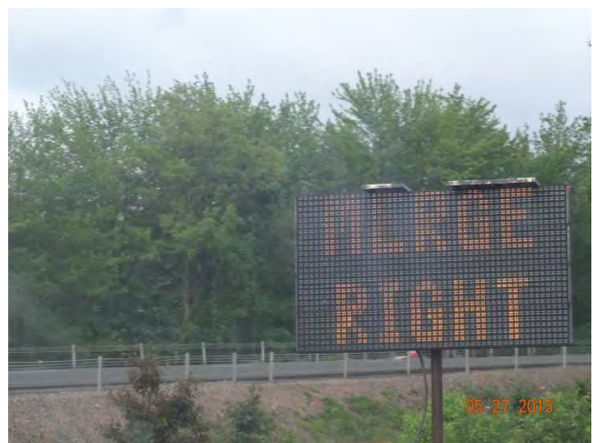
Eastbound (EB): The Changeable Message Sign (CMS) in the median
