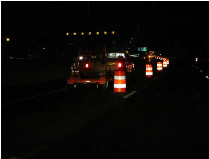
I-95 NB: An advance flashing arrow in the closed lane signaling with a straight bar that the lane is closed.
