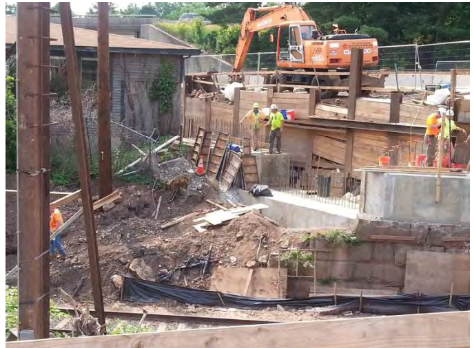
West Main Street: The Contractor working on the north side abutment.
