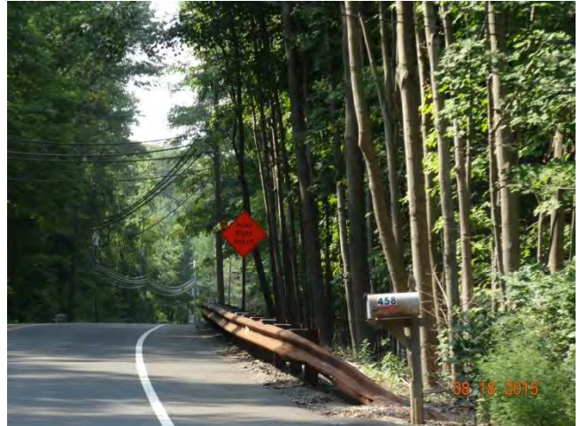
Route 53 SB: A post-mounted ROAD WORK AHEAD sign with a high-intensity warning light.
