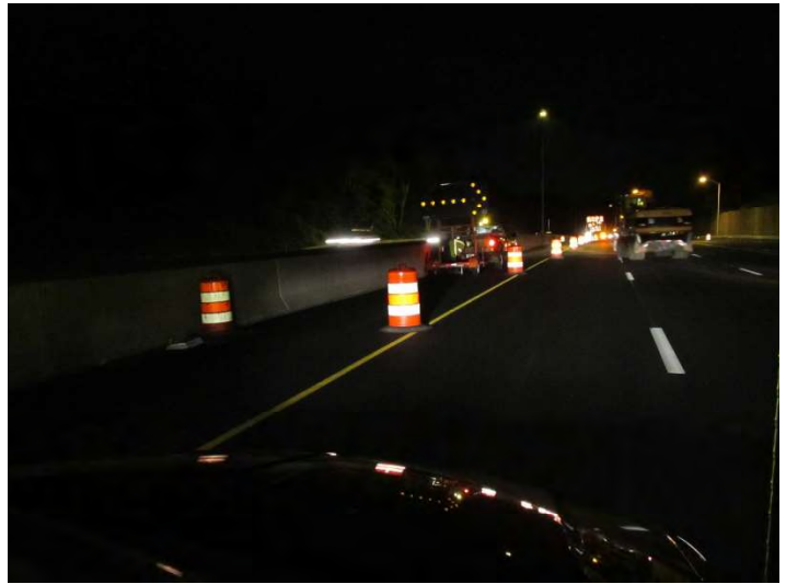
I-95 NB: The advance flashing arrow within the taper signaling to motorists to merge right.
