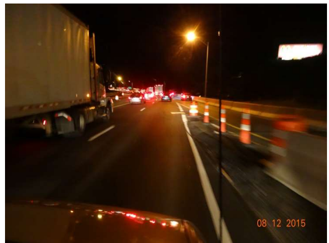
I-84 EB: The traffic passing through the work zone.
