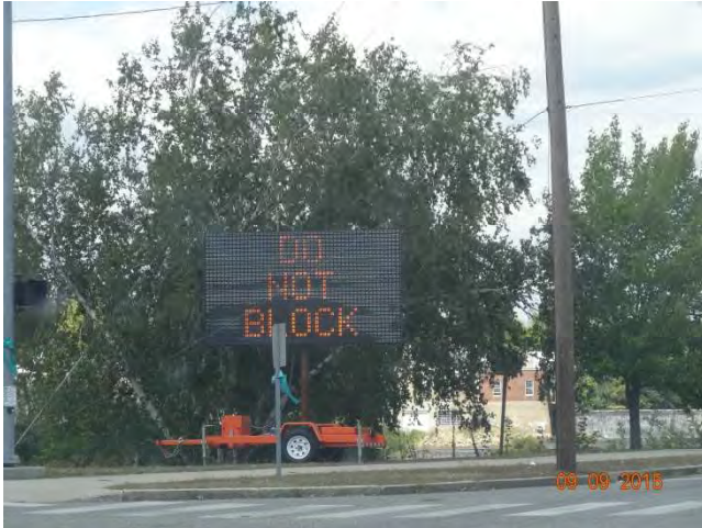
Kennedy Drive NB: The only Changeable Message Sign (CMS) for the project which is located behind the sidewalk. The first frame says DOT NOT BLOCK.
