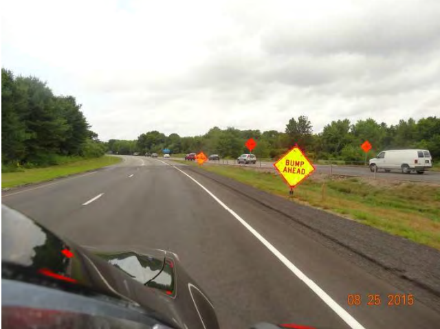
Route 11 NB: Route 11 merging with Route 2. Temporary signs warning motorists of BUMP AHEAD and BUMP, respectively. The reflectivity of the BUMP AHEAD sign is visibly displayed.
