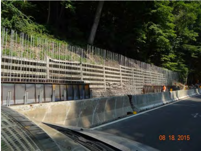
Route 53 NB: The work crew is replacing the retaining wall.
