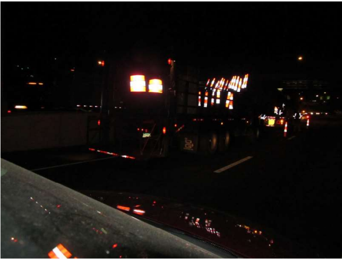
I-95 NB: Traffic cones used for the traffic pattern around the closed left lane.
