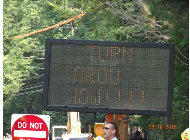
Old Mill Road NB: The third frame stating TURN AROUND NOW!!!!
