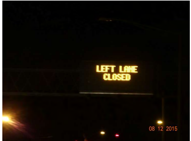
I-84 EB: The VMS stating LEFT LANE CLOSED on its second frame.
