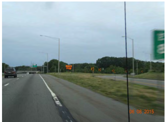
I-95 NB: Changeable Message Sign (CMS) at Exit 81 with a message to reduce speed.
