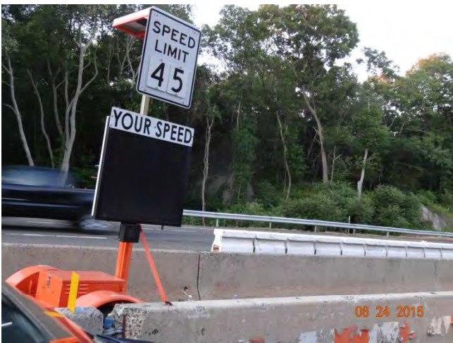
I-95 NB: The radar speed trailer in the median behind TPCB barrier
