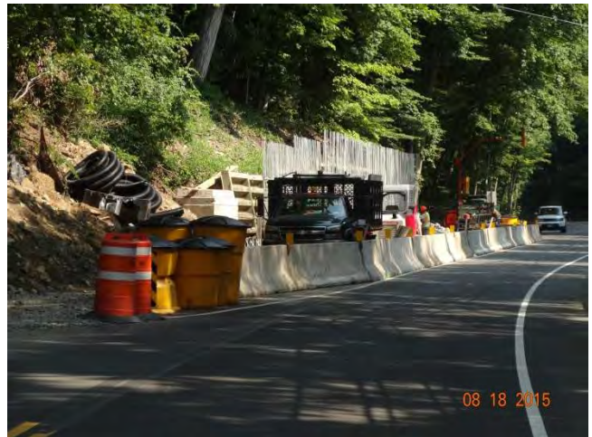
Route 53 NB: The work zone behind concrete barrier curb.
