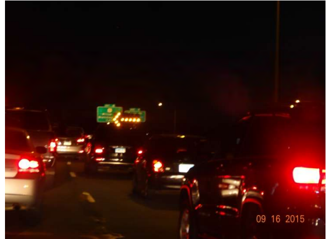
I-91 SB: A portable flashing arrow signaling for motorists to merge left.
