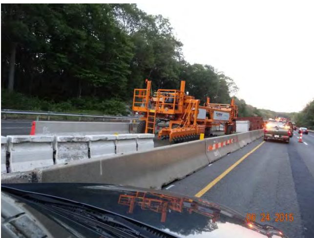
I-95 NB: The moveable barrier and with moving device
