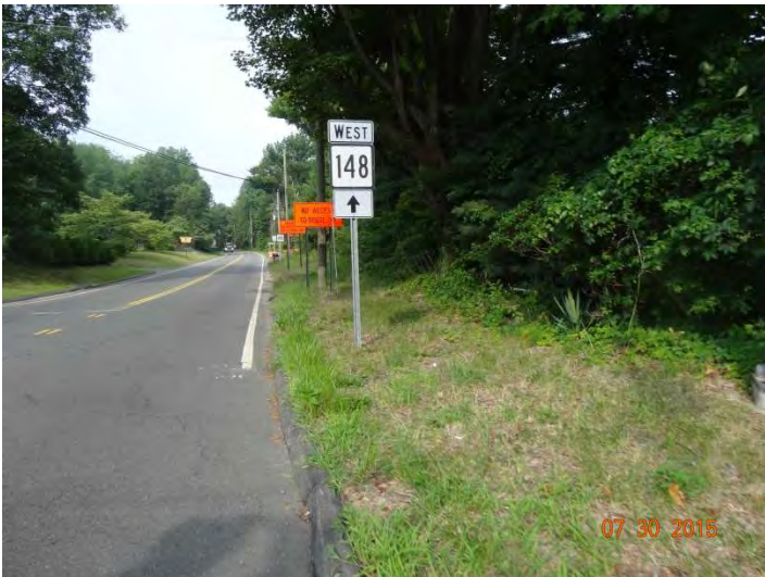
Route 148 WB: Behind the route sign, construction signs stating NO ACCESS TO ROUTE 79 and BRIDGE CLOSED 5.0 MILES AHEAD RTE 148 TRAFFIC ONLY.
