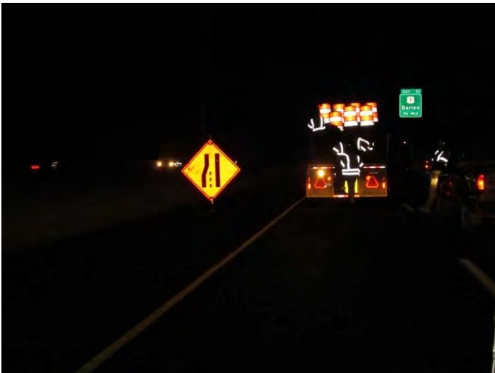
I-95 NB: A merge right depiction sign on the left side of the highway.
