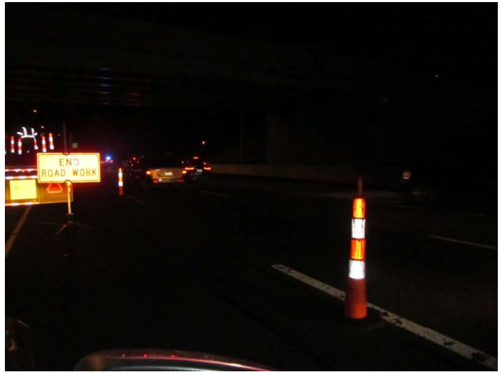
I-95 NB: The END ROAD WORK AREA sign directly after the lane closure with traffic starting to bypass the work zone. This sign was not visible to motorists and was not installed on both sides of the road.
