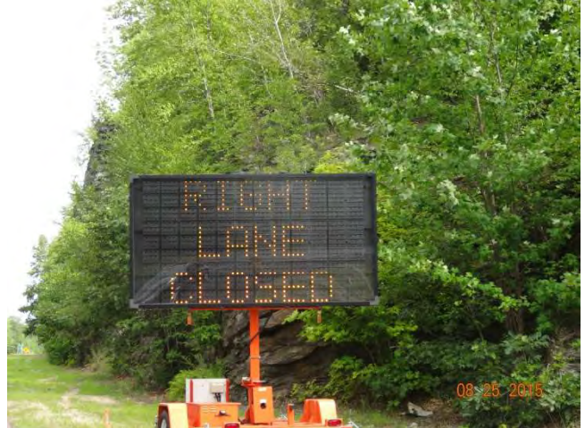
Route 11 NB: The CMS stating RIGHT LANE CLOSED on its second frame.
