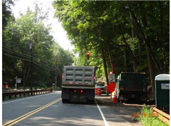
Route 53 SB: A red light on the temporary signal and a truck waiting at the stop bar signaled by the sign. There is another sign at the stop bar reminding cyclists to obey the traffic signal.
