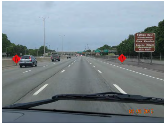
I-95 NB: Merge left signs on both sides of the road
