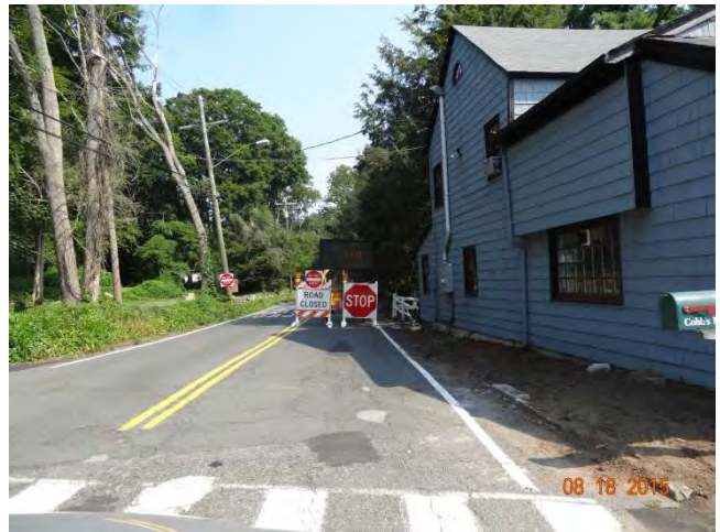
Old Mill Road NB: Type III barricades closing the northbound lane with a ROAD CLOSED and STOP sign in front. Also a Changeable Message Sign notifying motorists of the closure.
