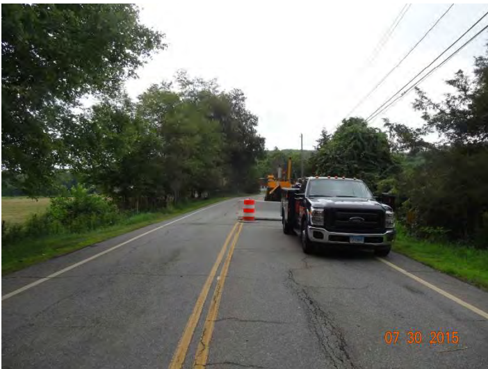
Route 148 EB: Concrete barrier closing the travel way on the road.
