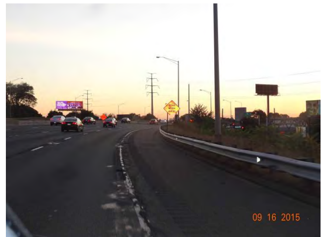
I-91 SB: A post-mounted ROAD WORK AHEAD sign with a barricade warning light attached. The bottom point of the sign has been broken off; the condition of the sign is poor and should be replaced.
