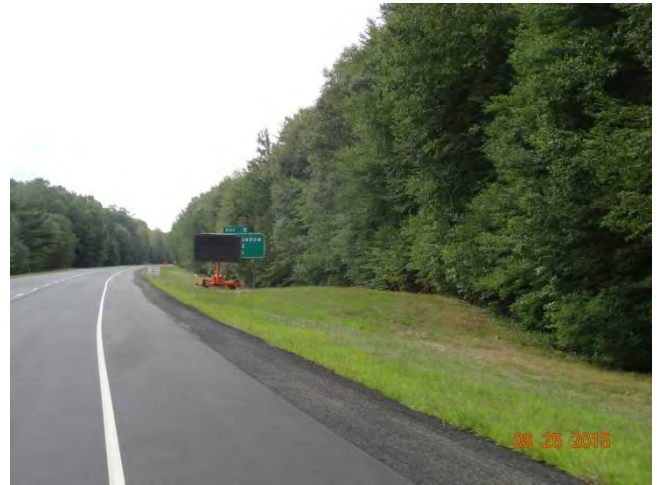
Route 11 SB: A Changeable Message Sign (CMS) that is currently not being used. It also is not behind any positive protection.
