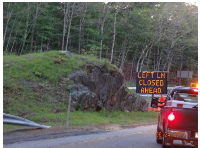
I-95 SB: The Changeable Message Sign in the Exit 72 gore area. This was the best location for the message sign although it is partially obstructed by the rock. The project is looking to move it to a better location now that the adjacent project is completed and their advance warning is removed.
