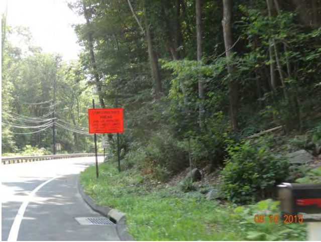
Route 57 SB: A post-mounted legal series sign on 7-foot posts.
