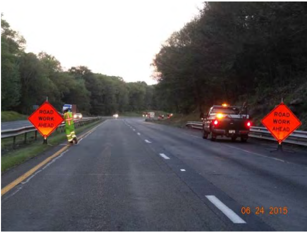
I-95 SB: The advanced warning deployed on both sides of the highway
