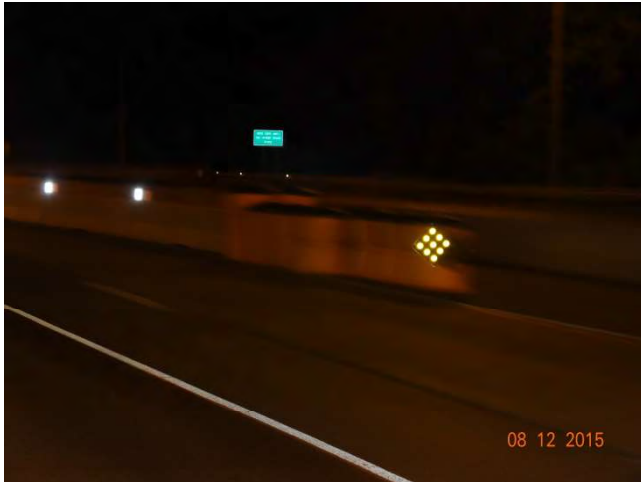
I-84 EB: A Type A Impact Attenuation System with delineator in front of the blunt end of concrete barrier.
