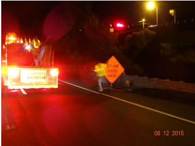
I-84 EB: LEFT LANE CLOSED AHEAD sign being set up.
