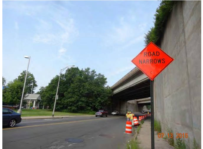
West Main Street EB: A post-mounted ROAD NARROWS sign west of the bridge.
