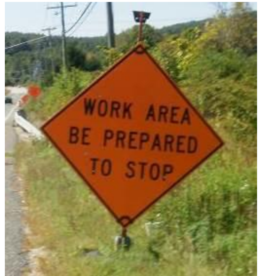
Additional signage provided by the contractor.
