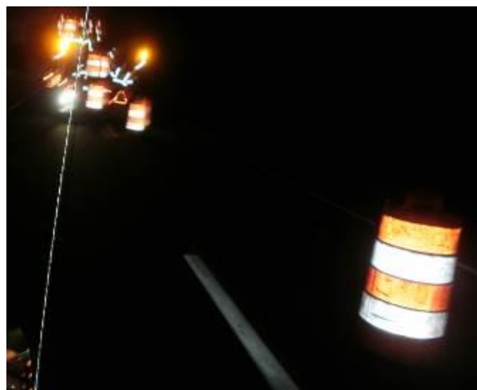
Traffic drums are placed for lane closure.
