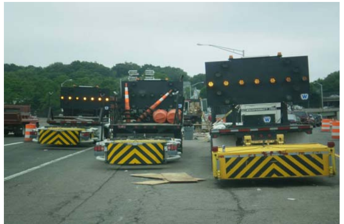
Figure 3: Work Area Protection
