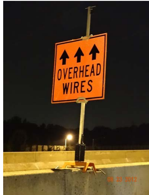
Median barrier clamping system for signs and safety sign used by contractor for trucks delivering materials. Good Practice
