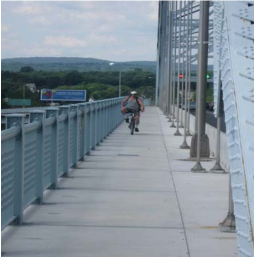
Bicyclist utilizing sidewalk during construction
