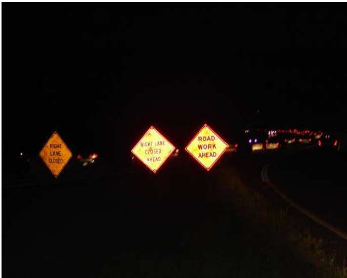
Ramp signs not installed; Again notice Type III versus Bright Fluorescent Sheeting.
