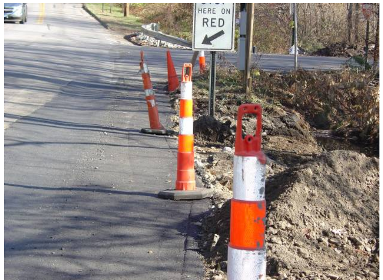
Missing or faded Stop Bar
