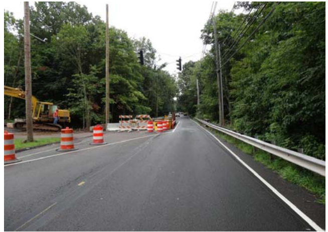
DE-9 delineator is temporarily blocked by the barrel. Type III barricade on the right has striped pattern sloping in the opposite direction.
