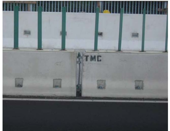
Anchored Barrier Curb with Glare screen
