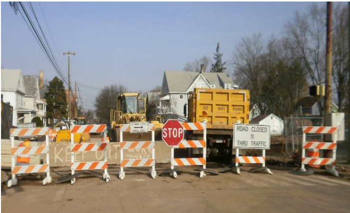
Type III barricades and signs placed at south end of bridge. Barricade stripes should all be sloping downward in the direction traffic is to pass (in this case to the left) and be retroreflective.
