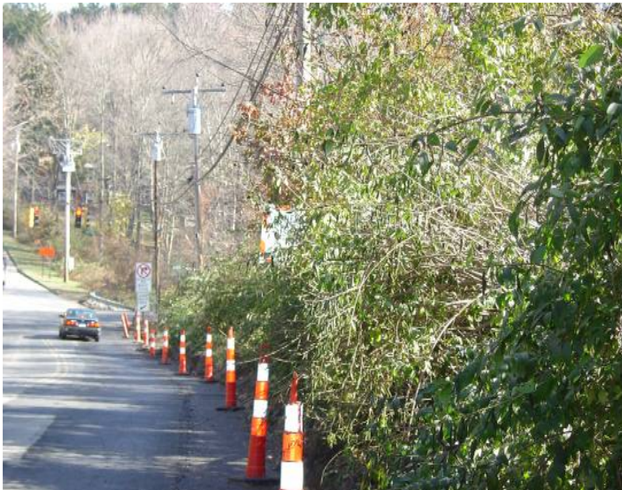
Overgrown brush blocking view of sign.
