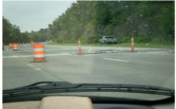
Sign in the distance and impact attenuation vehicle in the background with proper signal
