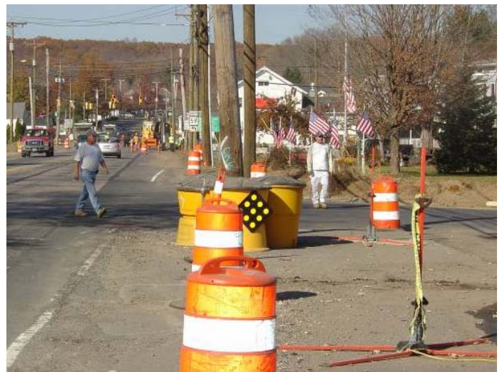
Impact Attenuation System protecting utility poles.
