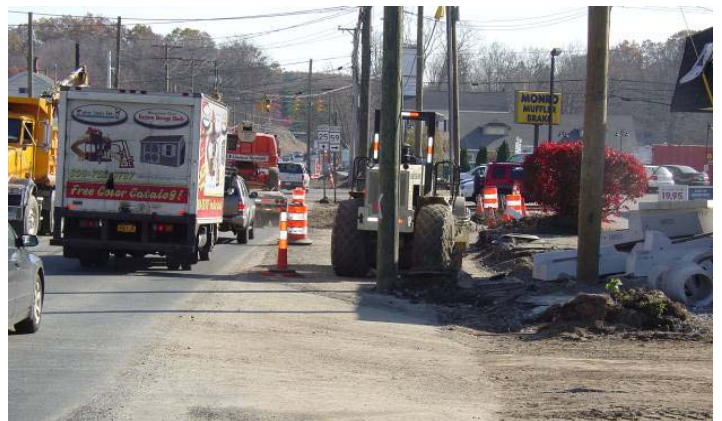
Lunchtime Traffic Queue. Utility pole requiring removal
