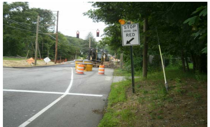
Proper placement of sign and pavement markings for temporary signalization at bridge Notified inspector about traffic barrel blocking view of Delineator
