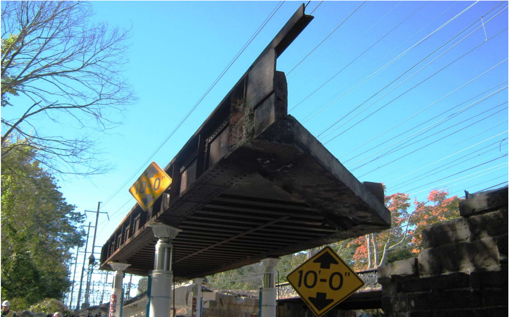
View of the removal of first two tracks.
