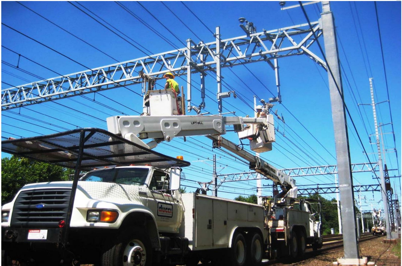
Workers install and adjust new catenary wire.
