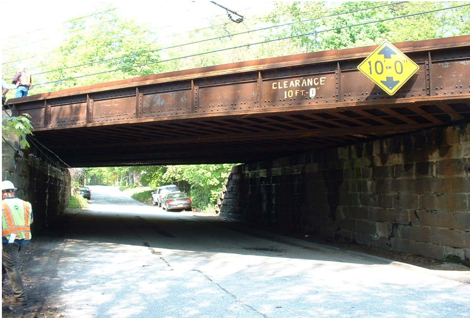
View before removal of first two tracks.
