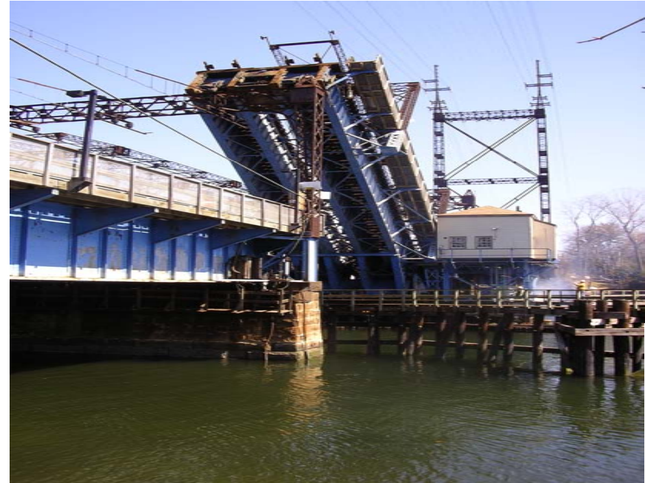
SAGAUTUCK (SAGA) MOVABLE LIFT BRIDGE
