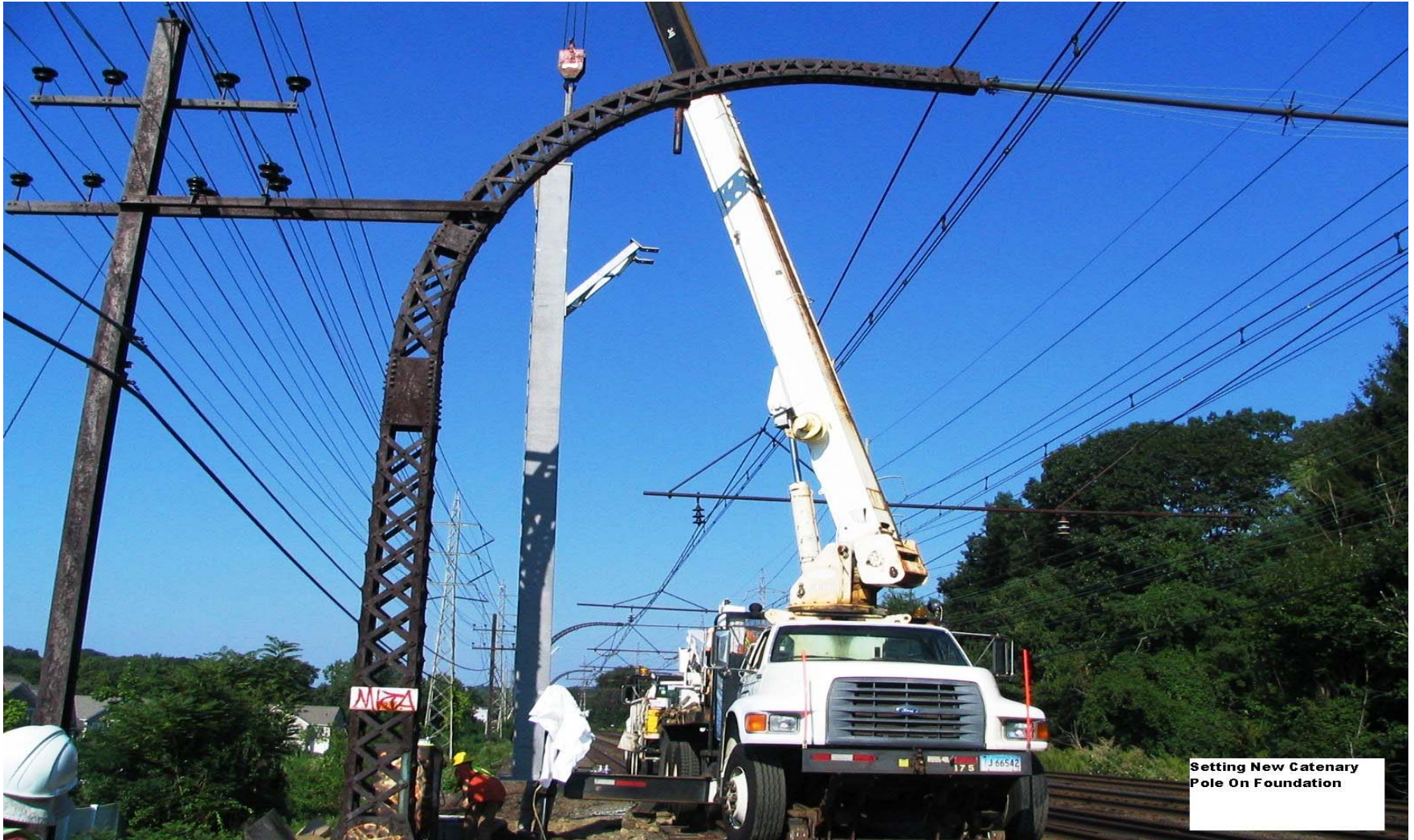
Experimental Arch Catenary
