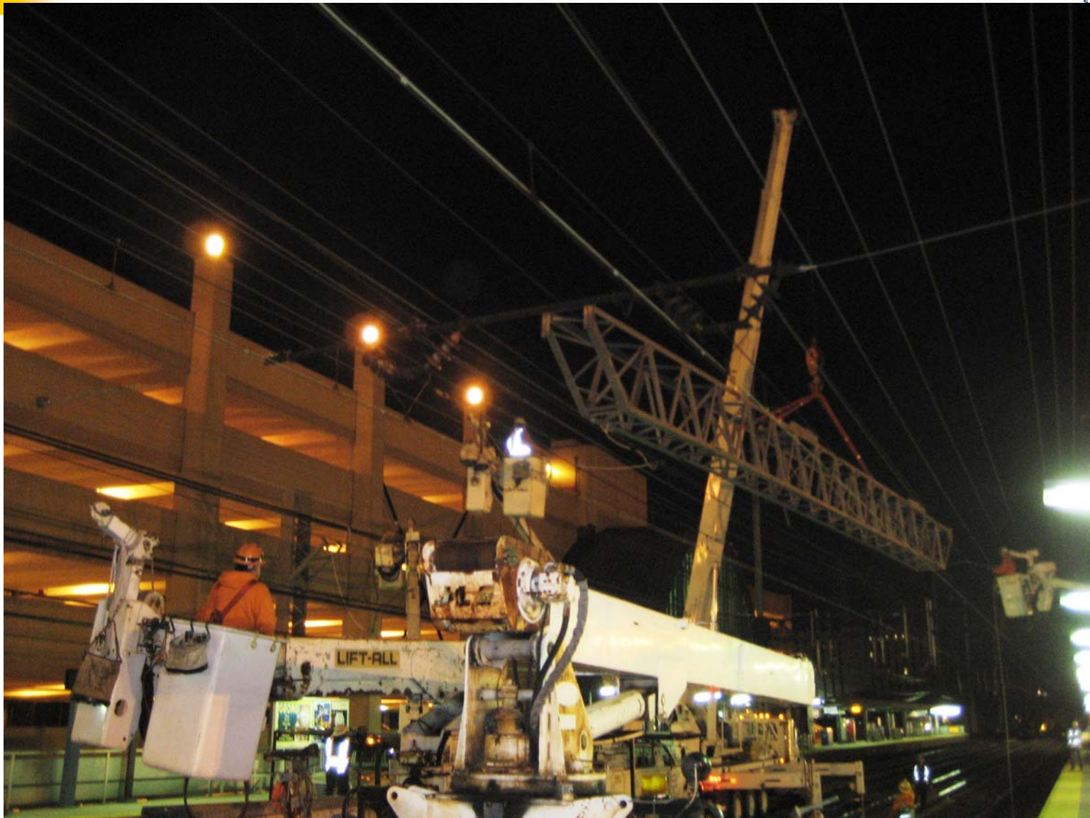
New catenary truss is lifted vertically to clear existing catenary.
