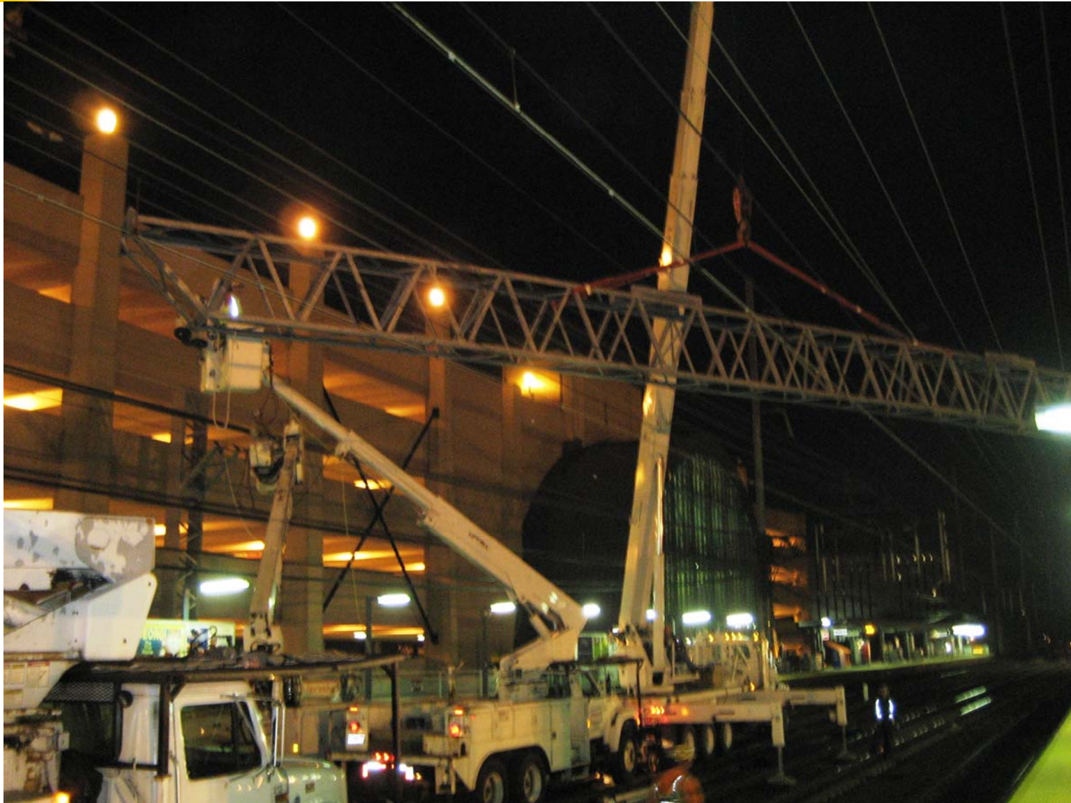
Spinning new portal truss over to its vertical columns.
