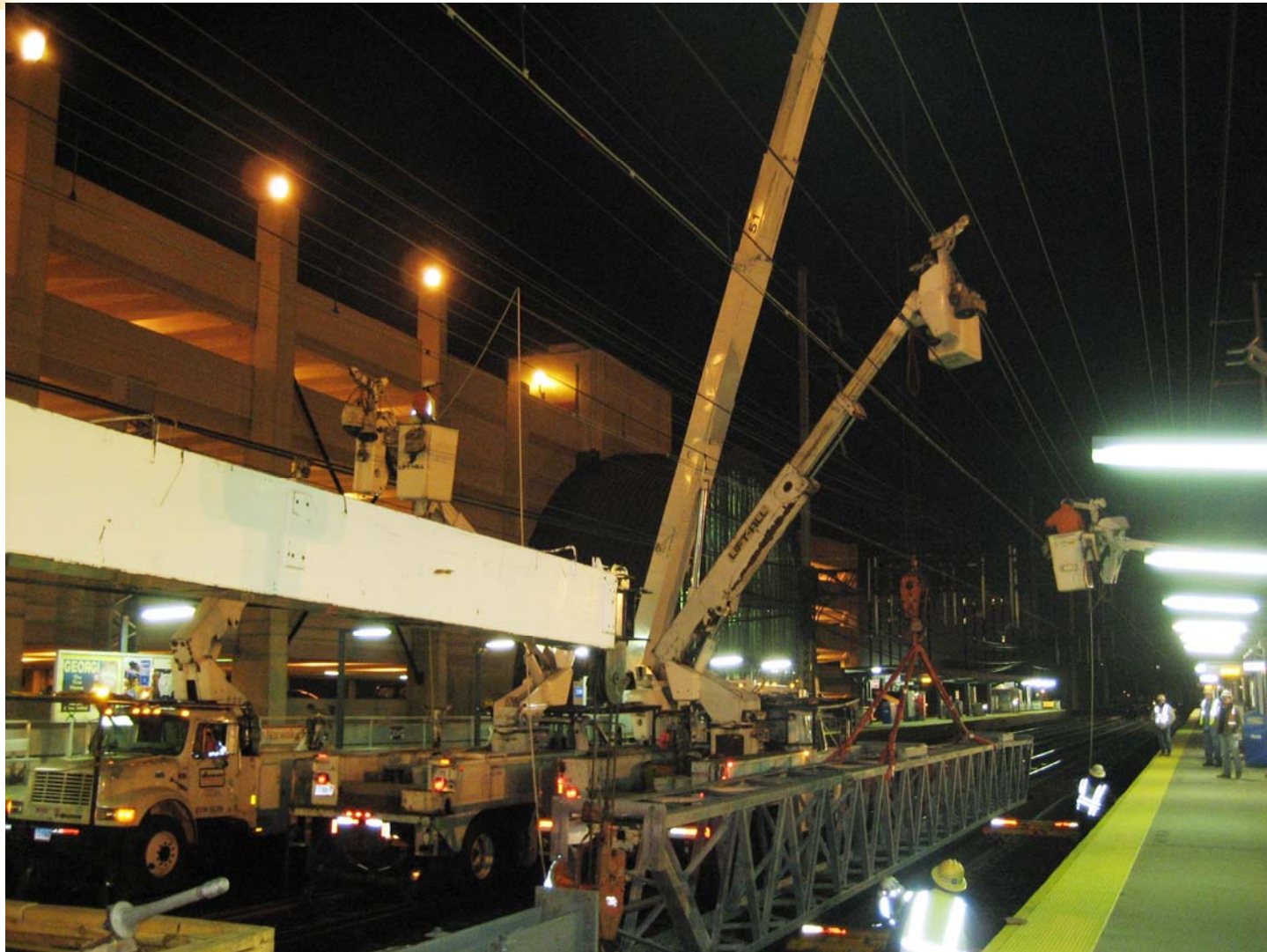
Preparing to lift new catenary truss.
