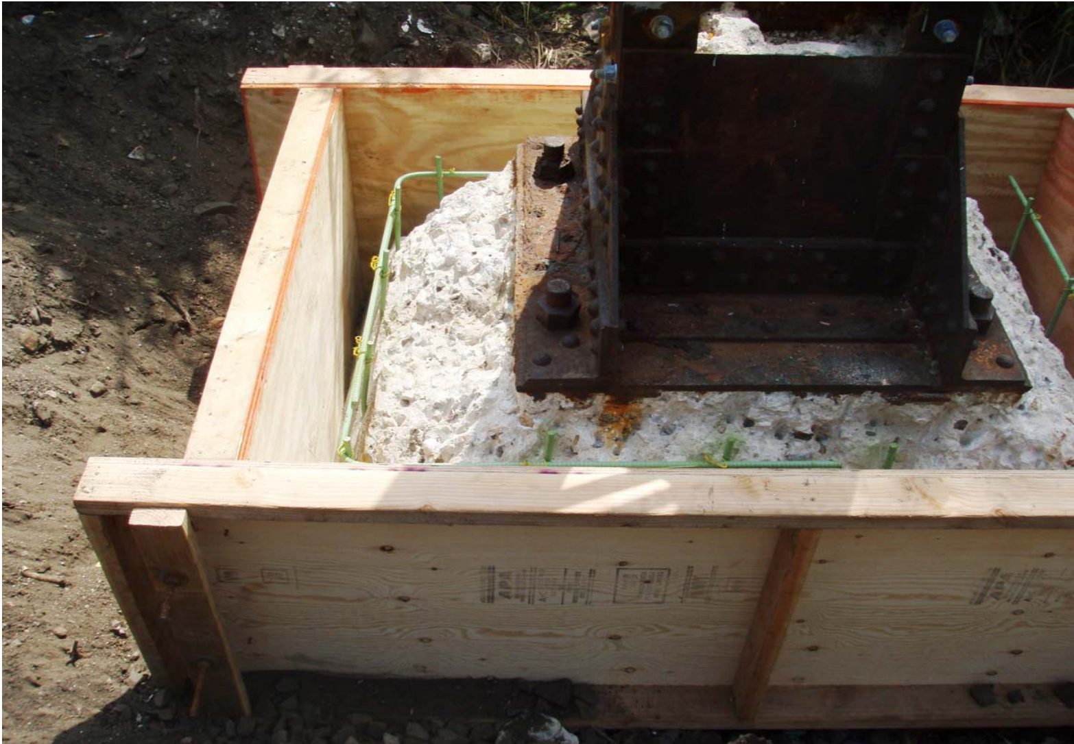
Foundation repairs – formed and ready for concrete.
