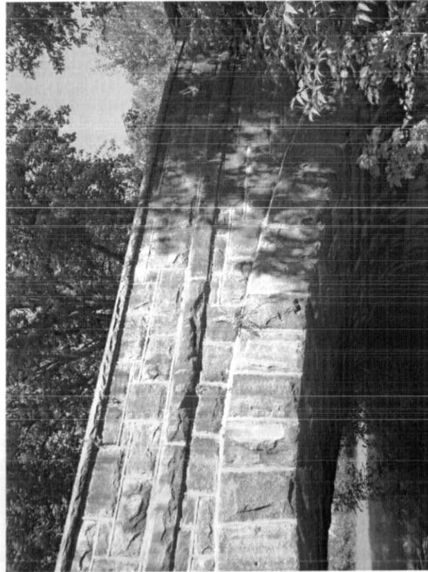
Photo # 17: Span 2, south spandrel and railing, typical.
