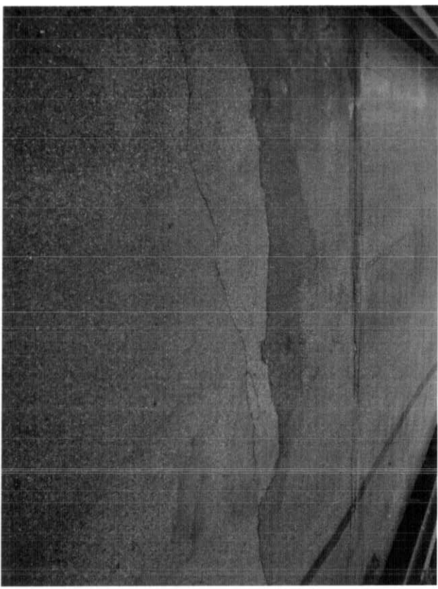
Photo # 5: WEST APPROACH PAVEMENT.
