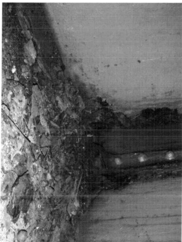
Photo # 27: BEAM END # 7 NORTH FACE AT ABUTMENT # 1
