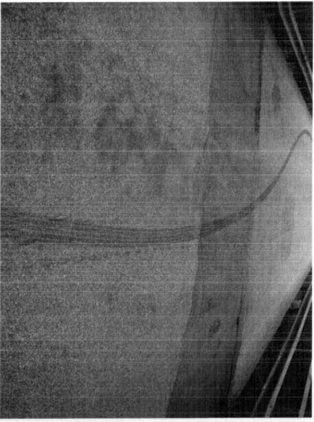
Photo # 6: EAST APPROACH PAVEMENT.
