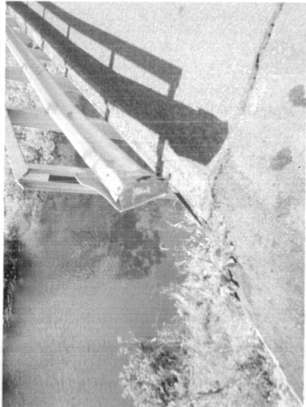
Photo # 7: Trailing edge bridge guide rail with terminal end (southwest corner shown)
