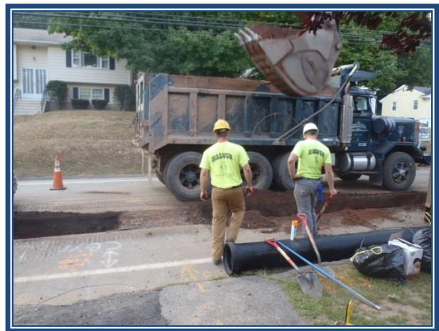
Meriden Swain Avenue Water Main Replacement
