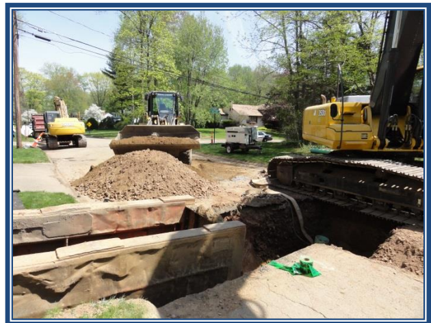
MDC –Pheasant Lane, Bloomfield Water Main Replacement
