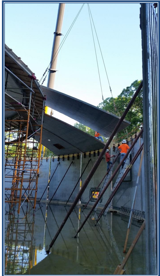
Southington Water Tower Construction
