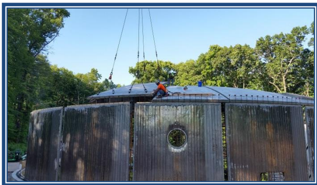
Southington East Side Tank Roof Panel Being Lowered in Place
