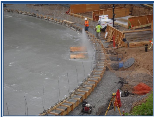
MDC North Storage Basin – Construction of Concrete Foundation of Tank
