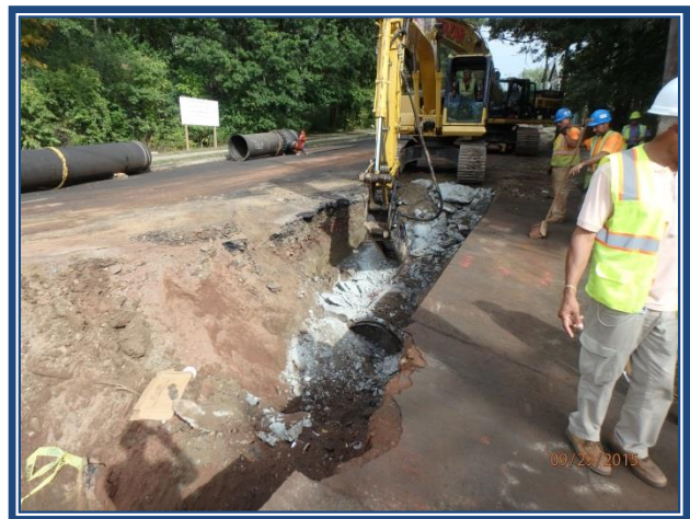
MDC Transmission Main Replacement – Removal of Old Main
