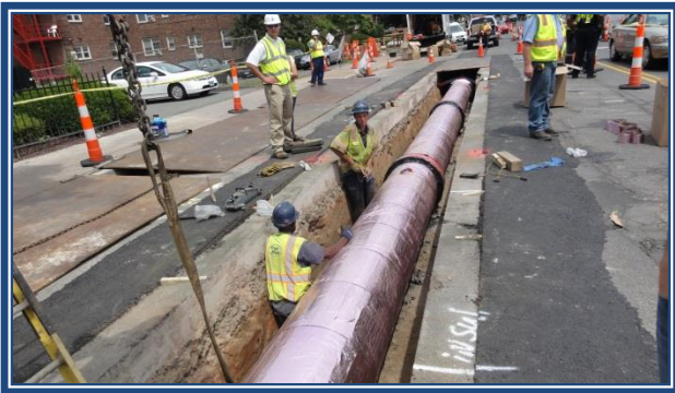
MDC Farmington #10 Installation of Insulated Water Main
