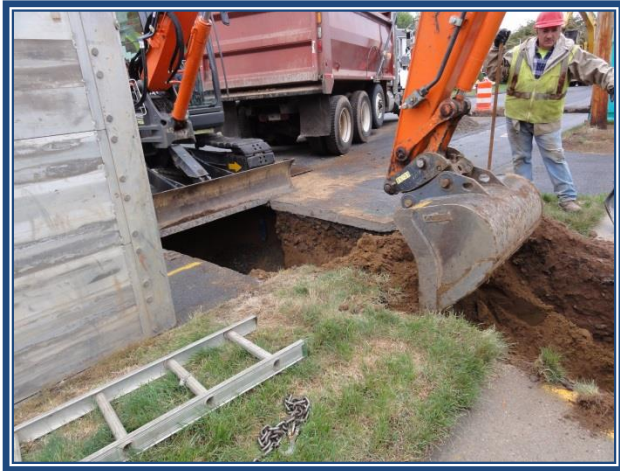
MDC –Wethersfield Water Main Replacement – Backfilling of Trench
