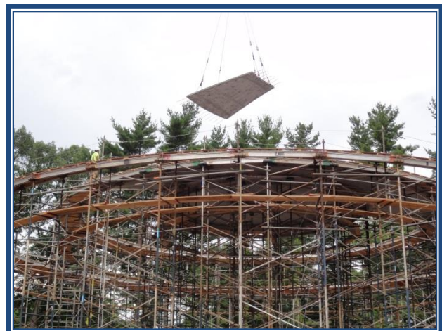
New Britain - Elam Street Storage Tank Replacement
