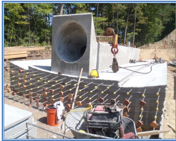
Wall panels and tank overflow being prepared for installation
