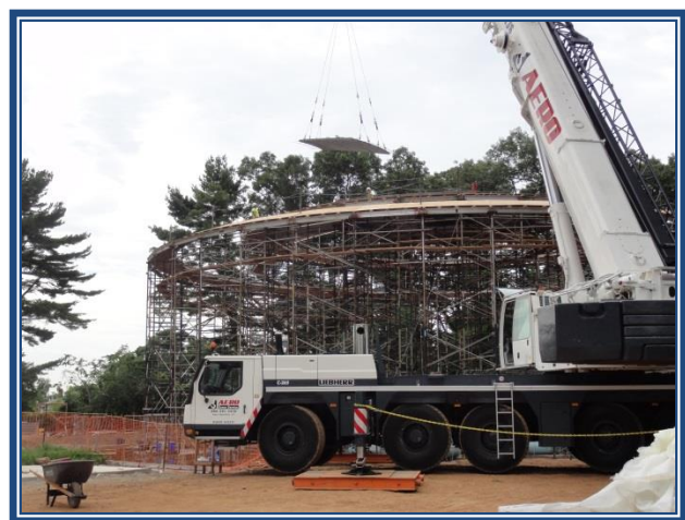
New Britain - Elam Street Storage Tank Replacement
