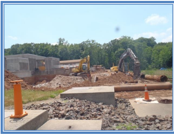
Meriden Water Treatment Plant Construction
