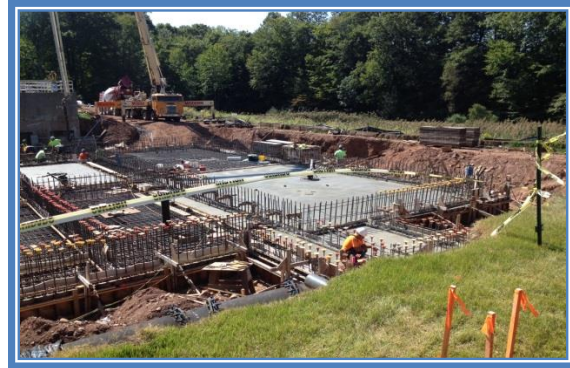
Meriden Water Treatment Plant Construction
