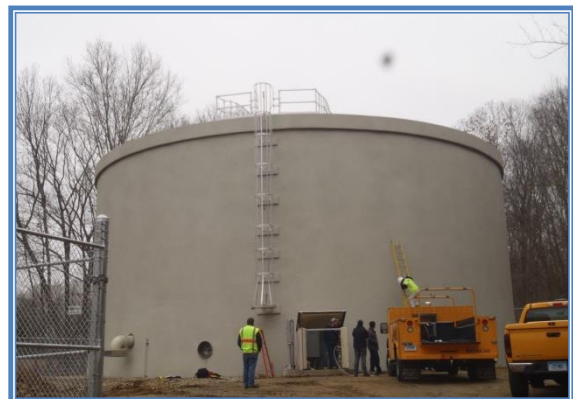
Final Inspection of the tank
