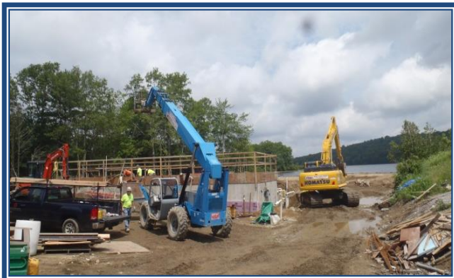
New London Pump Station Construction
