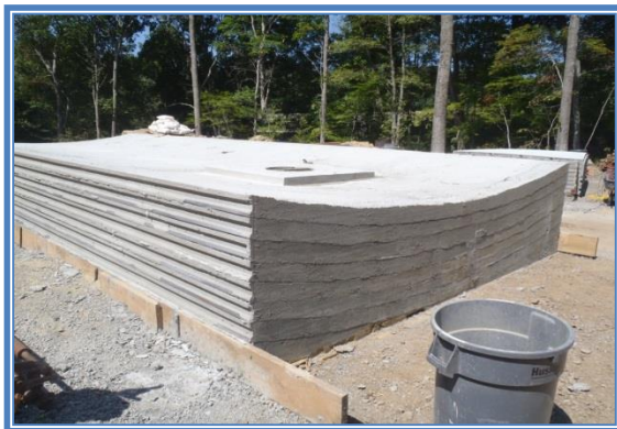
Tank wall panels were fabricated on site
