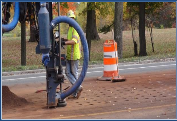
MDC-Boring holes to ease pavement removal for water main installation
