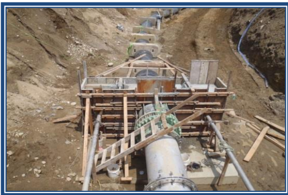
New London – New Intake Pipeline
