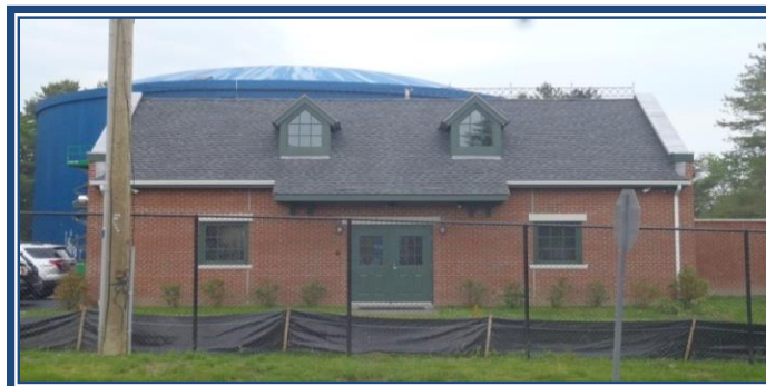
Norwalk First Taxing District- Recently Completed Booster Station, which provides water to the Spring Hill high service area, including Norwalk Hospital
