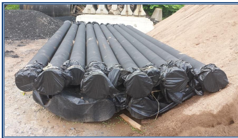
MDC - New water main line to be installed
