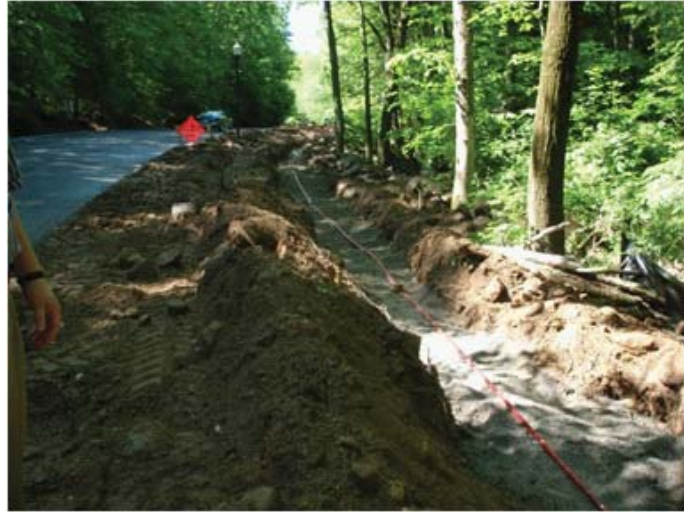
Woodlake Tax District – Water Main Installed
