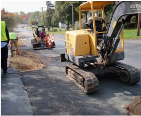
Town of Portland - Preparation of Water Main Installation
