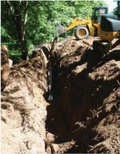
Woodlake Tax District – Installation of Water Main
