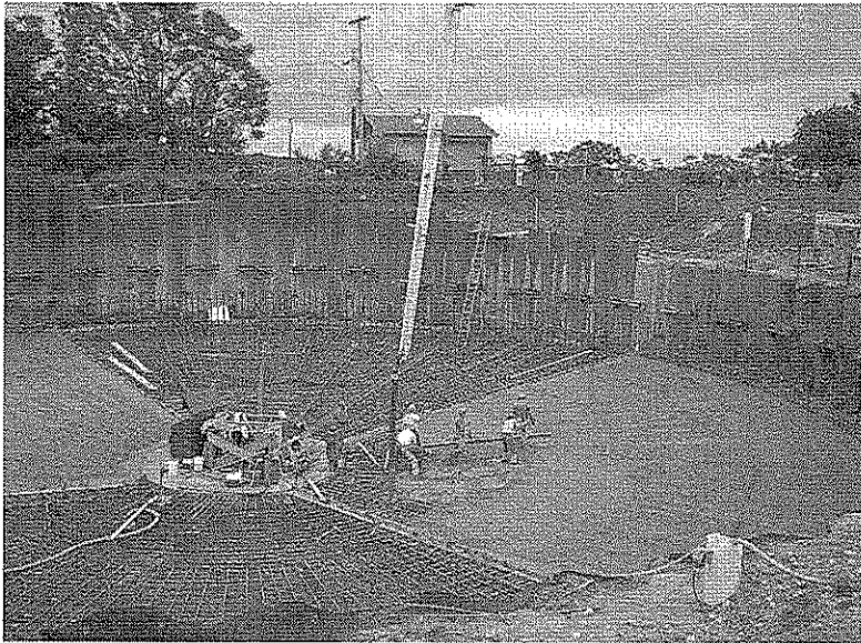
Stratford Wastewater Treatment Facility Clarifier Slab Placement
