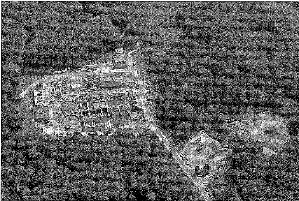
Aerial view of Groton Treatment Facility
