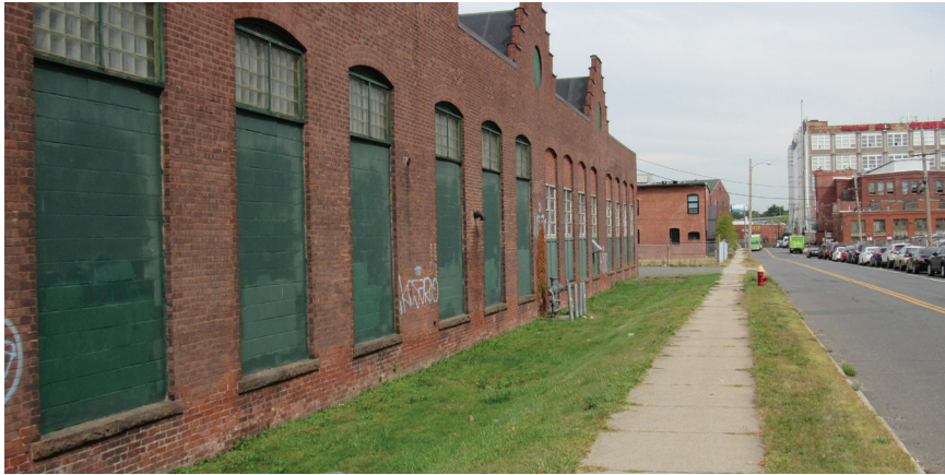
Existing Conditions on Bartholomew Avenue (Site B) Looking North
