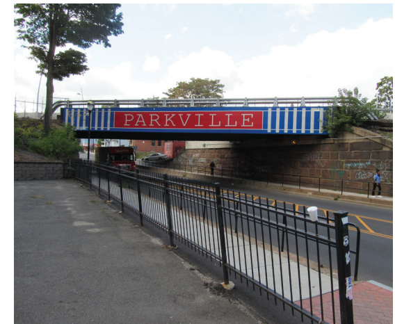
CT fastrak Guideway Bridge Looking West on Park Street
