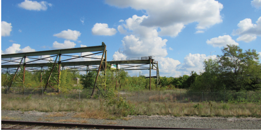
Existing Conditions on Suisman Site (Site F) Looking East
