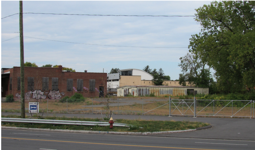
Entrance into Site F from Flatbush Avenue Looking North
