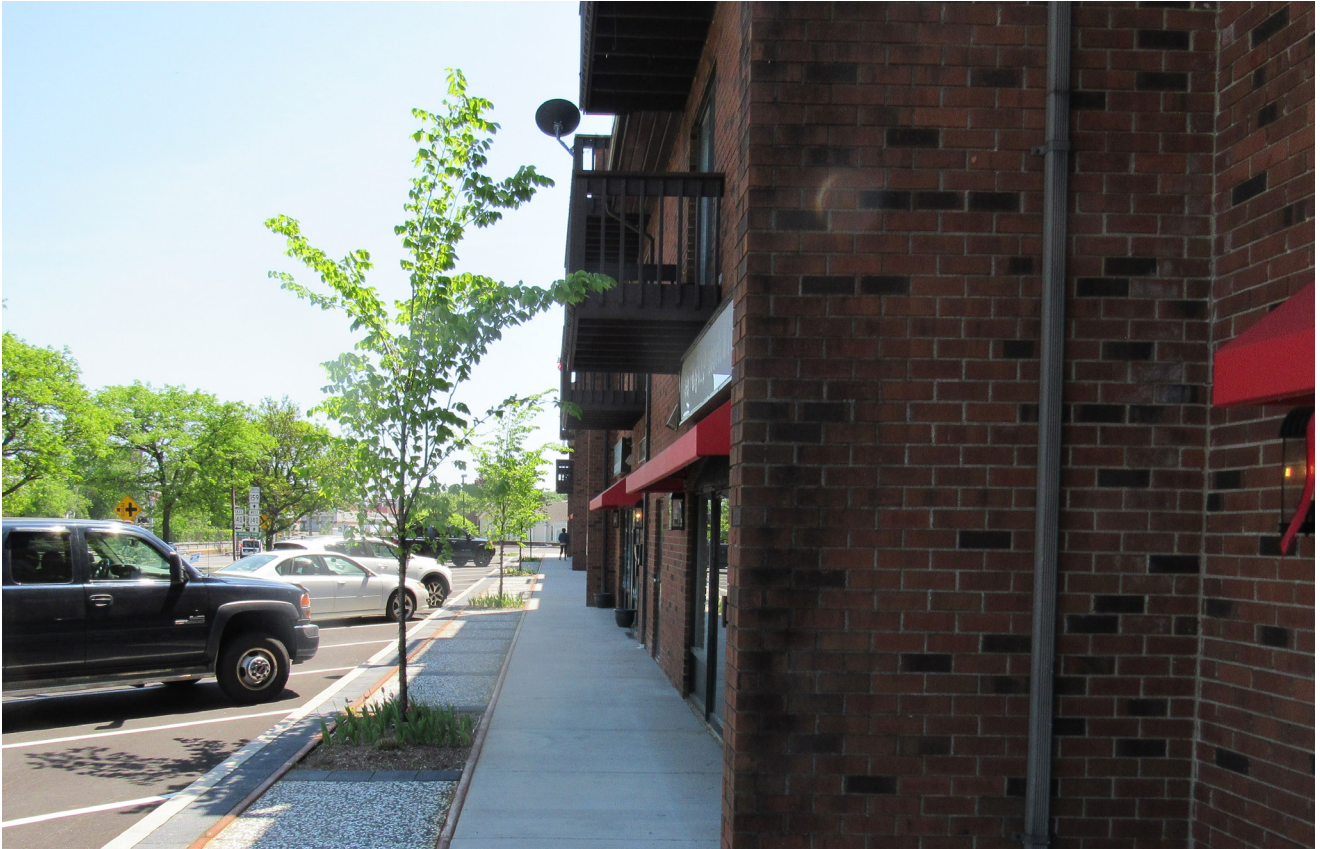
Streetscape Improvements along Main Street. Ongoing streetscape improvements in the future station area aim to create a welcoming environment for pedestrians.
