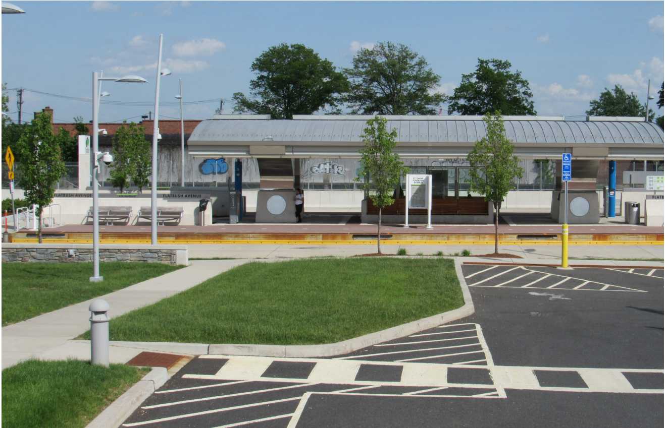
CTfastrak Flatbush Avenue Station. CTfastrak station across from the planned CTrail West Hartford Station.
