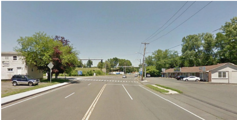
Figure 139: East Street existing conditions
