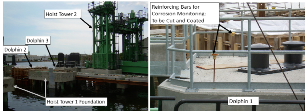
Figure 6.4: Construction of Ferry Terminal (Courtesy of Maine DOT)
