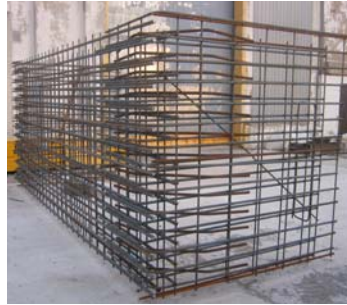
Figure 6.8: Partial Reinforcement (Courtesy of Kistner Concrete Products, Inc.)
