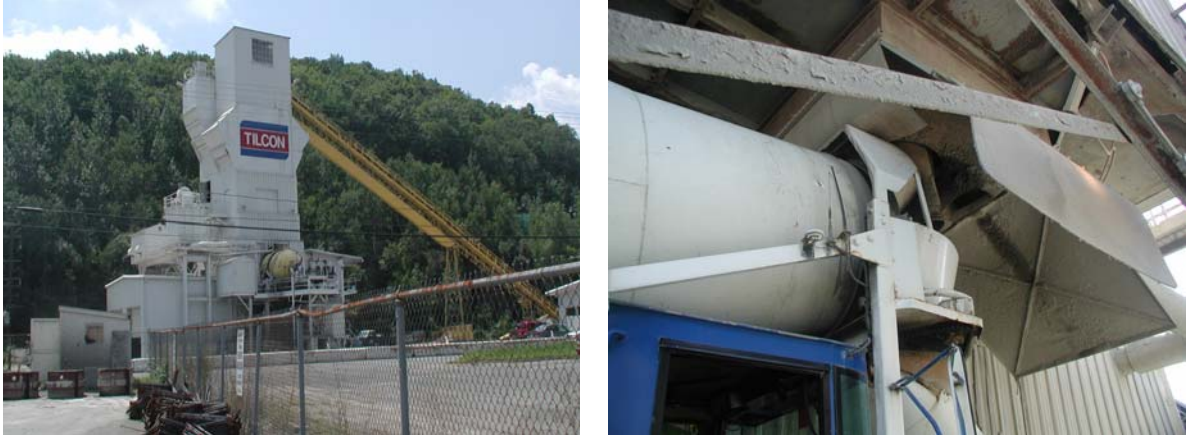
Figure 4.2: Central Batching and Mixing Plant Feeding Truck Mounted Concrete Mixers
