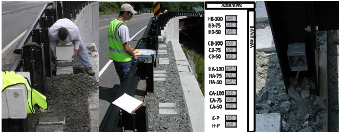
Figure 6.15: Placement of Test Slabs
