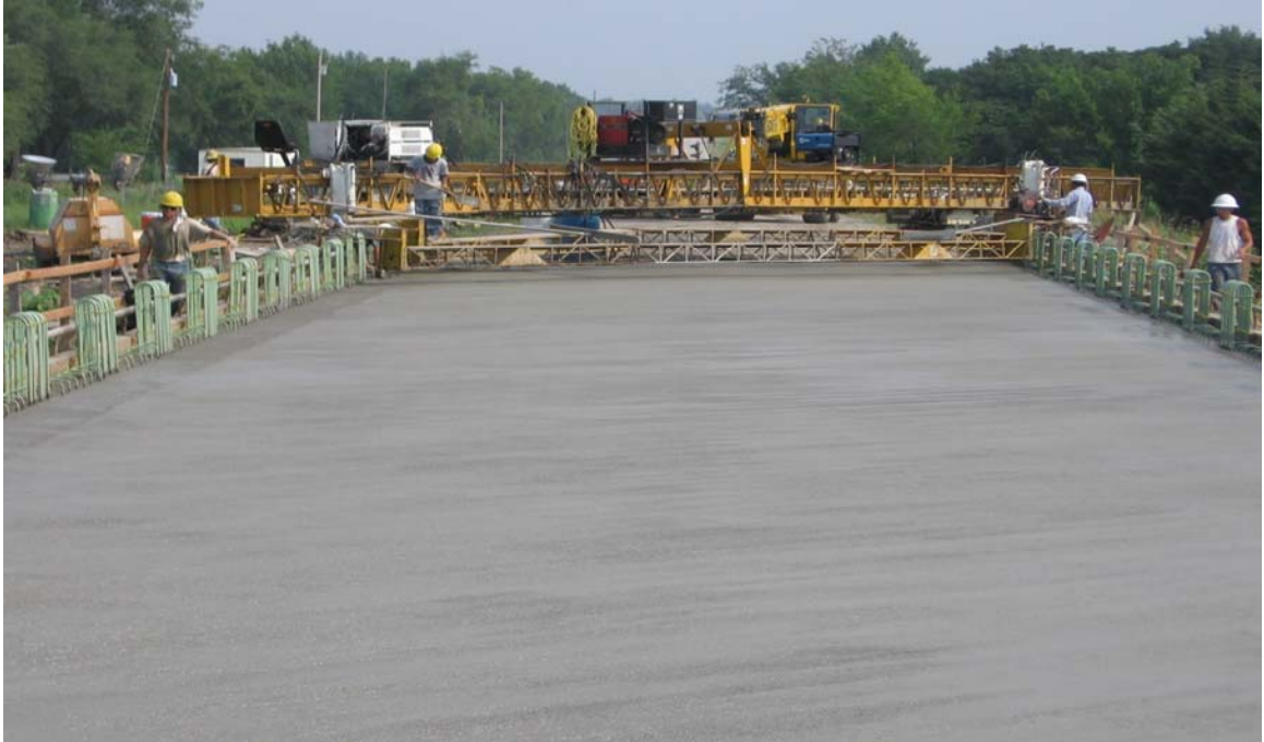
Figure 3.3: Kansas State DOT Hycrete DSS Project (Courtesy of Hycrete Technologies)
