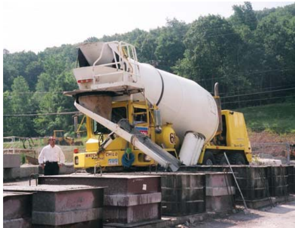
Figure 4.4: Front Discharge Concrete Truck
