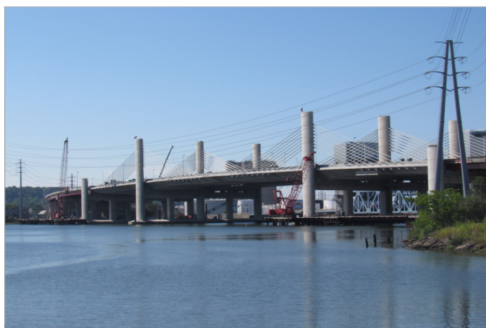
Fig. 2.1 Pearl Harbor Memorial Bridge at I-95
