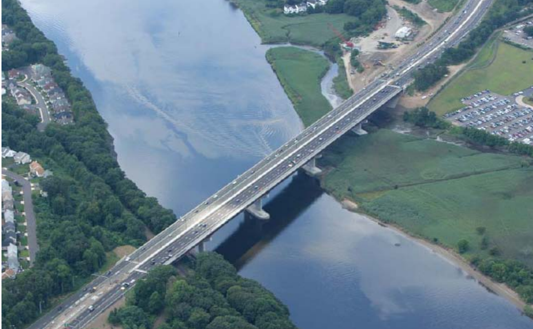
Figure 1. Aerial View of the Sikorsky Bridge
