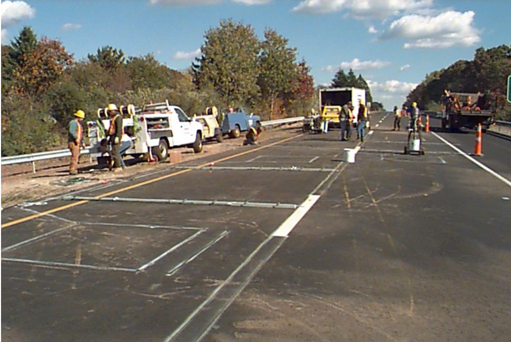
Image 11: Installation of Traffic Monitoring Equipment at CT SPS 9A Site, October 1997
