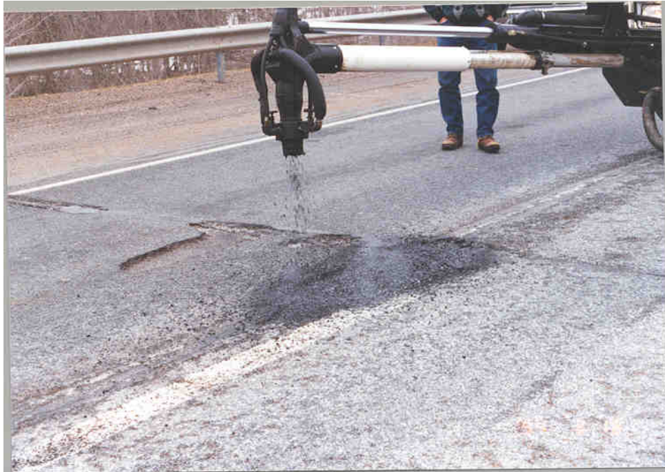
Image 8: Automated Pothole Patcher in Action
