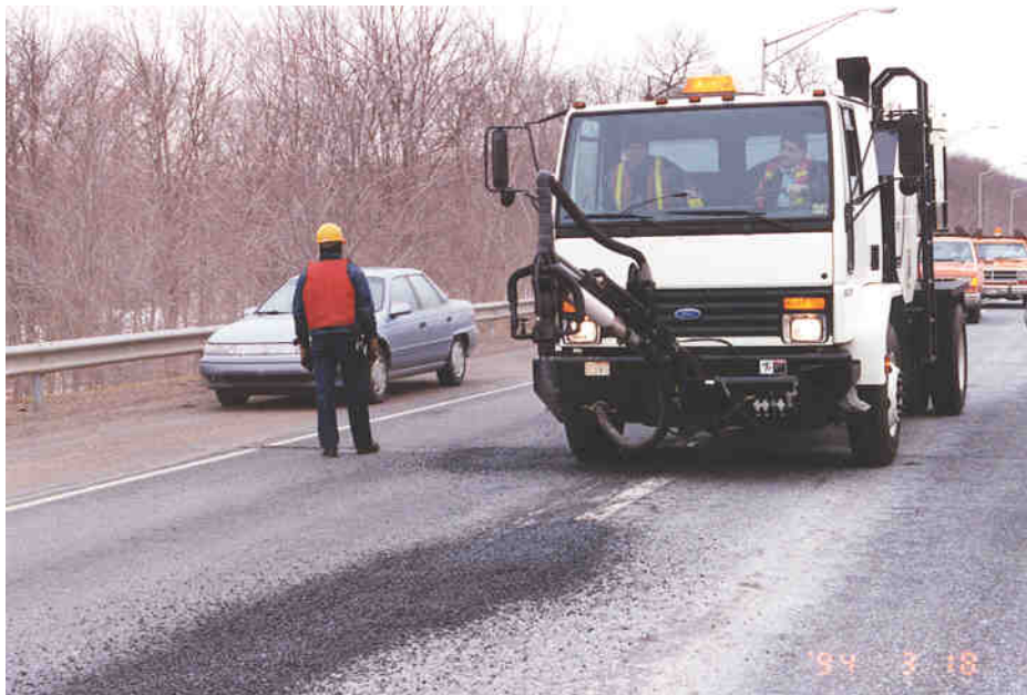
Image 9: Automated Pothole Patcher in Use in Connecticut
