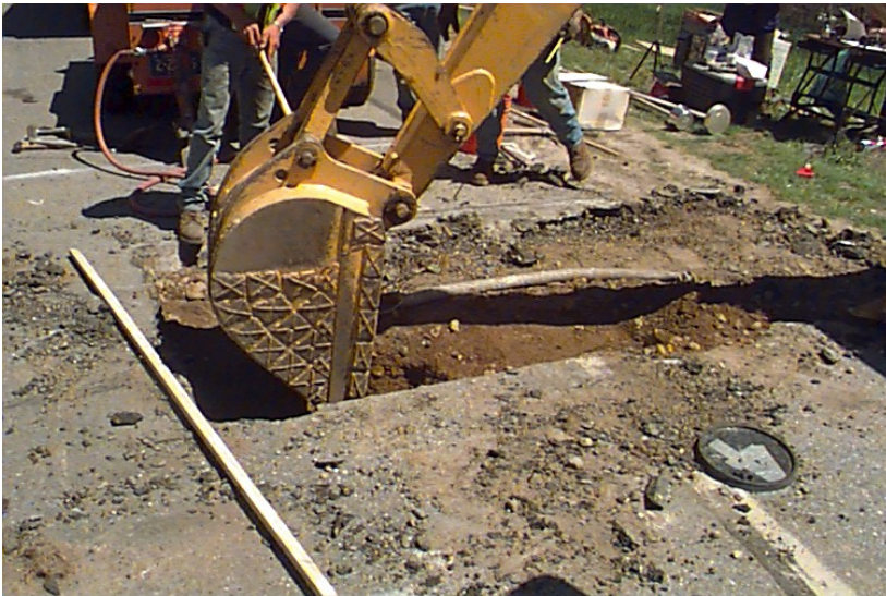
Image 13: Excavation by ConnDOT for Post Experimental Seasonal Monitoring Testing
