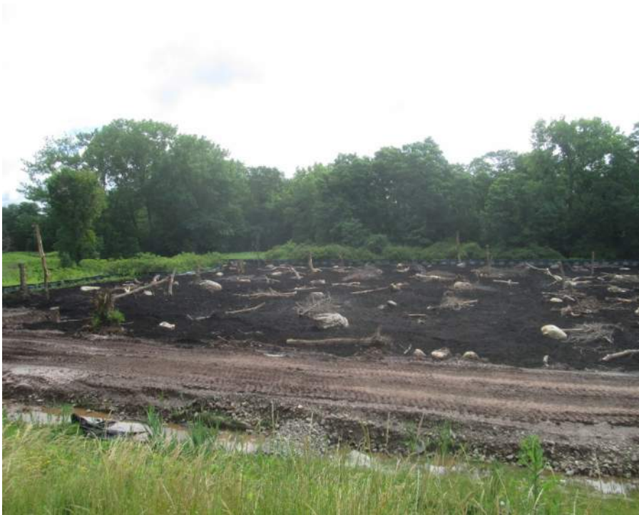
Completed Placement of Top Soil, Boulders & Woody Debris
