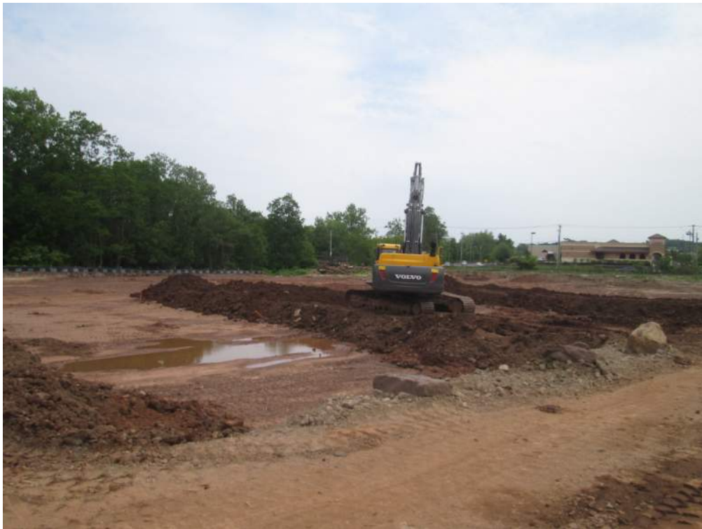
Installation of Haul Roads, Excavation, Placement of Topsoil, Boulders, and Wood Debris
