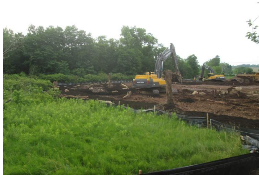
Installation of Haul Roads, Excavation, Placement of Topsoil, Boulders, and Wood Debris
