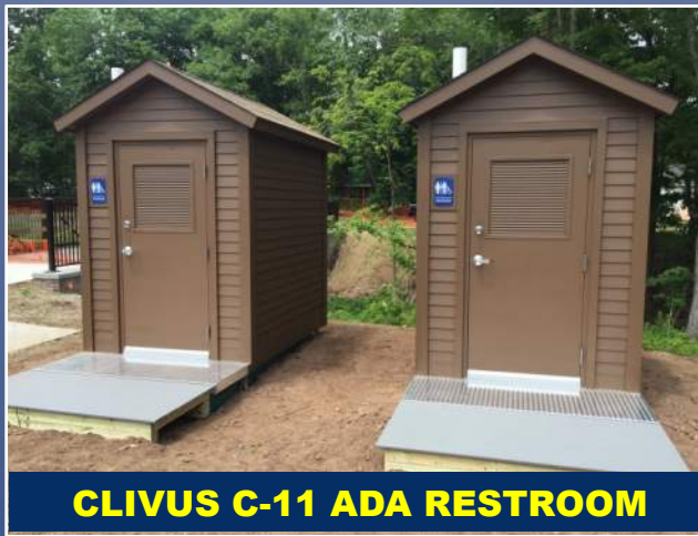
5. INSTALL FULLY ASSEMBLED UNITS
