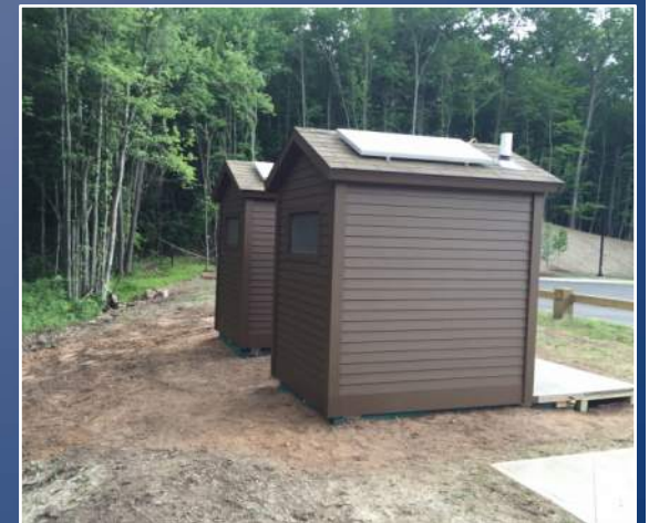
6. GRADING AROUND RESTROOMS
