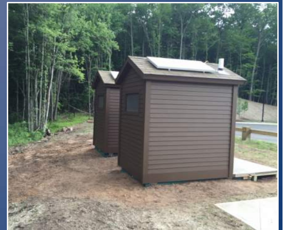
6. GRADING AROUND RESTROOMS
