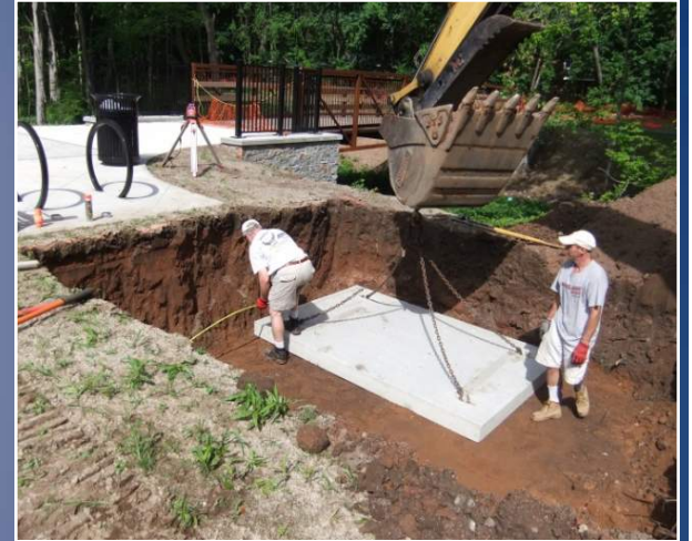
3. PLACE 6" CONCRETE SLABS
