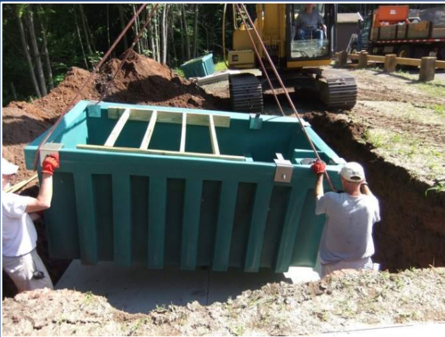
4. INSTALL COMPOSTING CHAMBER
