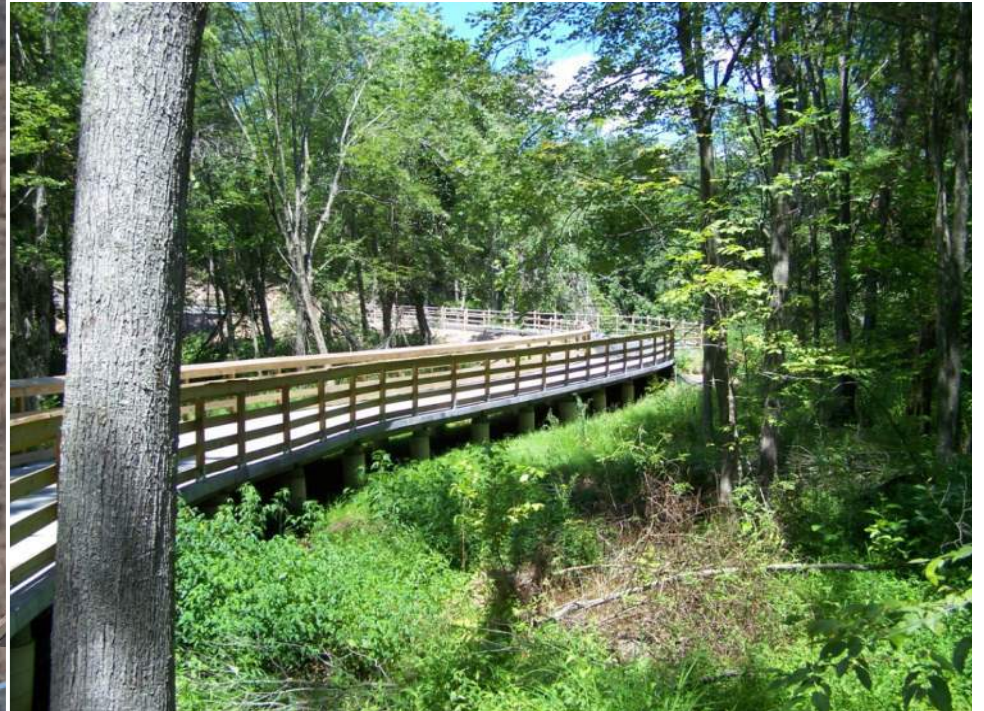
Precast Concrete Pier and Boardwalk System
