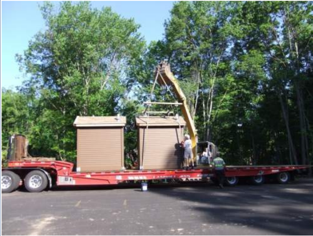
1. ASSEMBLED OFF SITE AND DELIVERED
