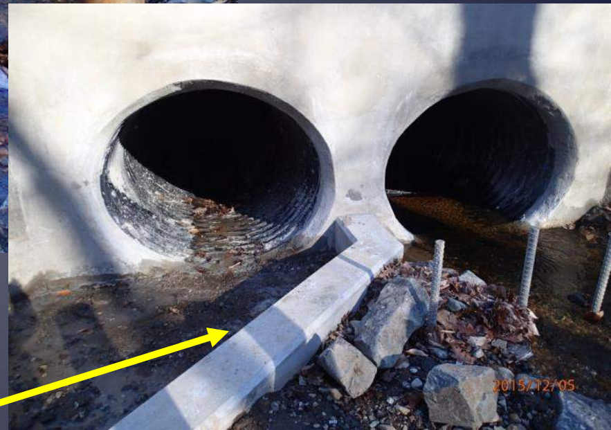
Diversion wall: average daily flows directed into baffled culvert. Flood flows conveyed into both culverts.
