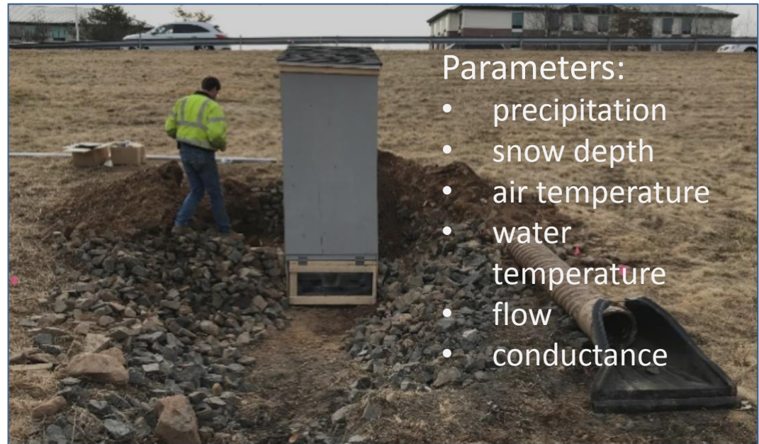
CTDOT Photo of USGS building an outfall monitoring station in Glastonbury
