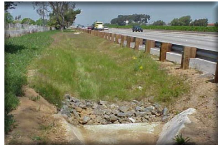
Grassed Channel (Biofilter Swale). Structural BMP Specifications for the Massachusetts Stormwater Handbook. Vol. 2 Chap. 2. Massachusetts Department of Environmental Protection. Retrieved from https://www.mass.gov/files/documents/2016/08/qi/v2c2.pdf
