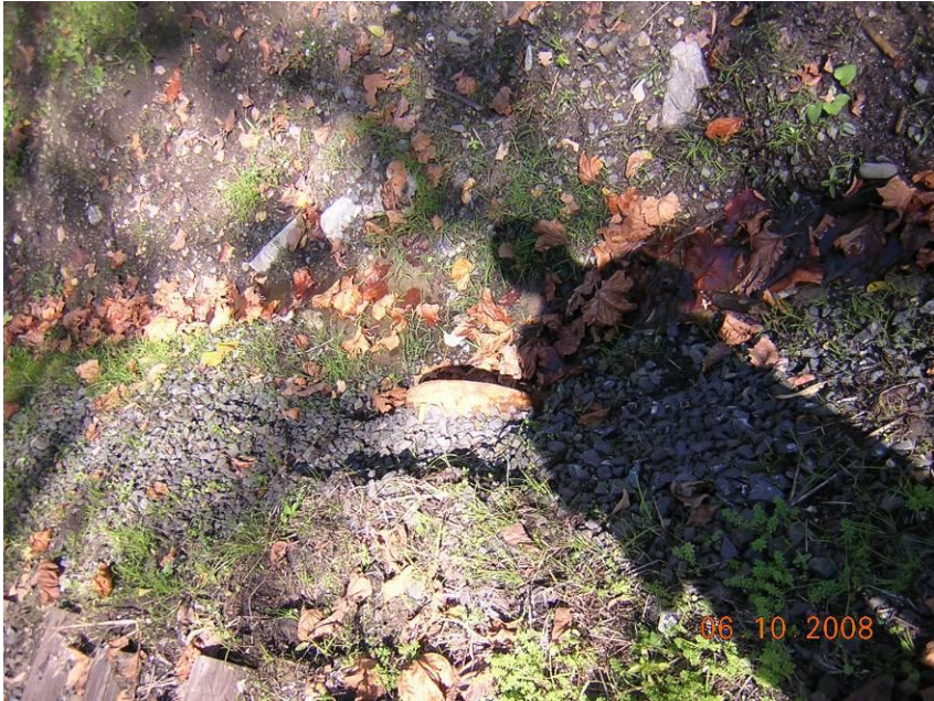
MP 4.9 (E) HRR – Drainage by tracks
