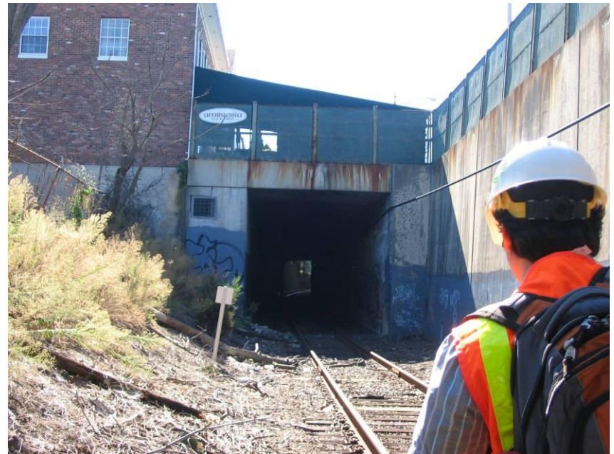
MP 1.5 (S02) MNR – North entrance of tunnel
