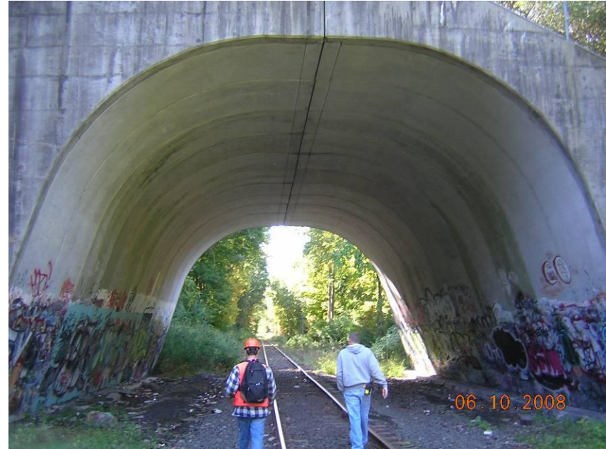
MP 1.67 (S) HRR – OH Gray's Bridge Rd.
