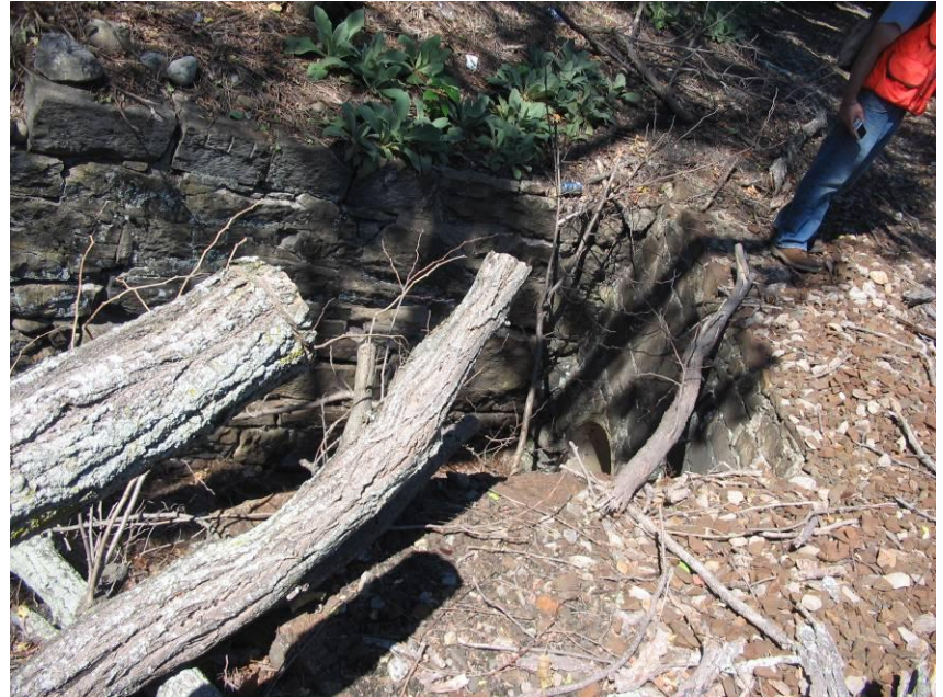
MP 3.85 (W) MNR – RCP under tracks
