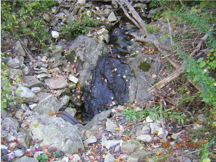
MP 1.91 (E) HRR – Drainage Pipe
