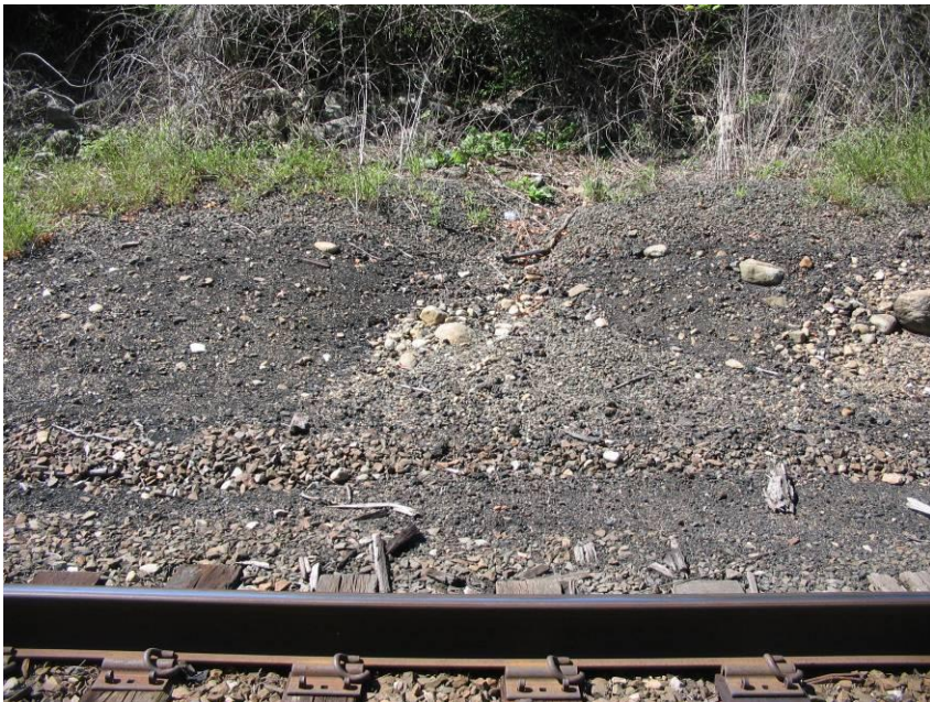
MP 4.90 (W) – Drainage by tracks
