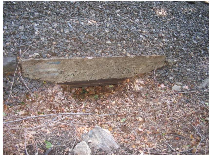
MP 4.36 (E) MNR – Culvert under tracks
