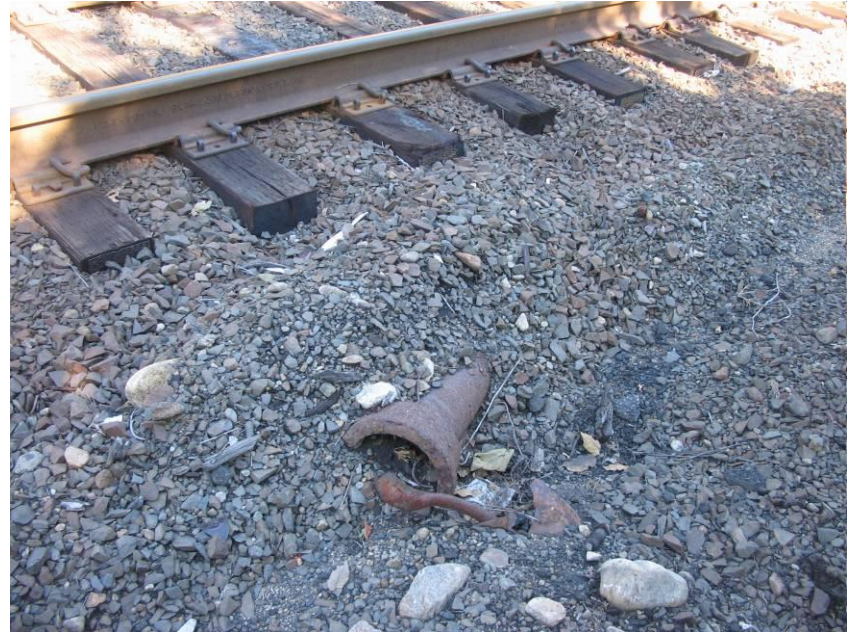
MP 1.1 (SW) MNR – Drainage by tracks
