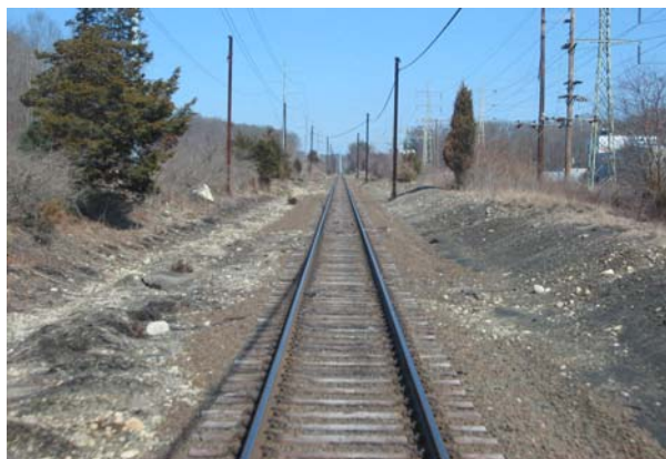
Utility lines in proximity of tracks (MP 5.30)
