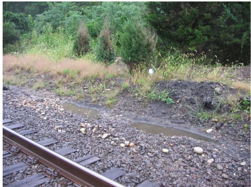
MP 5.1 (E) MNR – Drainage by tracks
