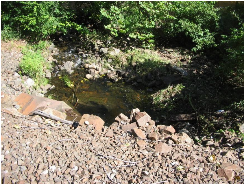
MP 3.98 (E) MNR – Drainage under tracks
