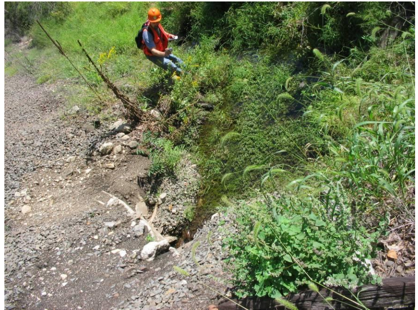
MP 7.7 (E) MNR - Culvert
