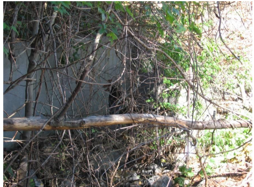
MP 3.42 (NW) MNR – RCP west of tracks
