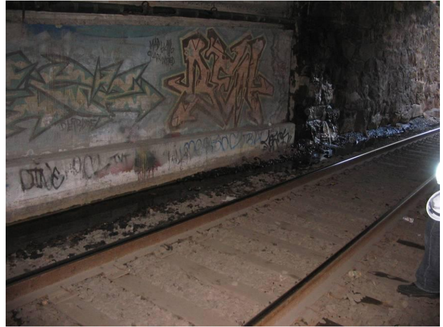
MP 1.4 (SE01) MNR – Drainage at south entrance of tunnel
