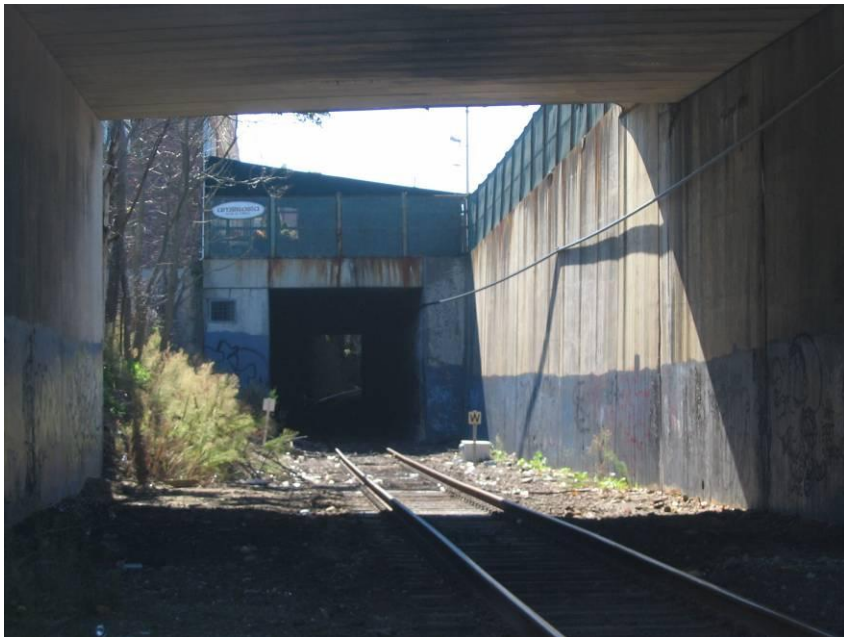
MP 1.5 (S03) MNR – North entrance of tunnel
