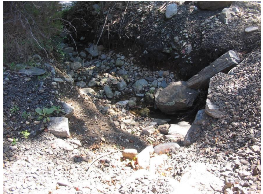
MP 4.43 (W) MNR – Culvert under tracks
