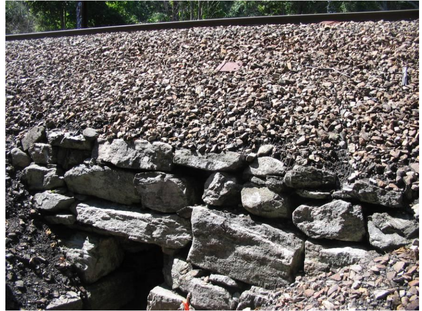
MP 4.75 (E02) MNR – Culvert under tracks
