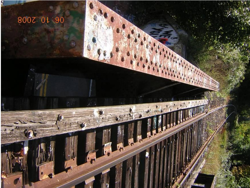
MP 2.51 (S) HRR – UG Junction Rd.
