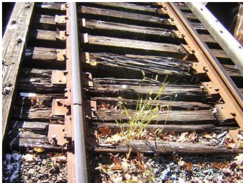
Figure 13 - Junction Rd (HRR – Berkshire Line MP 2.51)
