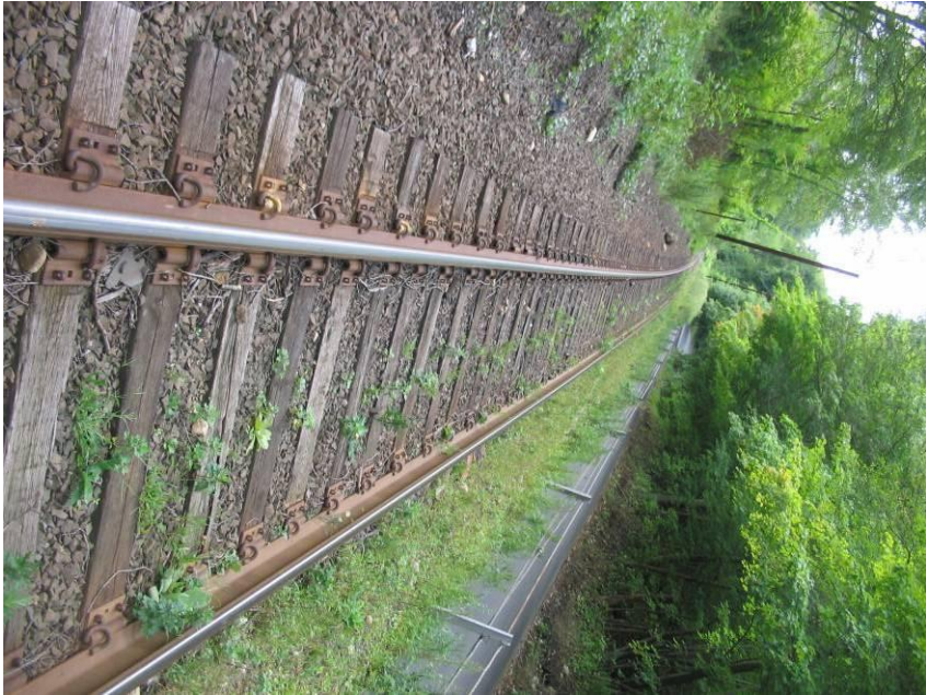
MP 15.6 (S01) MNR – OH fiber optics cable crossing
