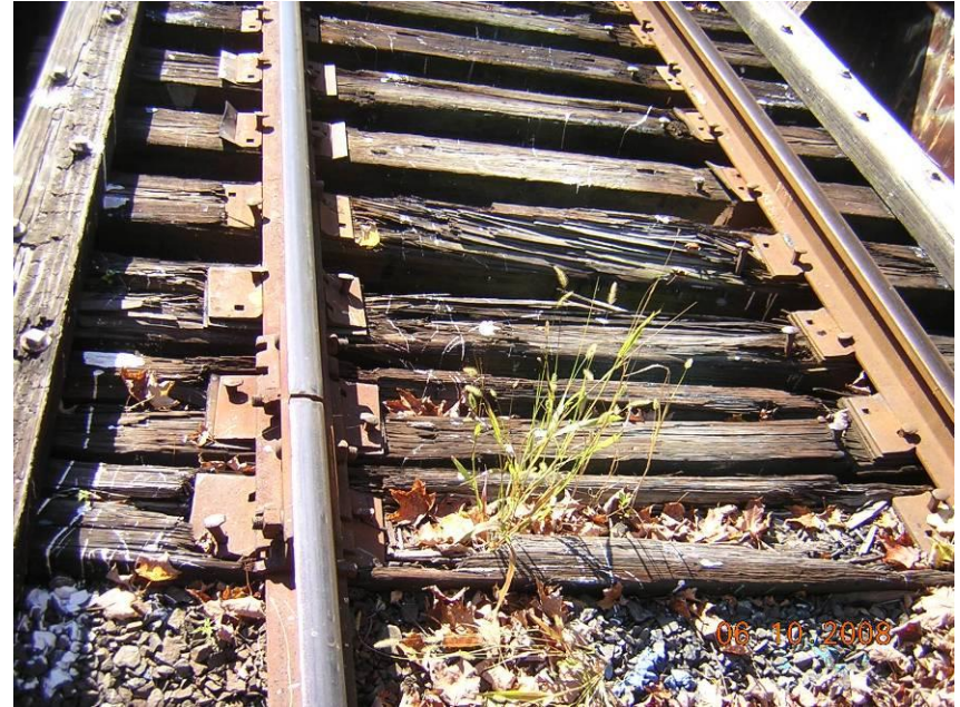
MP 2.51 (S) HRR – UG Junction Rd.
