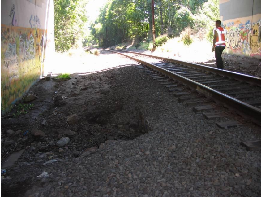
MP 4.3 (SW) MNR – Drainage under OH Route 7
