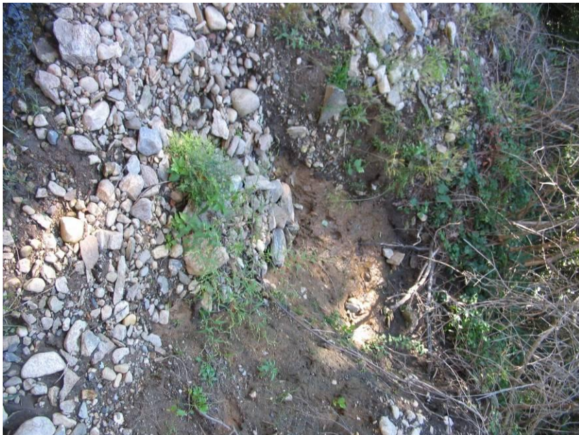
MP 4.60 (W03) MNR – Drainage by tracks
