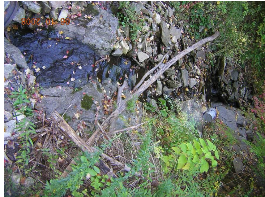
MP 1.91 (E) HRR – Drainage Pipe
