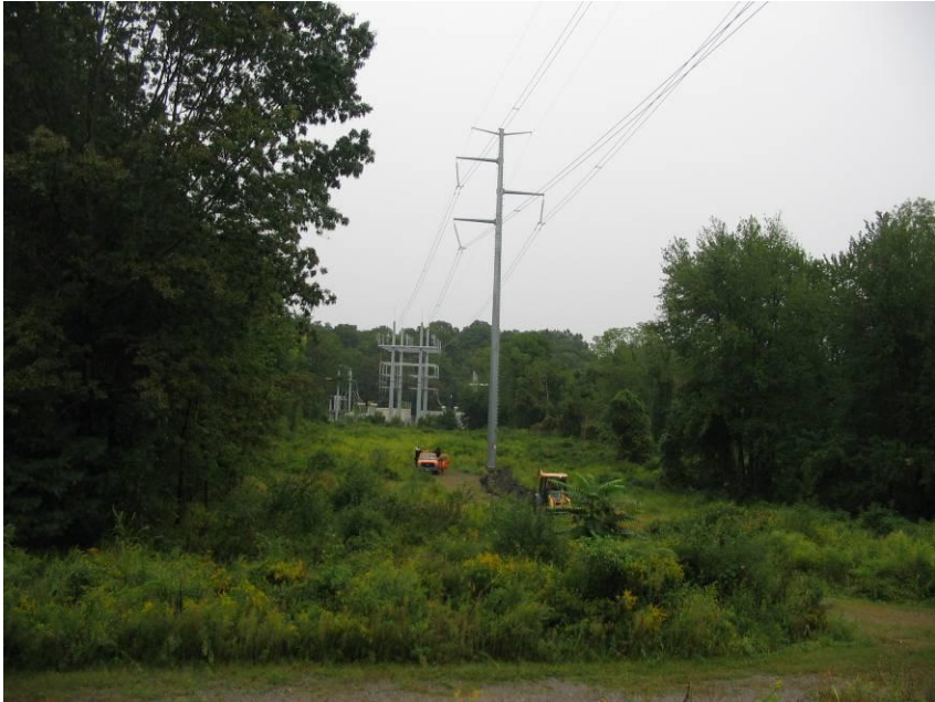
MP 5.59 (E) MNR – OH Power lines
