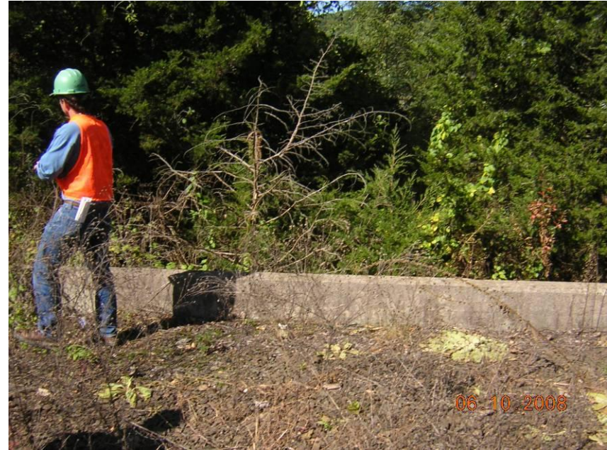
MP 80.0/0.0 (E) Maybrook/HRR – Concrete Structure East of Trks
