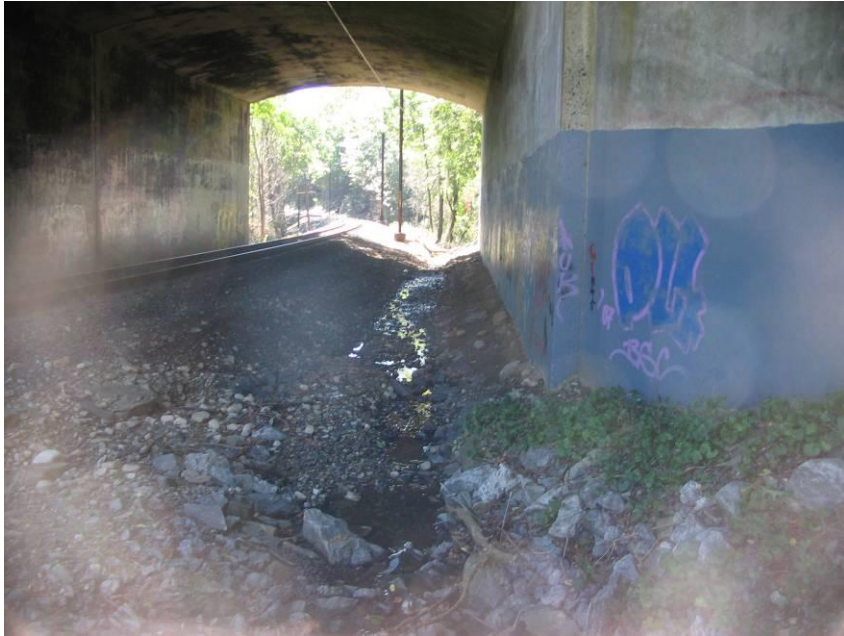
MP 3.42 (SW) MNR – Drainage under OH Merritt Parkway
