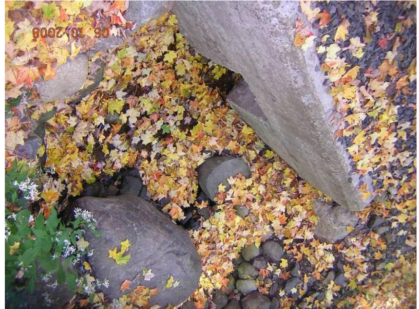
MP 3.7 (E) HRR – Culvert
