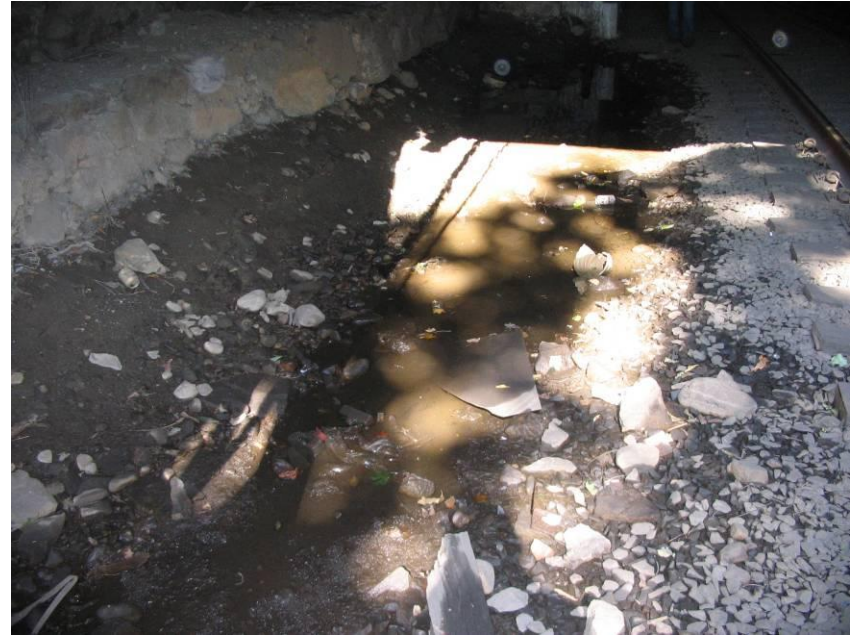
MP 1.4 (NW01) MNR – Drainage at south entrance of tunnel
