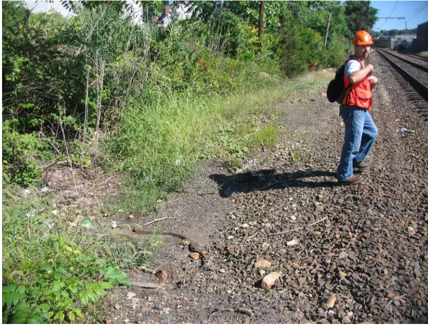
MP 0.7 (NW) MNR – Drainage by tracks
