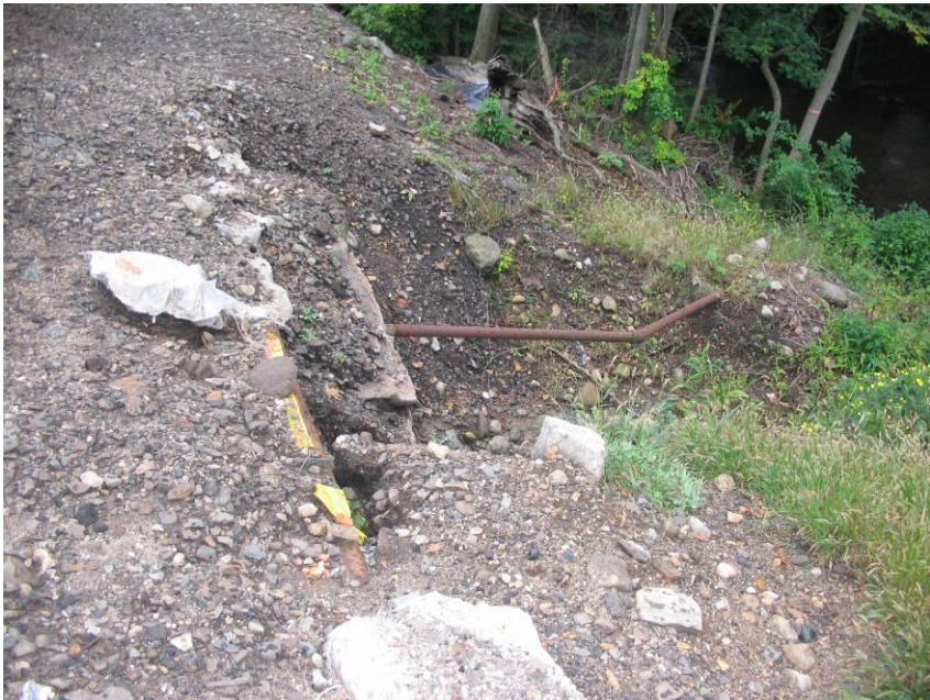
MP 7.25 (SE02) MNR - Culvert
