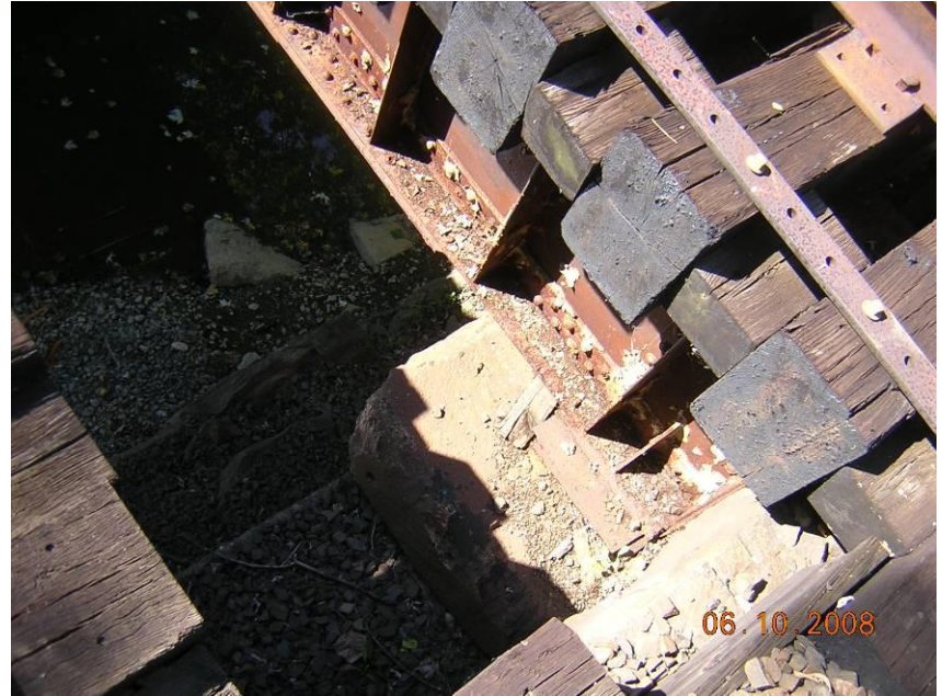
MP 79.65 UG Still River (Maybrook Line)
