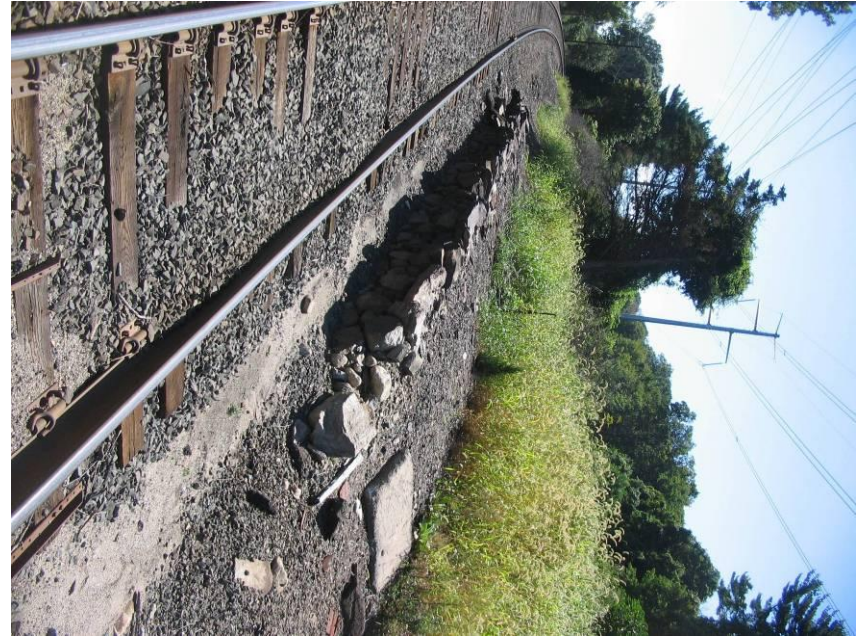
MP 4.93 (S02) MNR – Stone wall and OH utilities at Kent Rd.
