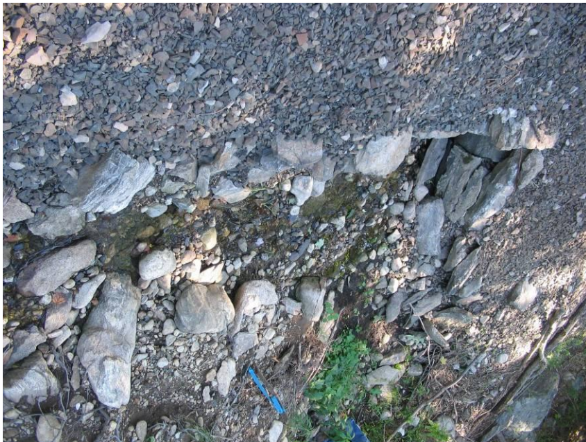
MP 4.43 (E) MNR – Culvert under tracks
