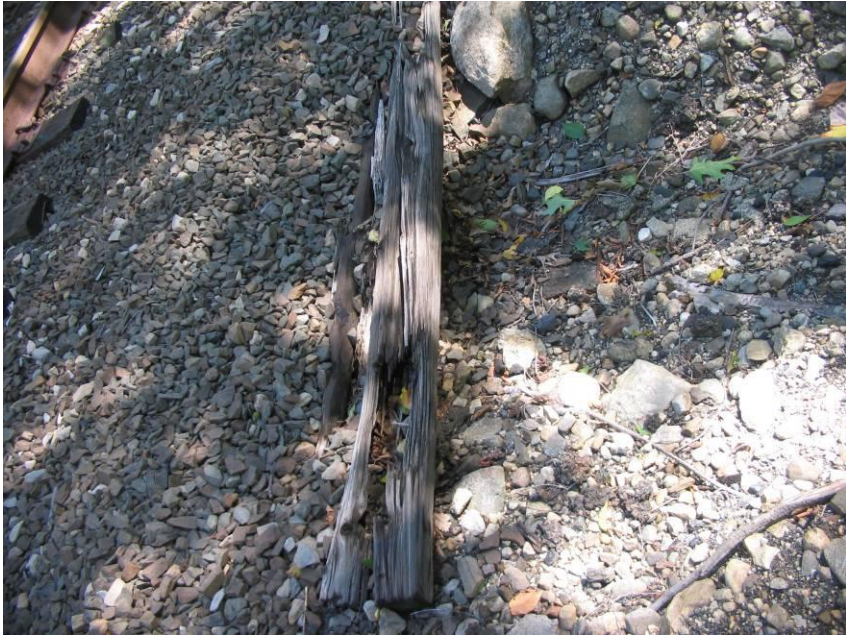
MP 13.5 (W02) Drainage under tracks
