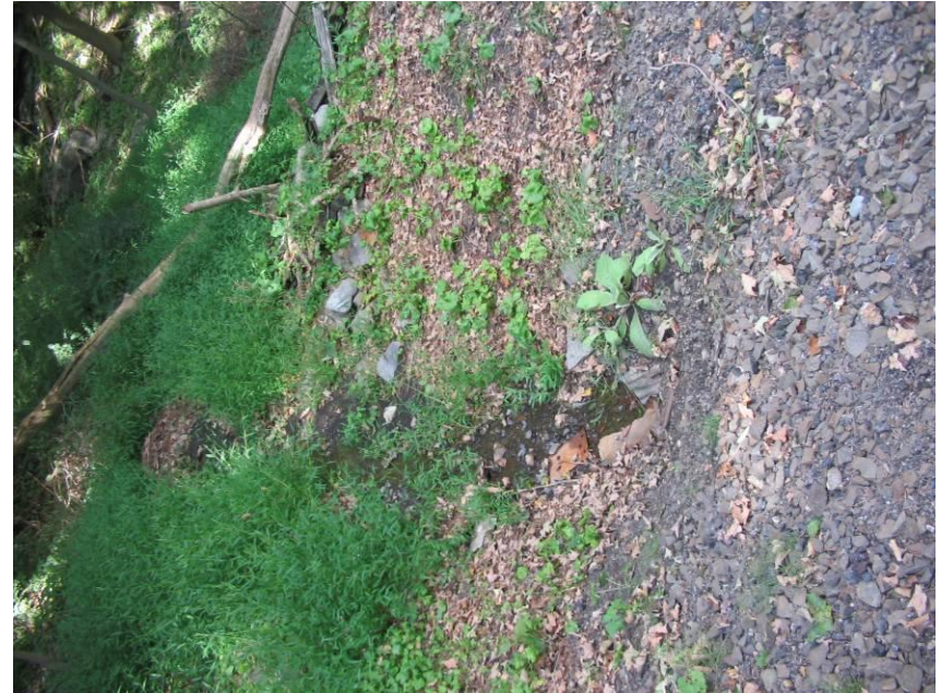
MP 14.9 (E) MNR – Drainage under tracks
