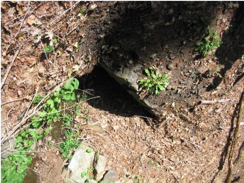
MP 14.9 (W) MNR – Culvert
