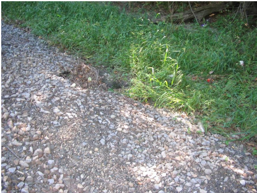
MP 4.31 (SW) MNR – Drainage by tracks
