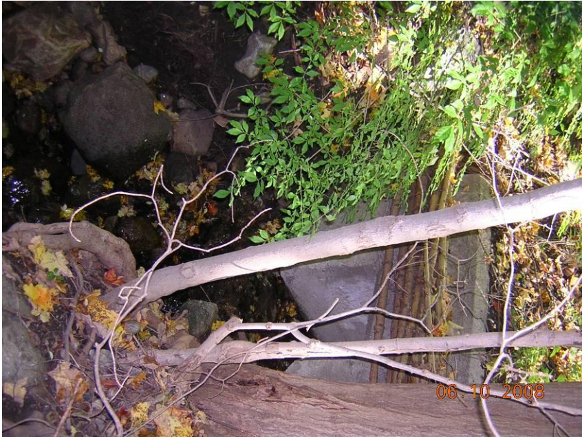
MP 3.7 (W) HRR – Culvert
