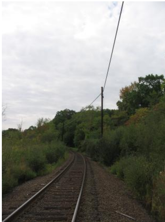
Figure 1 - Typical existing cat. poles supporting fiber optic cable (MNR MP 15.7)
