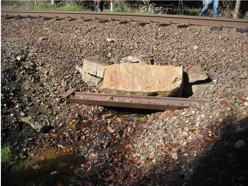
MP 9.2 (E) MNR – Drainage under tracks
