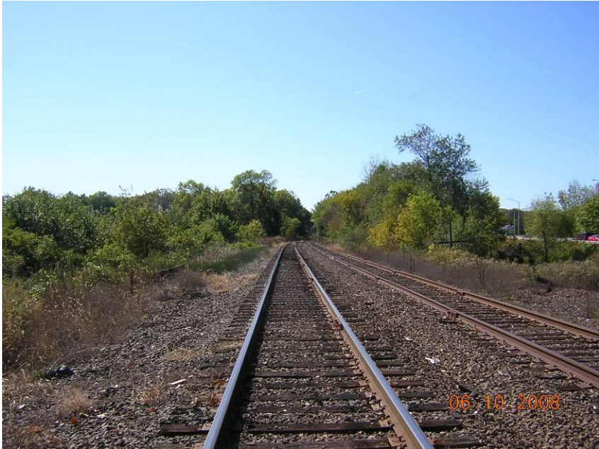
MP 79.8 (S) Maybrook Line
