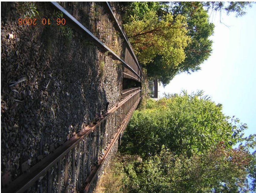
MP 79.65 (S) UG Still River (Maybrook Line)
