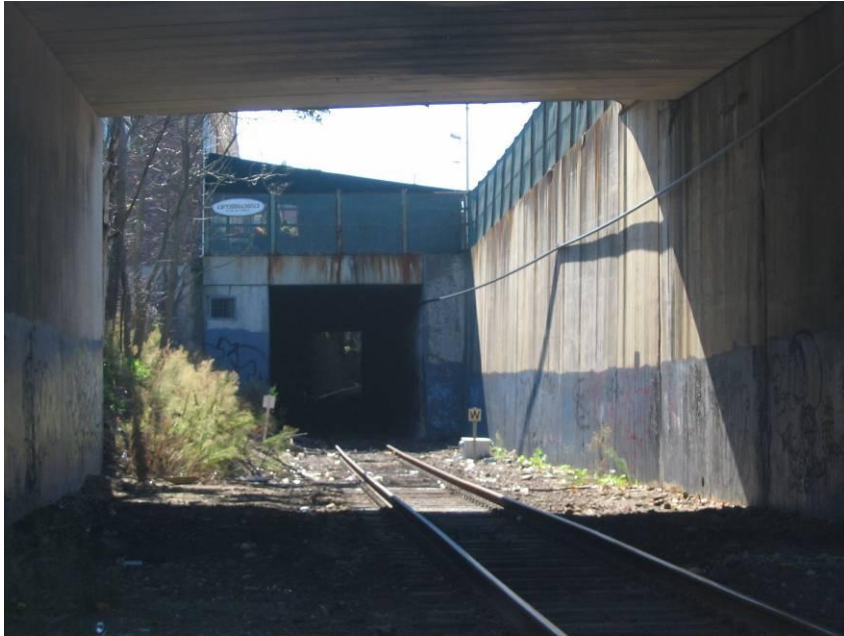
MP 1.5 (S01) MNR – North entrance of tunnel
