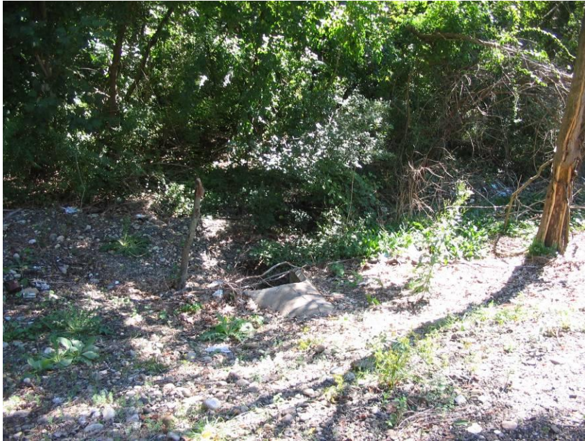
MP 3.3 (E) MNR – RCP under tracks
