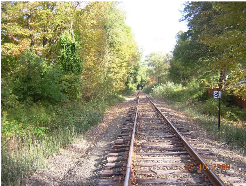
MP 8.0 (N) HRR – Mile Marker
