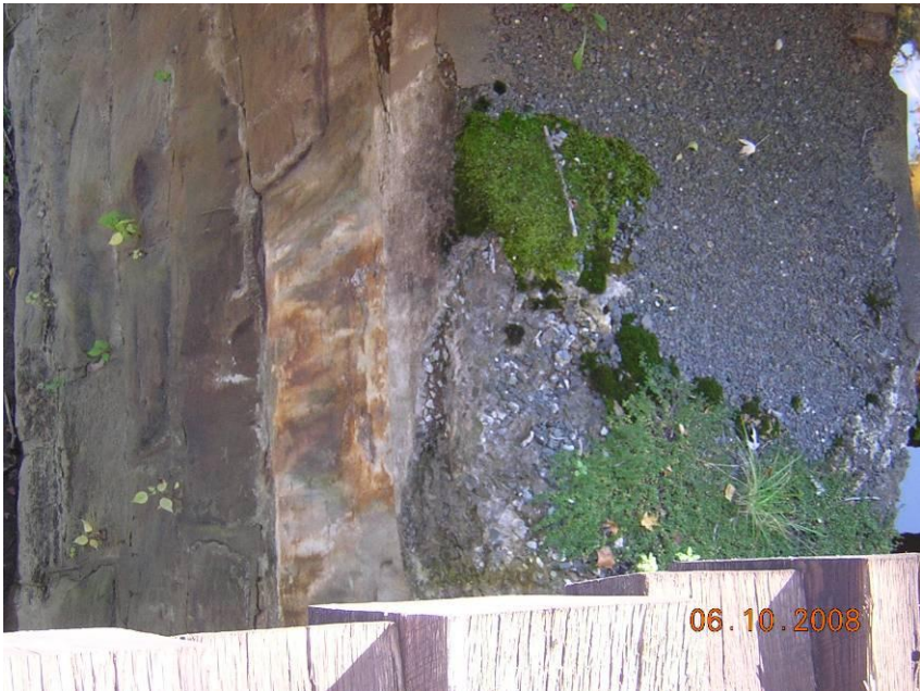
MP 79.65 UG Still River (Maybrook Line)
