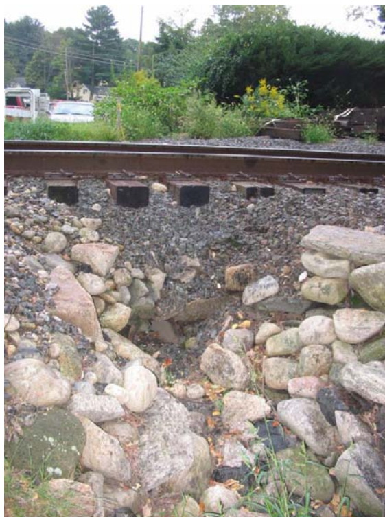
Typical Culvert Crossing (MNR MP 6.8)
