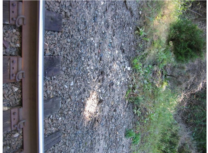
MP 4.31 (SE) MNR – Drainage by tracks
