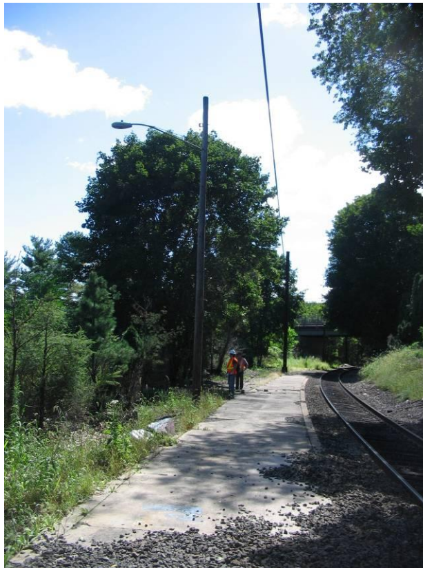
Figure 20 - Existing platform. Proposed location for Georgetown Station. (MNR MP 11.9)
