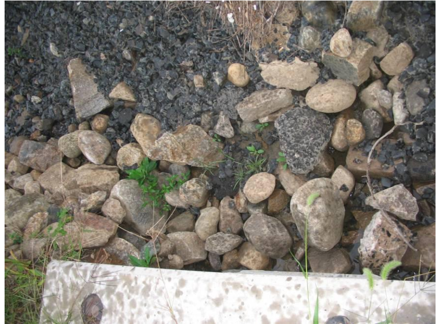
MP 7.17 (NE) MNR - Culvert
