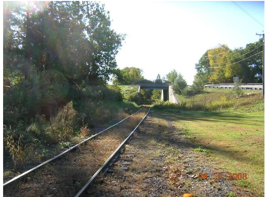
MP 4.5 (S) HRR – OH Whisconier Rd.
