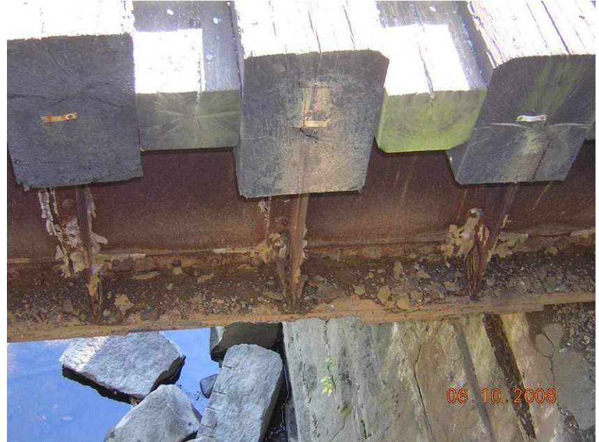
MP 79.65 UG Still River (Maybrook Line)
