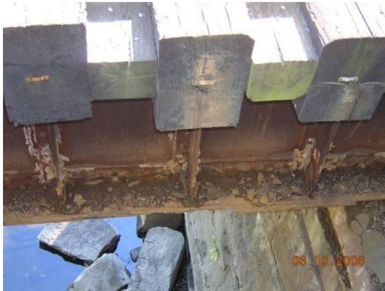
Figure 18 - MP 79.65 UG Still River (TILCON/Maybrook)
