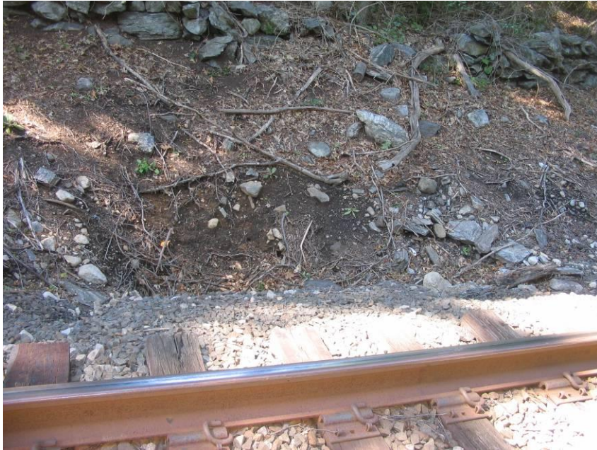
MP 4.36 (W01) MNR – Culvert under tracks
