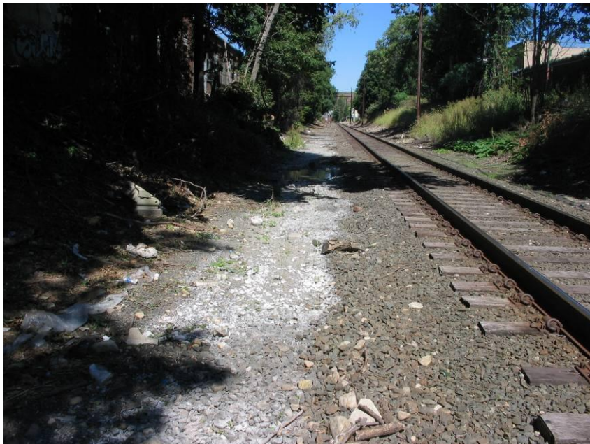
MP 2.7 (NW) MNR – Drainage by tracks
