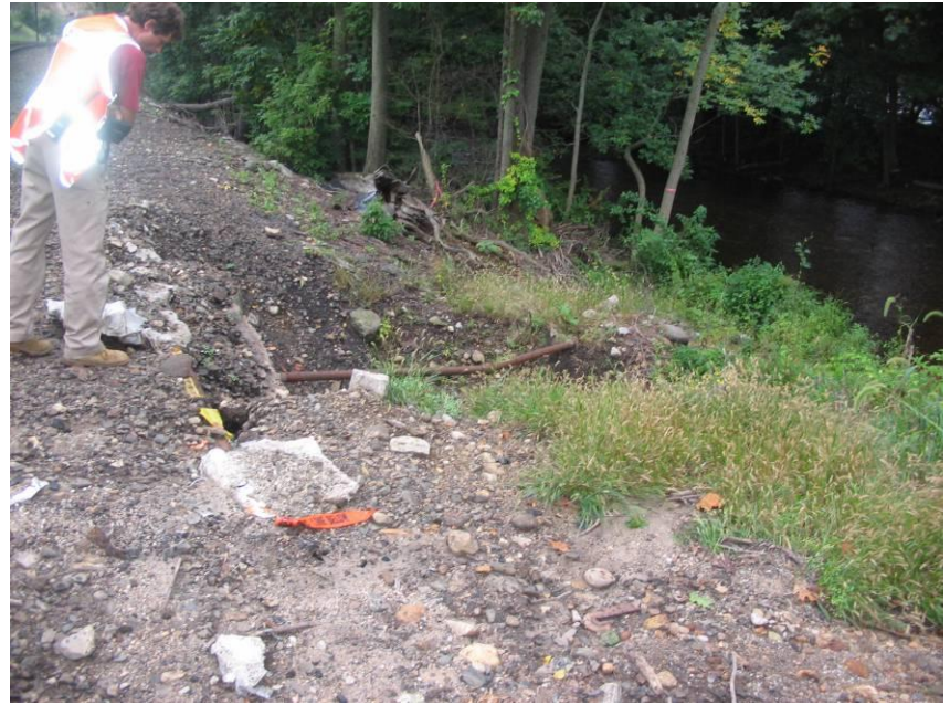
MP 7.25 (SE01) MNR – Culvert
