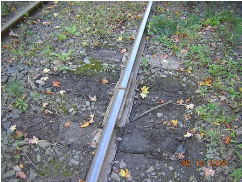
MP 1.67 (N) HRR – State of Trks by Gray's Bridge Rd.
