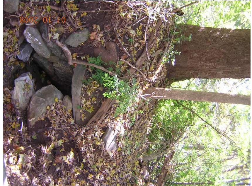
MP 4.6 (W) HRR – Culvert west of tracks
