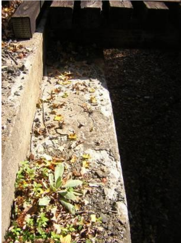
Figure 12 - Cattle Pass (HRR – Berkshire Line MP 2.96)
