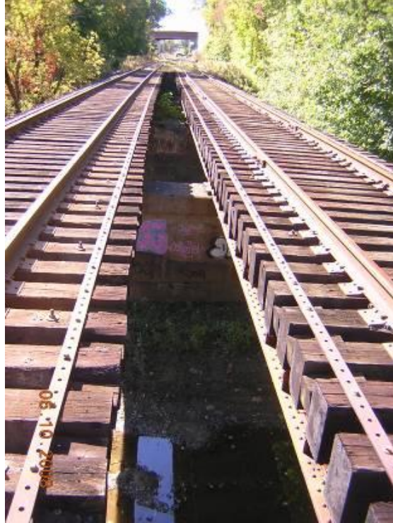
Figure 16 Still River (HRR - TILCON/Maybrook Line MP 79.65)
