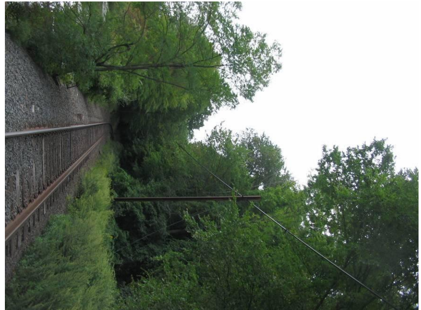
MP 15.4 (S) MNR – OH fiber optics cable crossing
