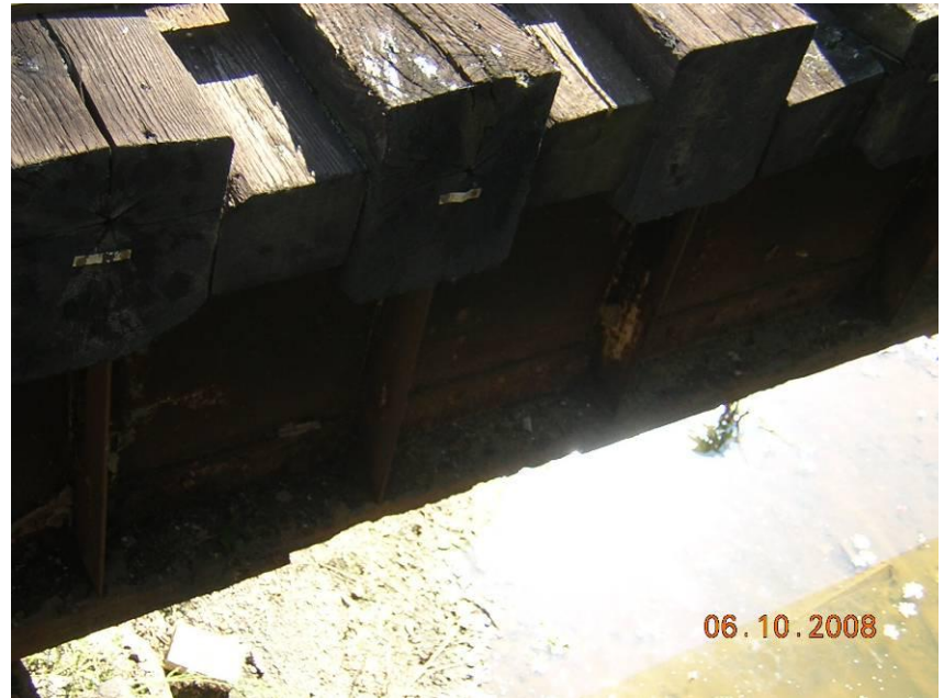
MP 79.65 UG Still River (Maybrook Line)
