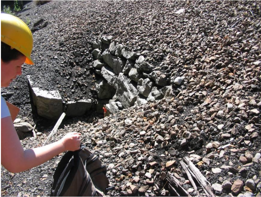
MP 4.75 (E01) MNR – Culvert under tracks
