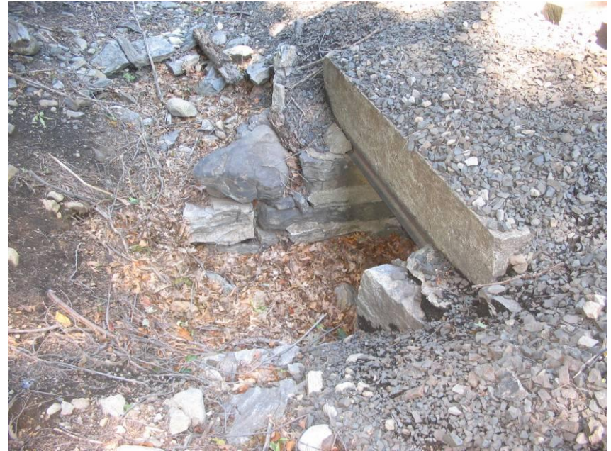
MP 4.36 (W02) MNR – Culvert under tracks
