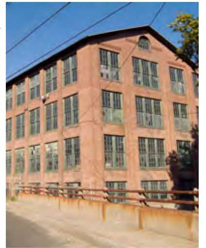
Georgetown - Existing Structure
