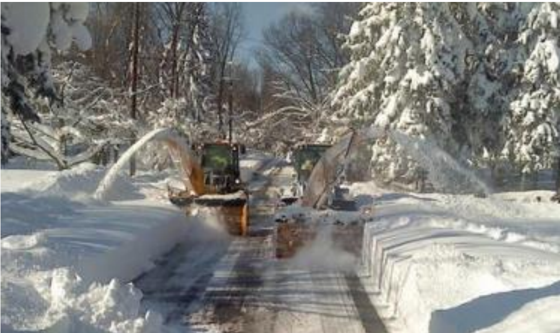
CTDOT personnel opening roadway due to an extreme weather event
