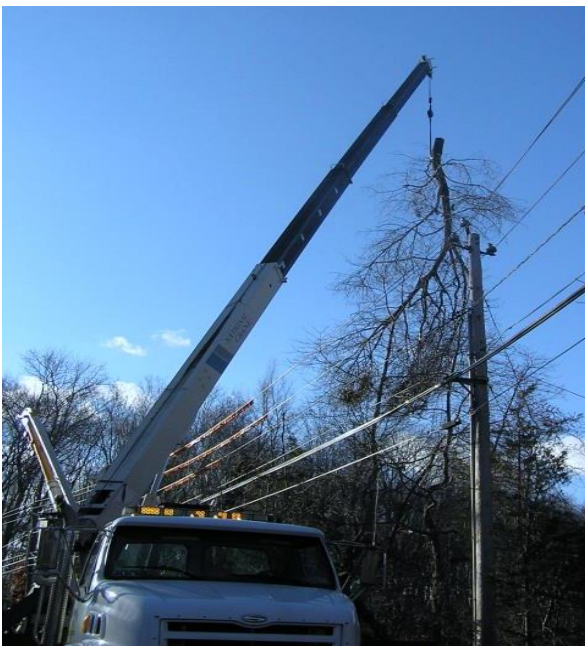
Route 17 Portland - Contractor crane removing tree over utility wires
