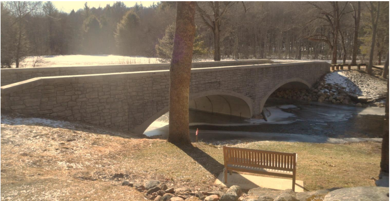
Slopes cleared of brush at Bridge 04731, Stone Mill Road over Fenton River, Mansfield
