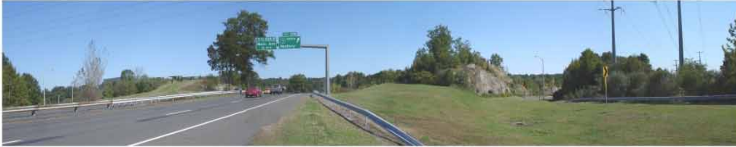
EXISTING CONDITION VIEW B
