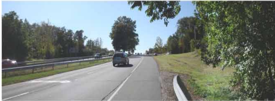
EXISTING CONDITION VIEW H
