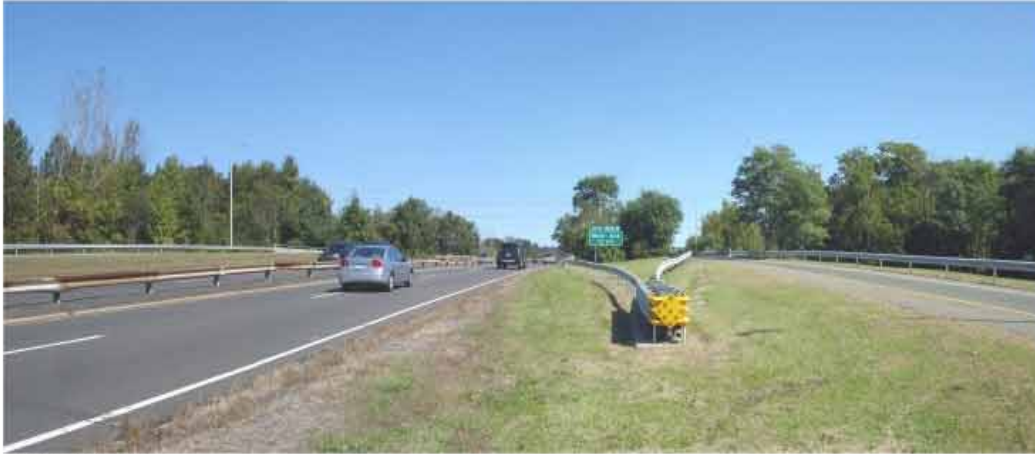
EXISTING CONDITION VIEW A
