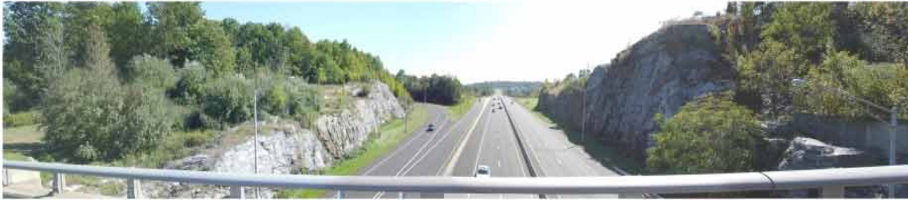
EXISTING CONDITION VIEW C
