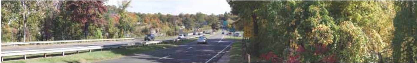
EXISTING CONDITION VIEW E
