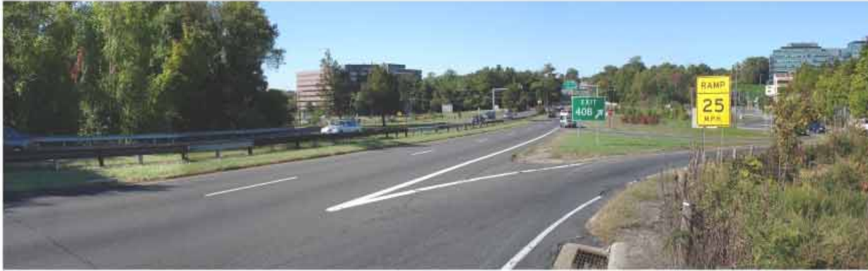
EXISTING CONDITION VIEW F
