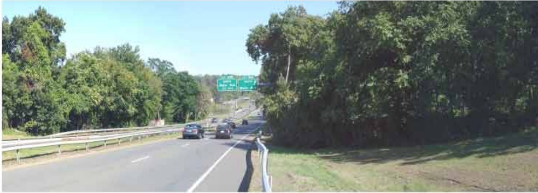
EXISTING CONDITION VIEW D
