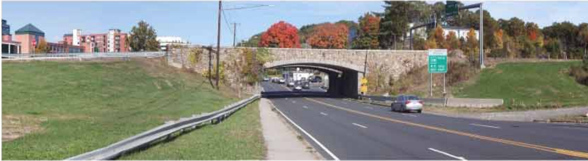
EXISTING CONDITION VIEW G
