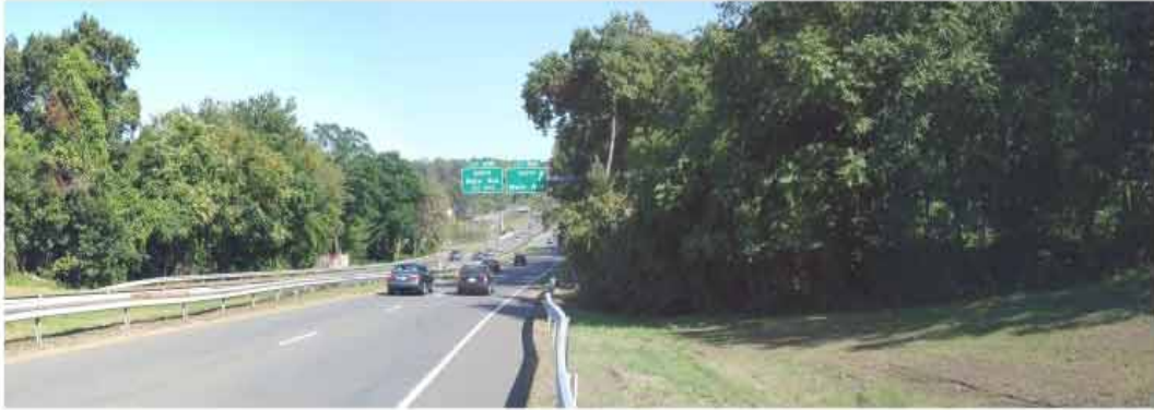
EXISTING CONDITION VIEW D
