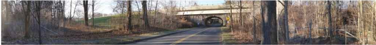
EXISTING CONDITION VIEW S1
