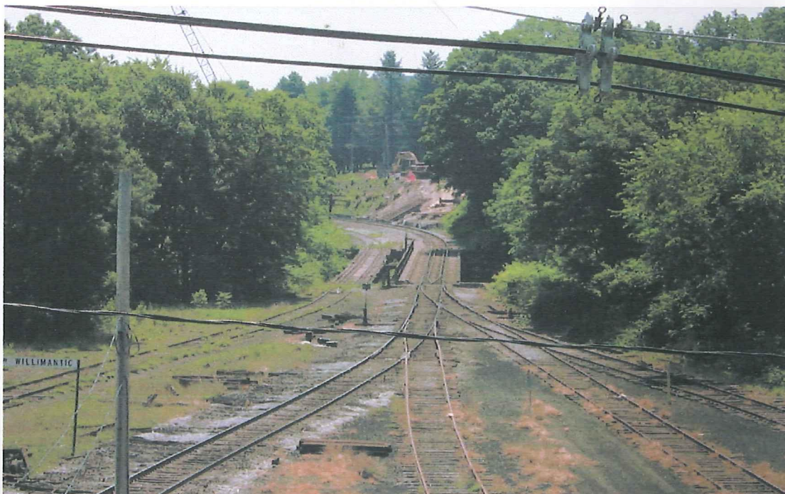
Approach to Bridge, Facing Easterly
