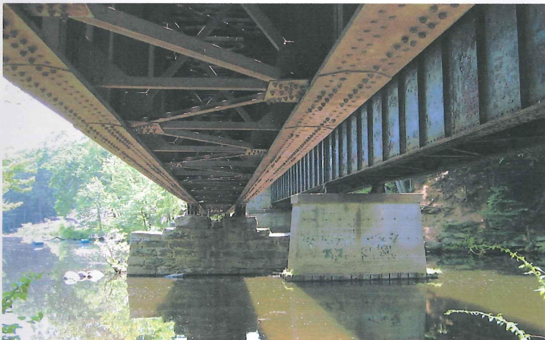
View Under CDOT Track Facing Easterly
