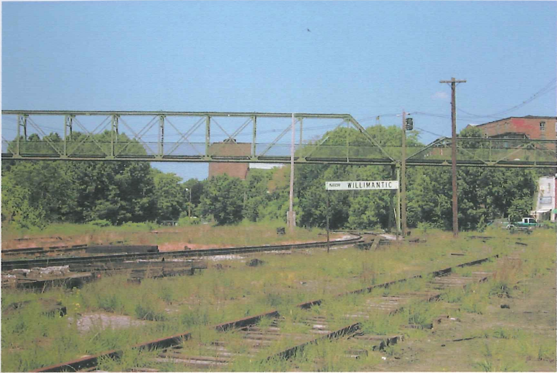
View of Center Span, Looking Easterly
