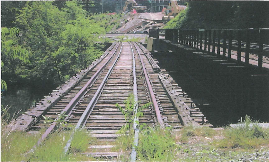
CDOT Track Looking Easterly, Central Vermont Track on Right
