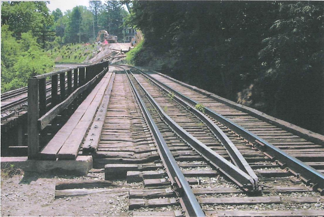
Central Vermont Track, Facing Easterly CDOT Track on Left
