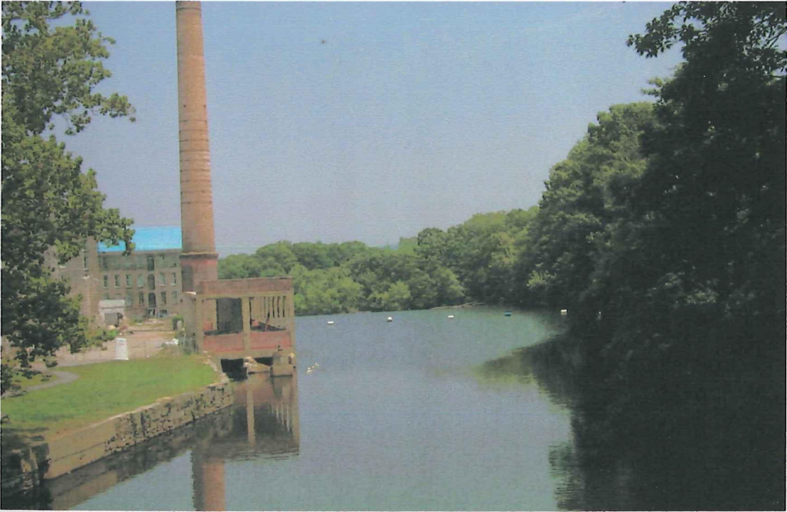
View From Beneath Bridge, Looking Easterly At Willimantic River
