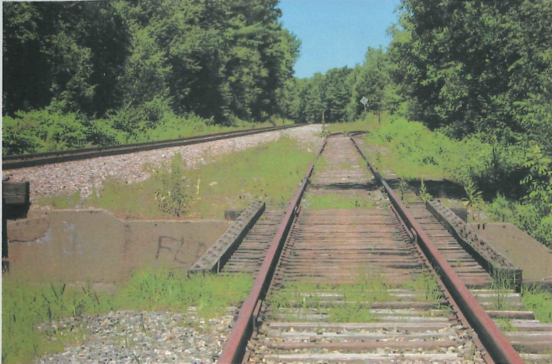
CDOT Track, Looking North Westerly
