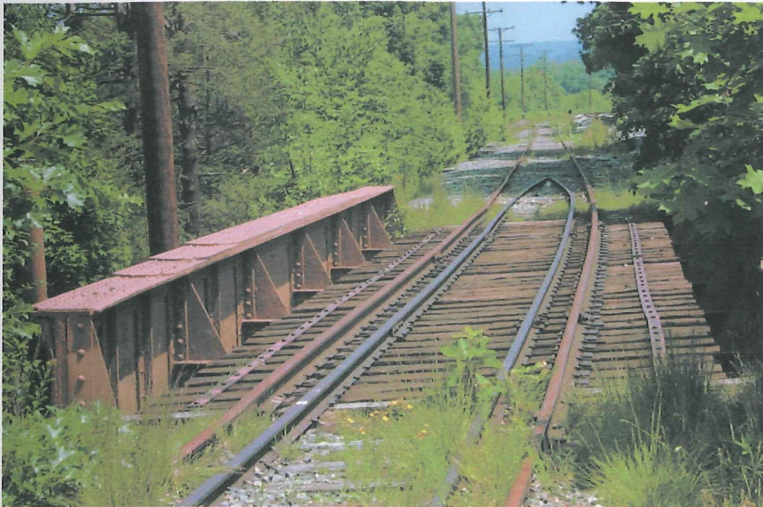
CDOT Track Looking Easterly
