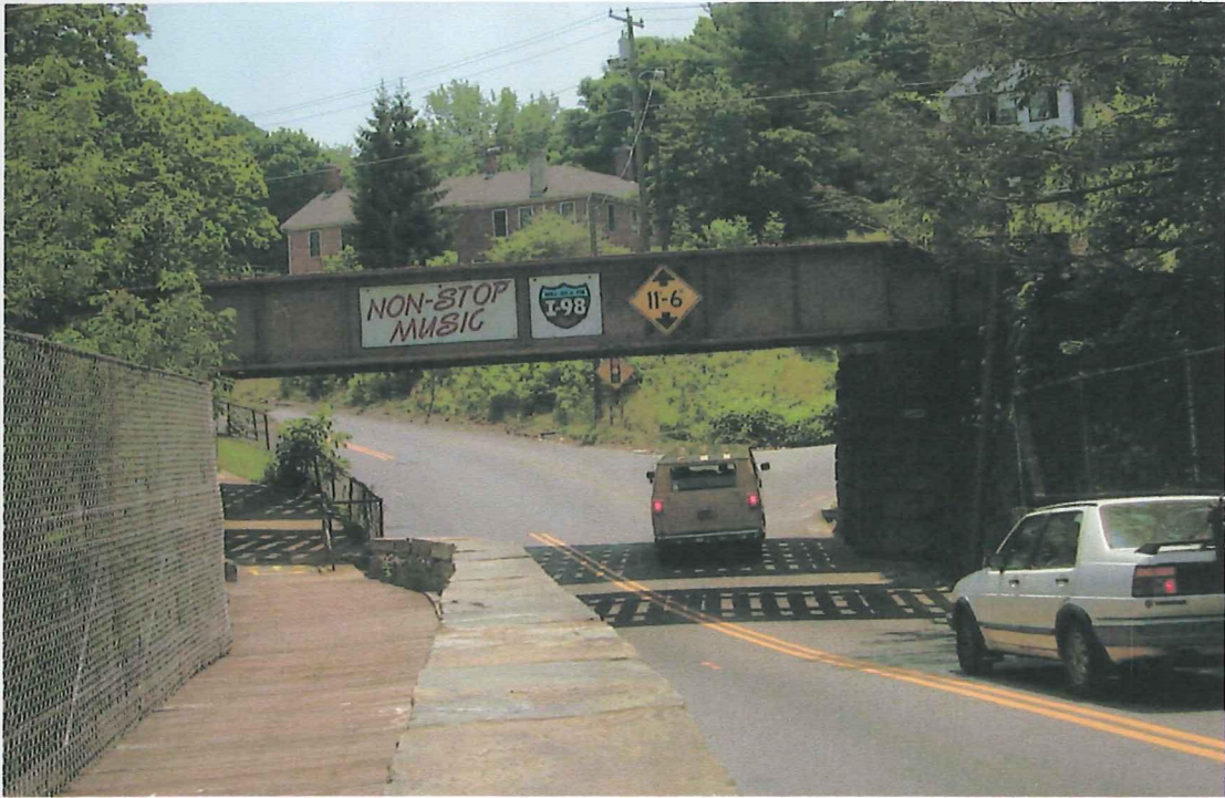
Bridge over South Main Street, Looking Southerly
