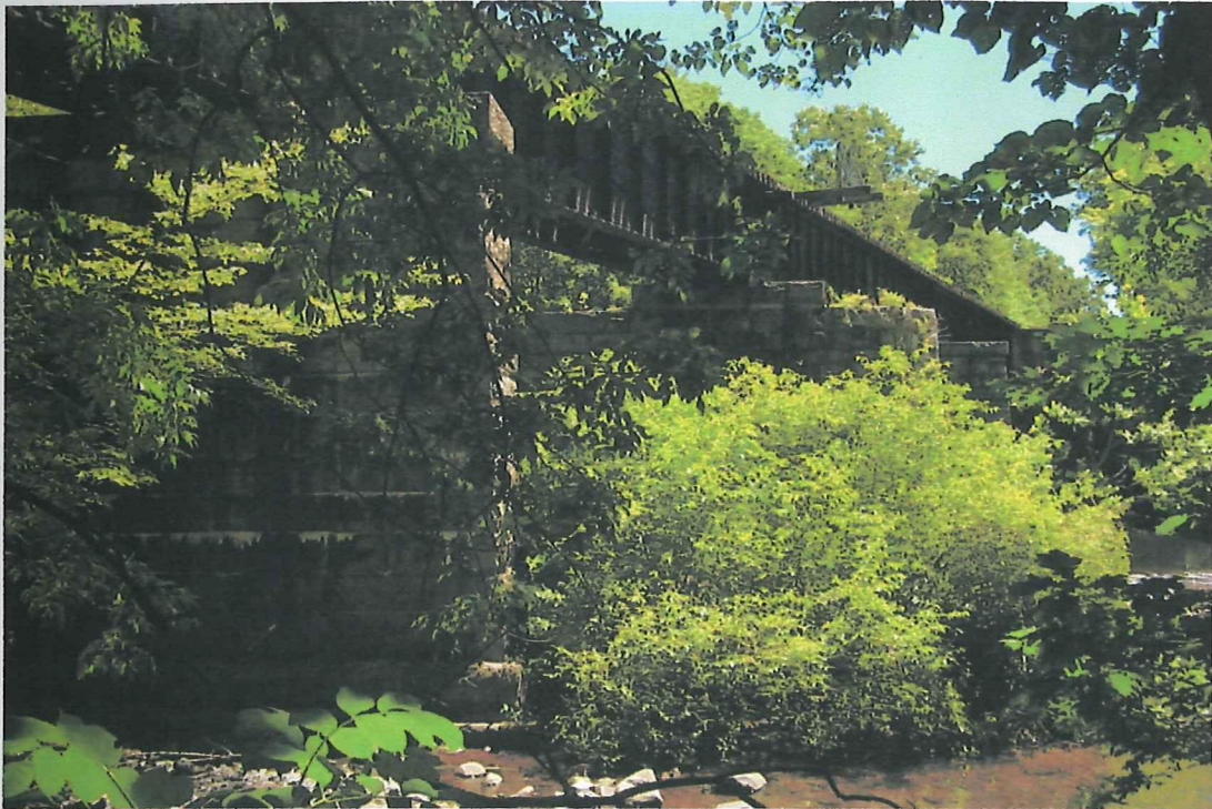
View of Span and Abutments, Looking Southeasterly
