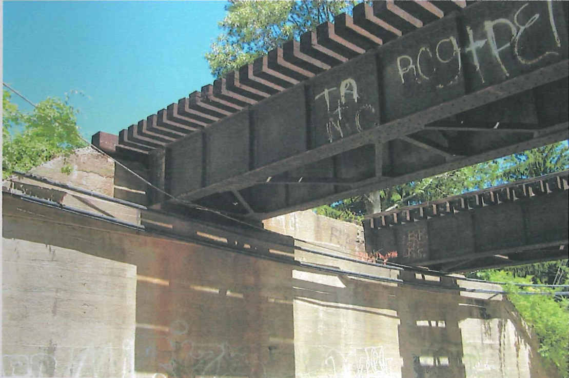
View Under Central Vermont Track, Looking North Westerly
