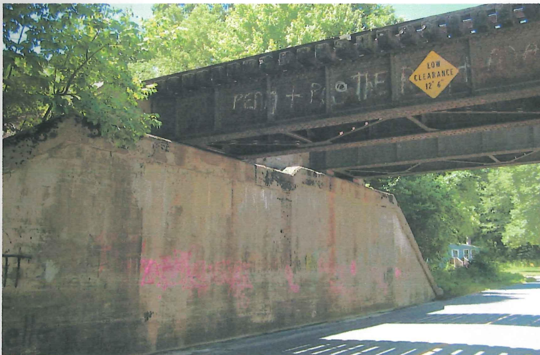
Southerly Abutment, View Under CDOT Track
