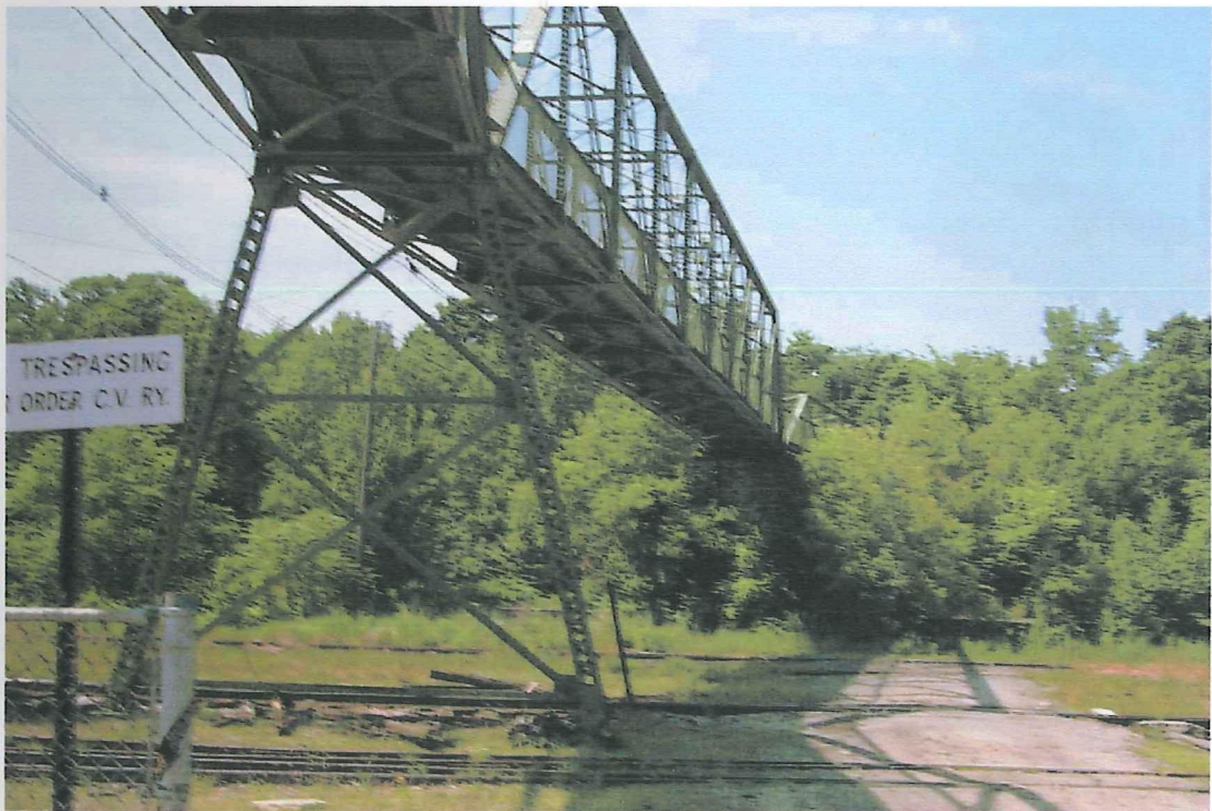
View Beneath Bridge Looking Southerly
