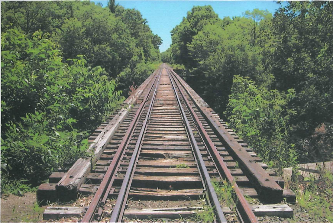
Top of Bridge, Looking Southerly
