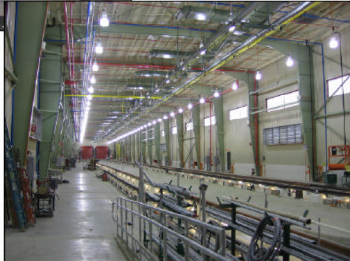
Connecticut Commuter Rail Running Repair Shop Constructed 2006 - New Haven
