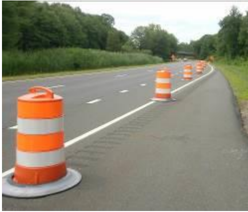
Start of lane closure on NB Route 9
