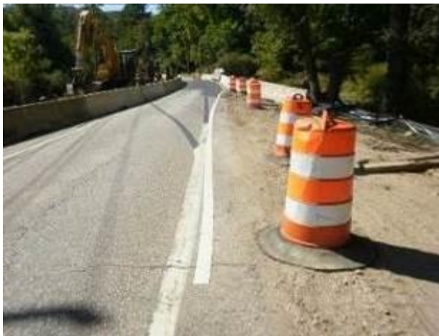
Eradicated and new pavement markings at work site.
