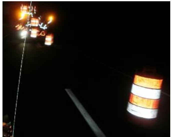
Traffic drums are placed for lane closure.
