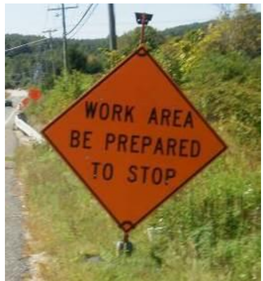
Additional signage provided by the contractor.
