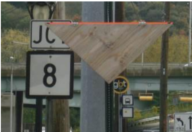
The “Right Lane Closed Ahead” sign is hinged to fold down when not in use.
