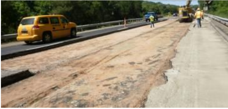
One lane traffic traveling through work site
