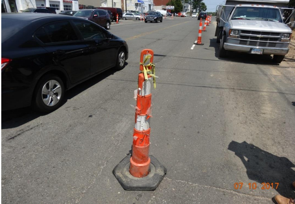
Photo 15: This cone has lost a significant amount of reflective material. Cones in poor condition should be replaced.
