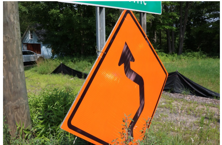
Route 74 WB: This ROAD WORK AHEAD sign is posted on waffle board which is not an acceptable material to use.
