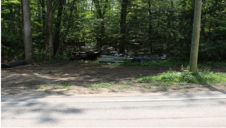
Photo 8: Here, materials are stored well outside the required clear zone of 16 feet off of the roadway.
