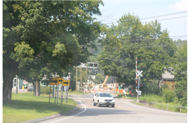
Phelps Way: The next advance warning sign about the road work ahead or a temporary signal ahead is only a few feet from the project site.
