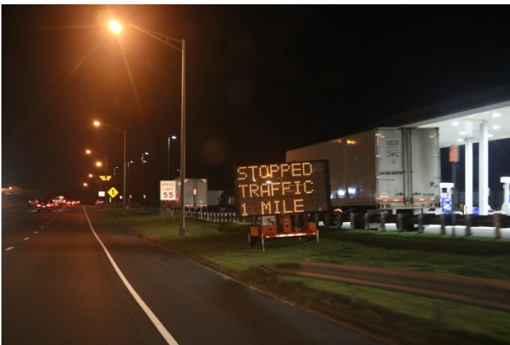
I-95 NB: A CMS a part of the PWZMS states BE PREPARED TO STOP, STOPPED TRAFFIC 1 MILE on two frames.
