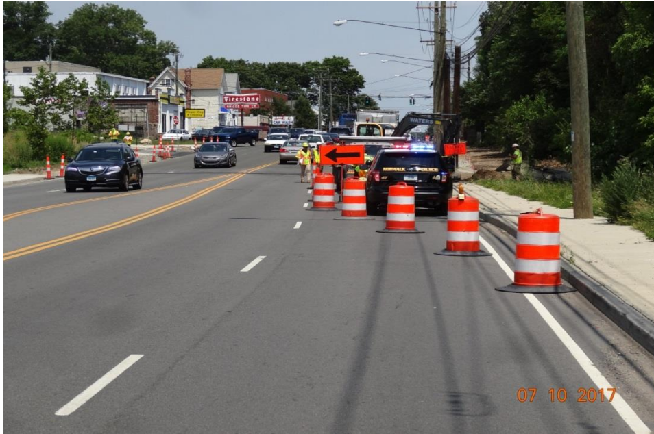
Photo 5: Route 1, NB approaching the tapered section. The warning lights on the barrels are unnecessary and may become projectiles if hit. If the warning lights were needed the attachment system would have to be submitted and approved by the Department. Also, the “Sidewalk Closed” sign should be accompanied by a Type 3 Barricade located just behind the sign.
