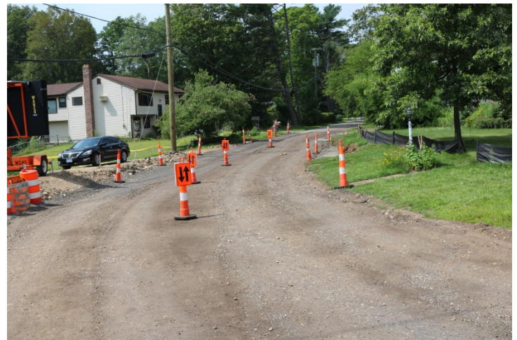
South River Road: The road is divided with bidirectional traffic signs in the center. Also, one of the CMS stationed on the left.
