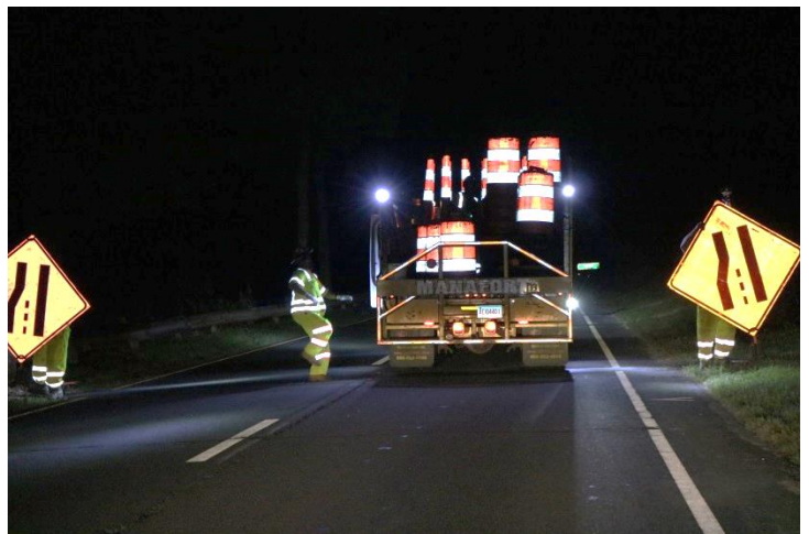
Route 15 SB: The last signs installed are the merge right signs.
