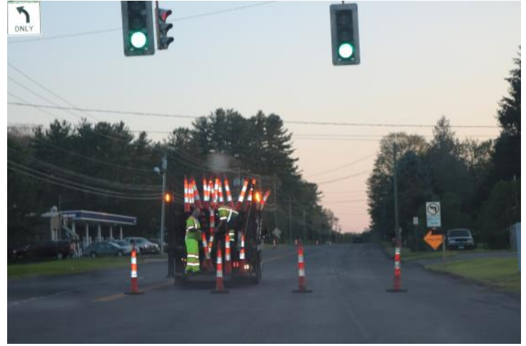
The crew closes off the WB lanes at the intersection.
