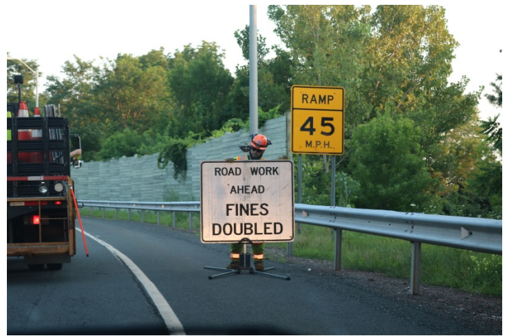
I-91 SB Exit 25: A FINES DOUBLED sign is installed on the on ramp.
