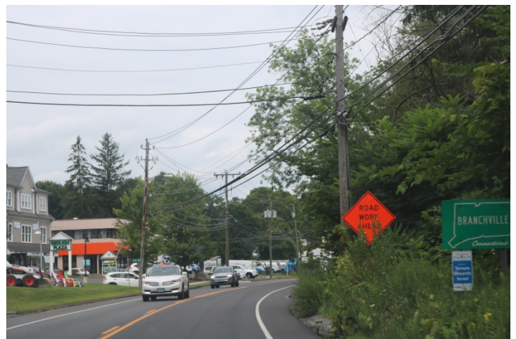
Route 7 NB: The next signs in the advance warning are post-mounted but tree or shrub growth has obstructed the messaging for the signs. Selective clearing will improve the visibility of the signs.
