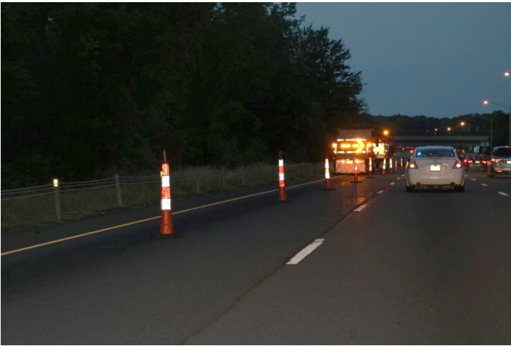
I-91 NB: The pattern is comprised of 42-inch cones which are preferable especially on the interstate. A TMA is within the taper and has an advance flashing arrow signaling to merge right.
