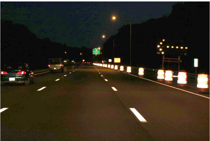
I-91 SB: A portable flashing arrow within the taper after dark is indicating to merge left.
