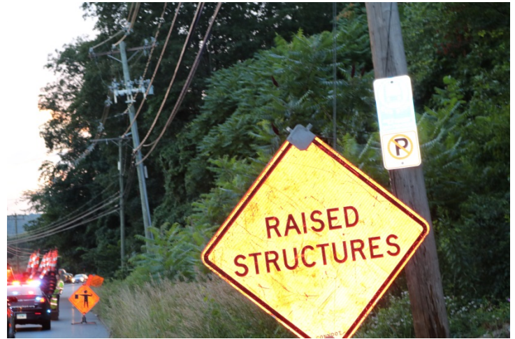
Route 63 NB: This RAISED STRUCTURES sign is in acceptable condition.
