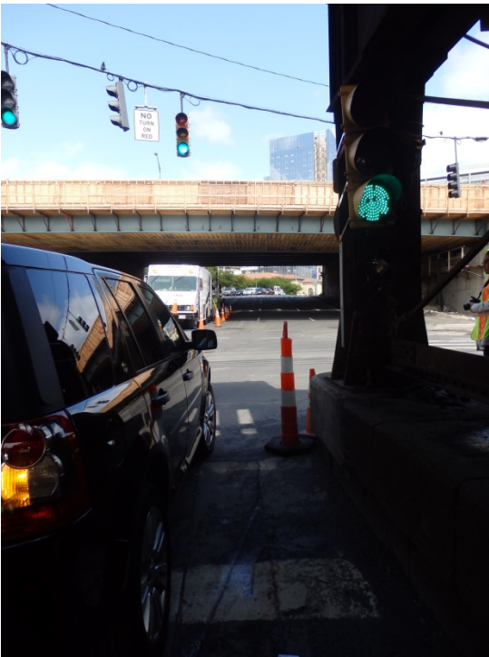
Atlantic Street: Here are the other temporary configurations of the traffic signals that are difficult to see from under the bridge.
