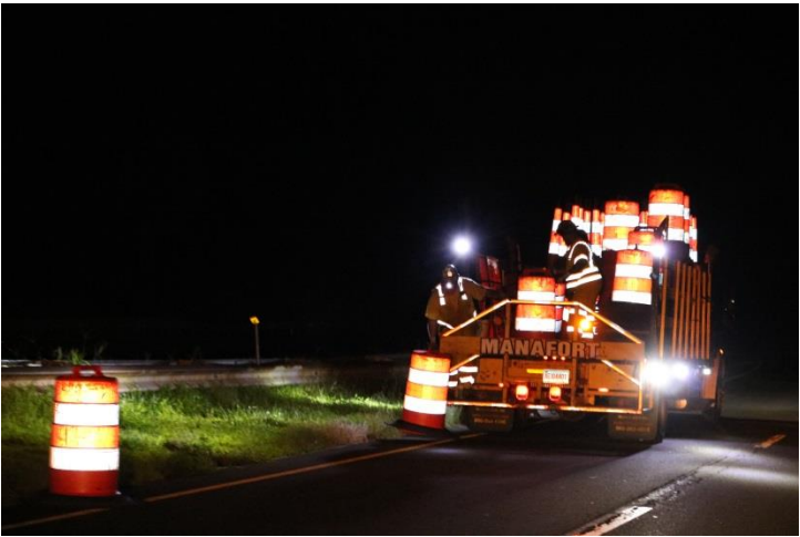
Route 15 SB: The taper is installed using traffic drums.
