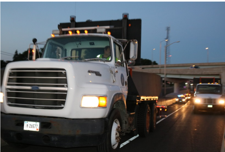
I-95 SB: The Rolling Road Block used while installing the pattern.
