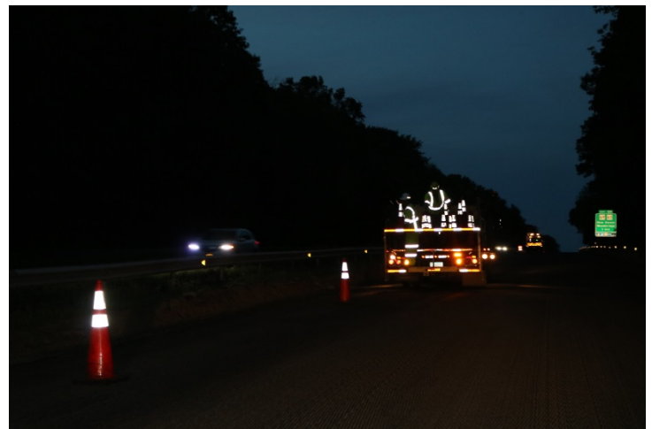
Route 15 NB: The tangential of the pattern being installed with 36 inch cones.
