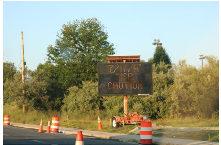
Route 6 EB: The only Changeable Message Sign for the project. Maintenance provided this and this is the only one they could procure. The sign's first frame: MILLING & PAVING STARTING, the second frame: 7/17/17 USE CAUTION.
