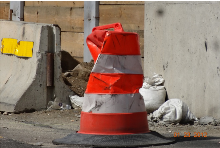
I-95 Exit 8 Off Ramp: This traffic drum is terribly misshaped and needs to be replaced.
