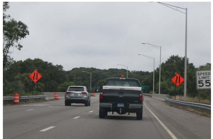
I-95 SB: The last advance warning signs are the merge right chimney signs.
