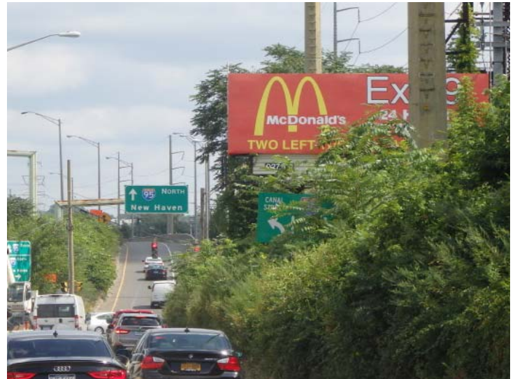
South State Street: A sign to indicate direction of the lanes at the next intersection needs vegetation clearing in front. The sign indicates there are three lanes: left turn lane, through lane, and a through and right turn combo.
