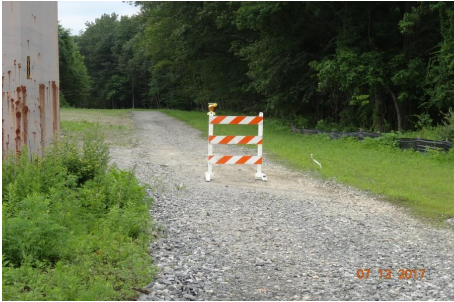
Photo 2: Type 3 Barricade installed to help prevent vehicles and pedestrians from proceeding any further.
