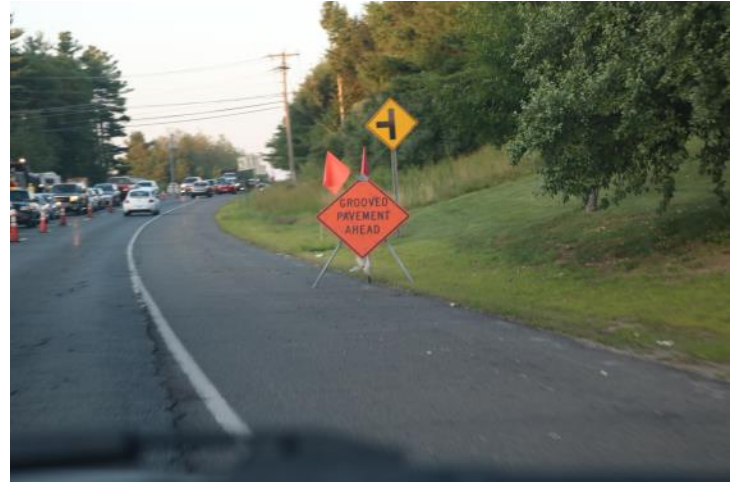
Route 6 WB: Signs are placed to inform the motorists of the temporary road way condition. This one states GROOVED PAVEMENT AHEAD.
