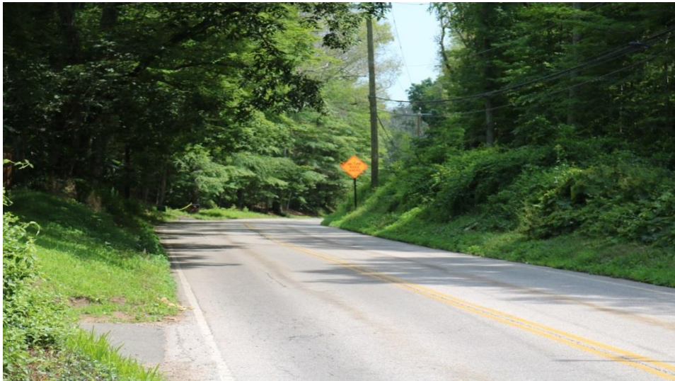
Photo 1: Photos 1 and 2 show permanently mounted construction signs were well placed in areas with good sightline for drivers.
