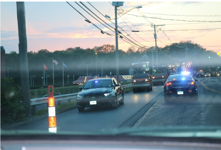
Route 63 NB: The equipment mobilizing to the work area.
