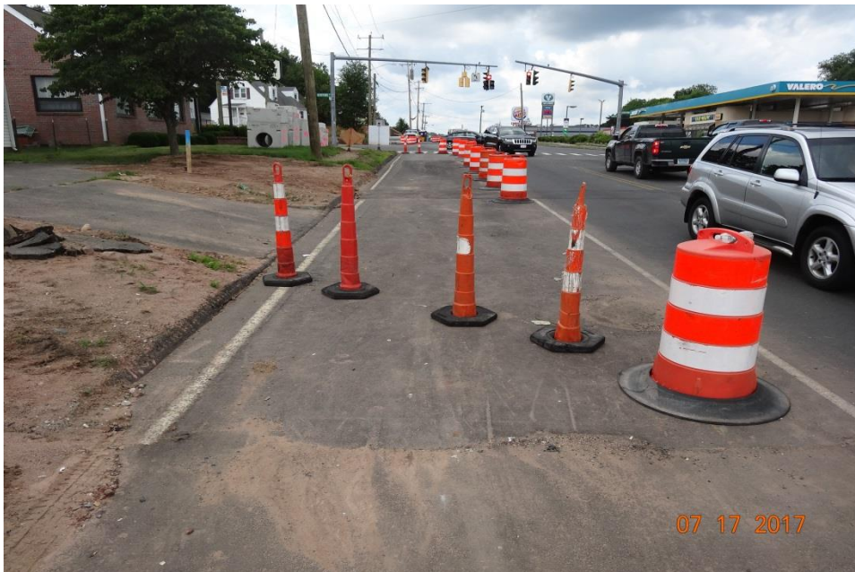
Photo 16: Cones that do not meet the reflectivity requirements need to be removed from the project and replaced with cones in good condition.
