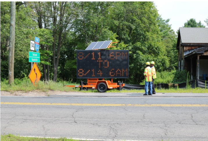
Route 74: Another CMS, just east of the project, is off the road and currently not being used but will inform motorists of the weekend closure. The two frames stating "Route 74 EB to Be Closed 8/11 6PM to 8/14 6AM".
