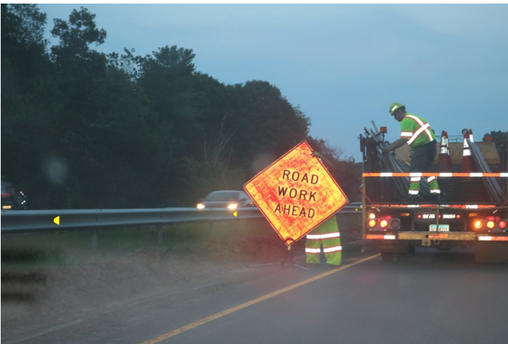
Route 15 NB: Another construction sign stating ROAD WORK AHEAD.
