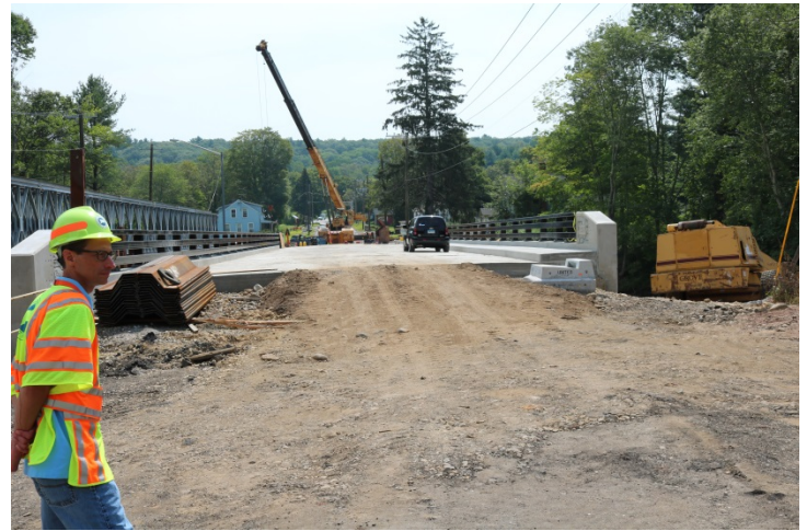
Route74 (Tolland Stage Road): The new bridge being built.
