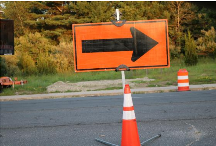
Another arrow sign was installed the end of a business driveway to inform motorists they can only turn right when proceeding out.
