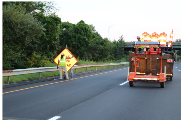
I-91 SB: The first temporary sign installed is ROAD WORK AHEAD.
