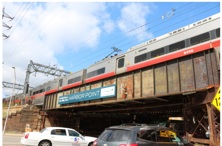
Atlantic Street: The Metro-North Railroad bridge overhead
