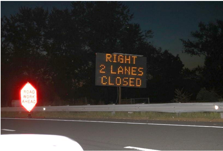
I-84 WB: A Changeable Message Sign stationed before Exit 50 states RIGHT 2 LANES CLOSED.
