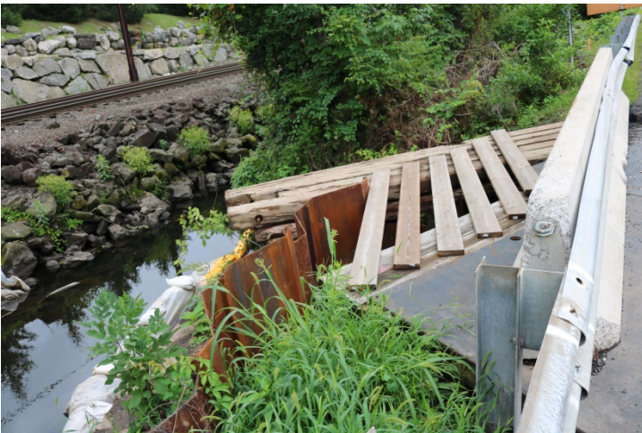
The temporary sheet piling on the east side of the bridge
