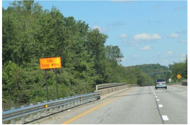
I-395 NB: The post-mounted END ROAD WORK sign.
