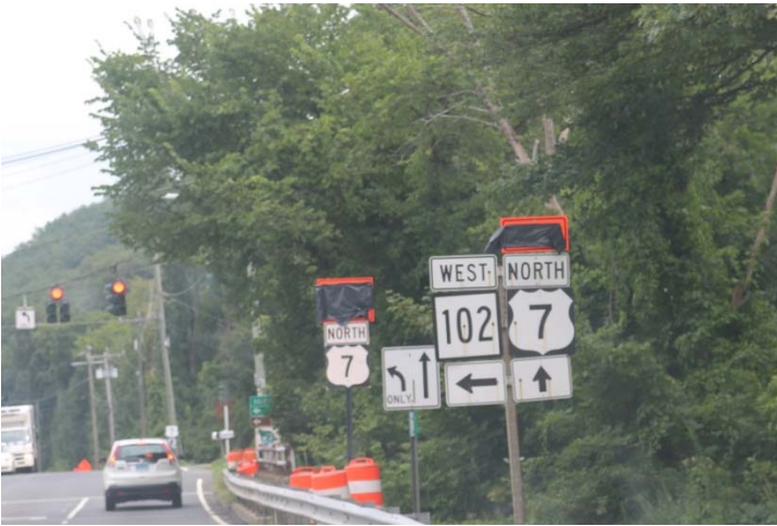
Route 7 NB: More detour signs that are posted on existing sign posts are covered during the week.
