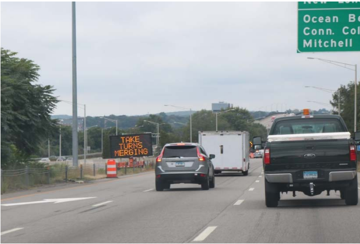
I-95 SB: Another CMS is located in the shoulder of the median. It states "TAKE TURNS MERGING" on its first frame.
