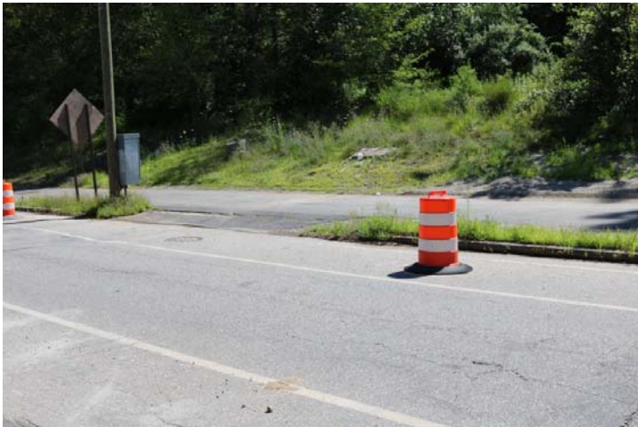
Tracy Road: An existing ramp for the multi-use path.
