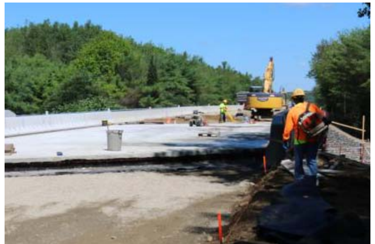
I-395 NB: The work zone over Tracy Road.
