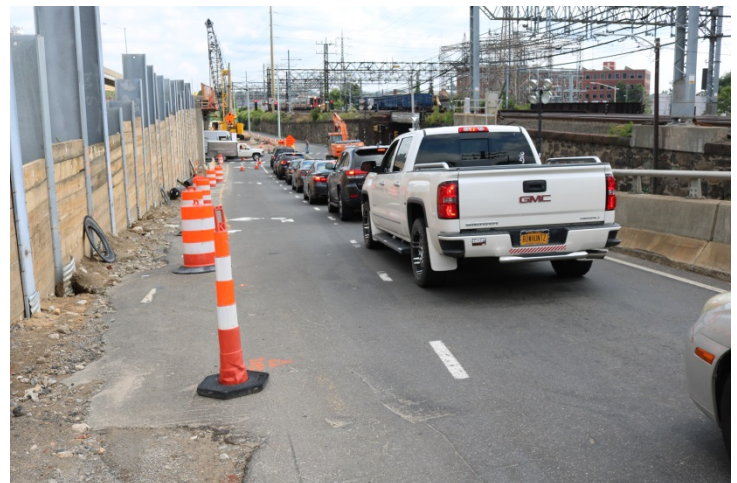
I-95 Exit 8 Off Ramp: The left turn lane is only closed at the end. The lane closure should have started farther back to prevent vehicles from entering the left turn lane.
