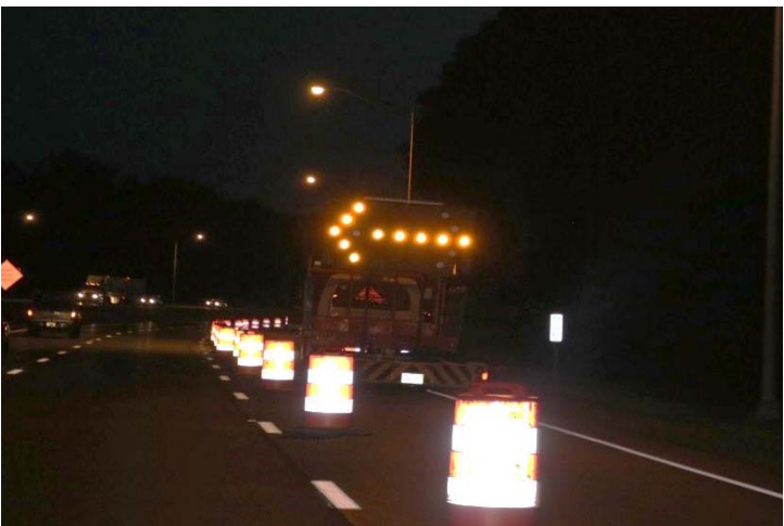
I-91 SB: A TMA within the taper has a flashing arrow indicating to merge left.
