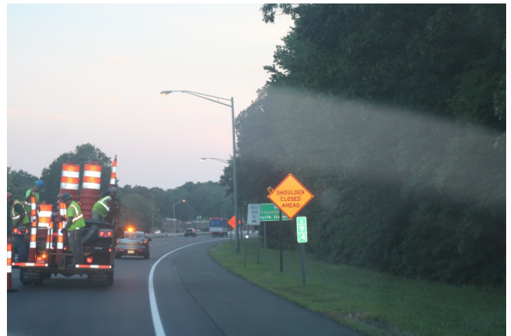
I-91 SB: A post-mounted SHOULDER CLOSED AHEAD sign has a warning light attached.
