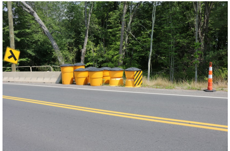
This impact attenuation system is the only one with a Sign No. 50-5032 at the nose.
