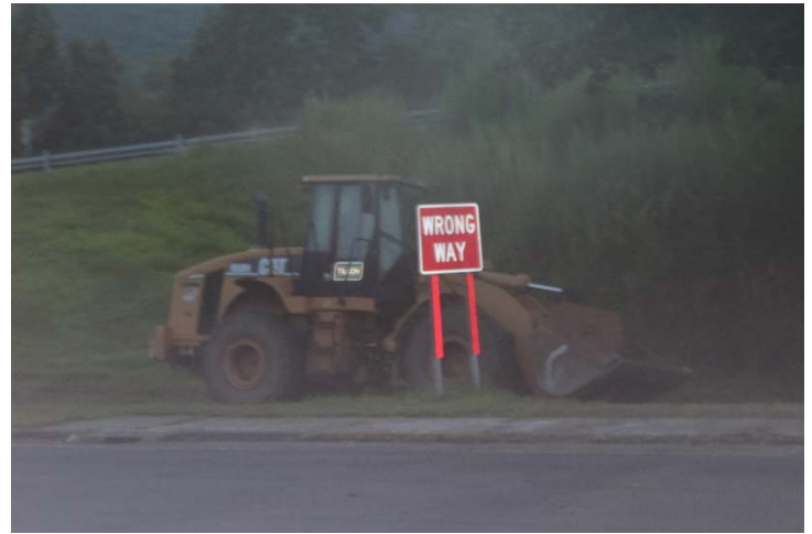
Route 63 NB: Equipment in the staging area off Route 8 Exit 26.
