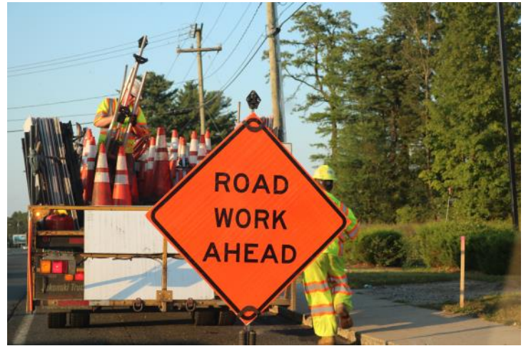
The next temporary construction sign is ROAD WORK AHEAD.
