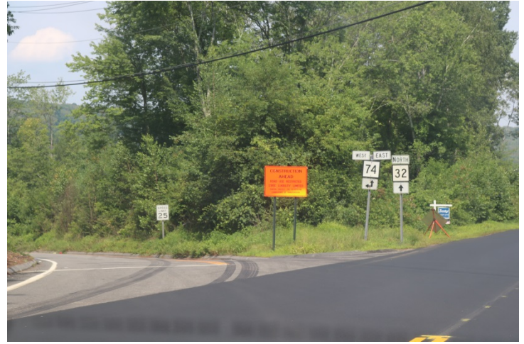
Phelps Way: The only sign in advance of the project on this road is a legal sign. There was no sign warning about the temporary signal.
