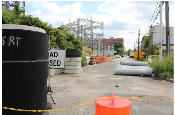
Manhattan Avenue: Material storage area
