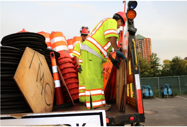
The construction signs are mounted on plywood which is an acceptable material to use.
