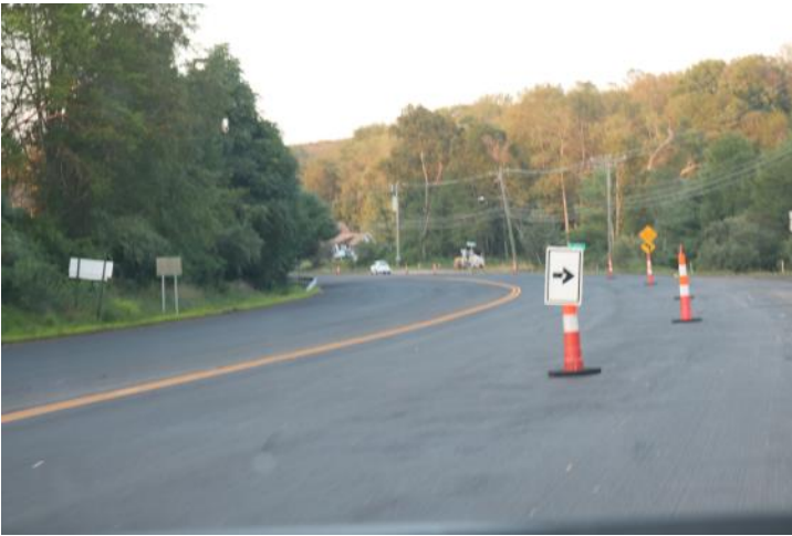
Route 6 EB: This pattern uses little arrow signs mounted on the traffic cones just after an intersection.
