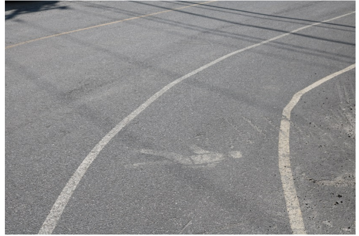
The pedestrian path has been painted in NCCC's parking lot to detour pedestrian traffic around the site. The markings need its paint refreshed.
