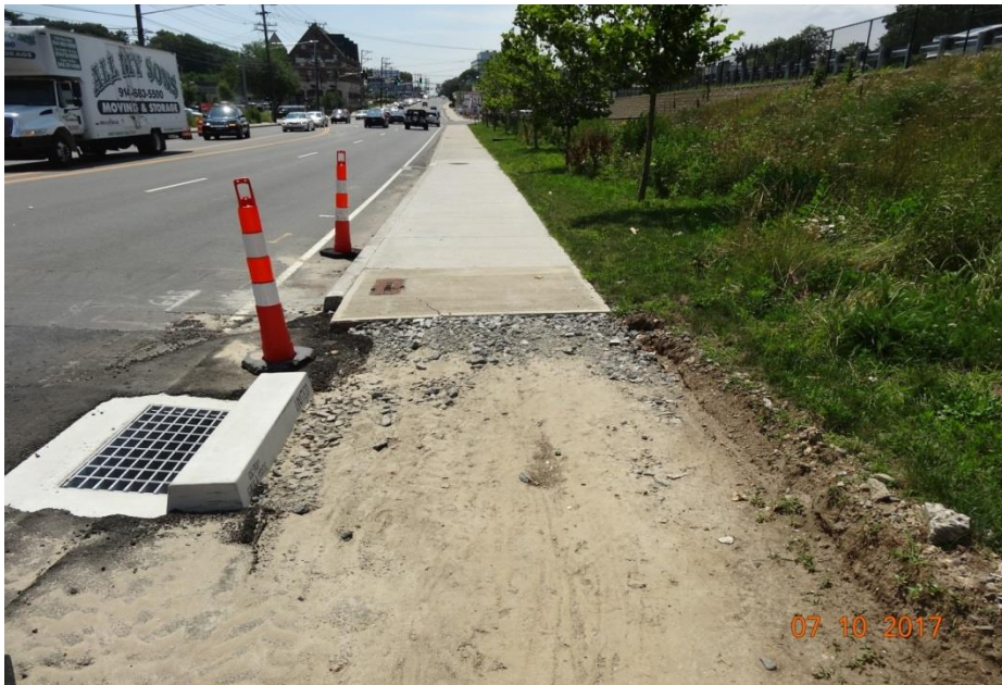
Photo 8: Showing the southern end of the same sidewalk as in Photo 7. The crushed gravel ramp formed at the transition is approximately 6 inches high by 12 inches long. The existing sidewalk condition has not been matched or made better at this location.
