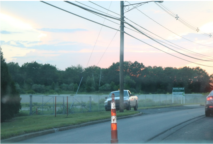
Route 63 NB: Some of devices need replacing like the cone above.
