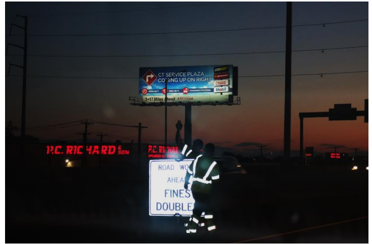
I-95 SB: The first sign installed is a FINES DOUBLED sign.
