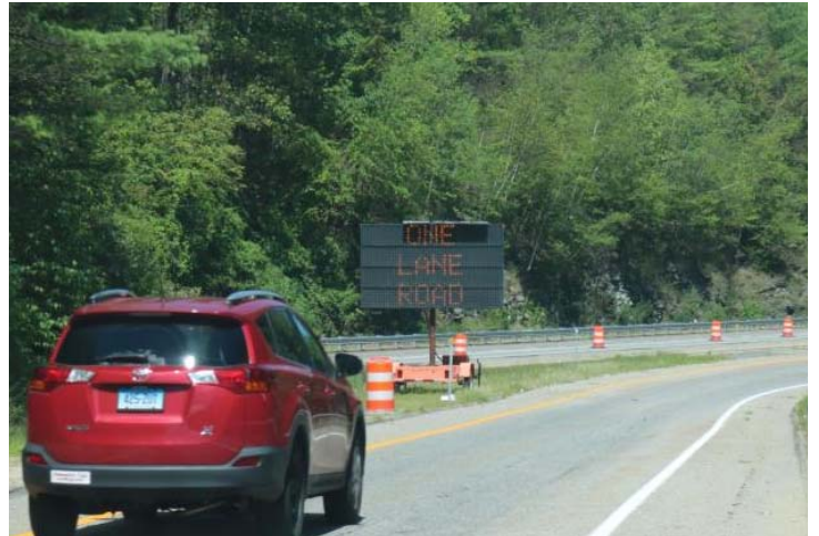
I-395 NB, Exit 94 On-Ramp: The first frame for the CMS states "ONE LANE ROAD". The lighting on the CMS appears too dim for daylight but the message is still readable as a motorist moves closer to the CMS.
