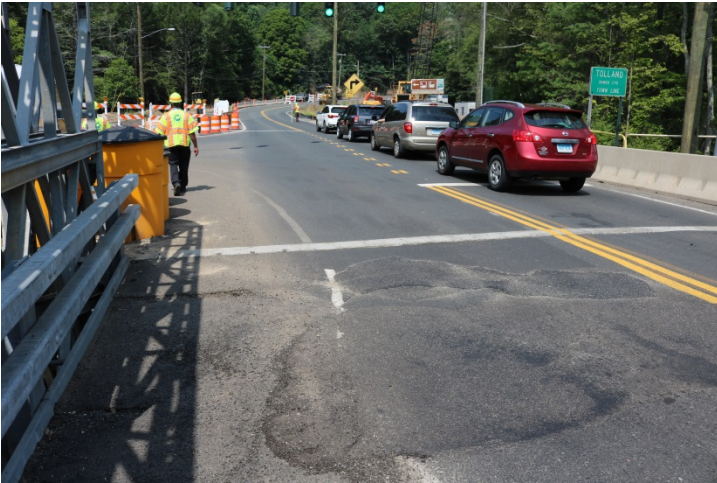
Route 74 WB: There is delamination of the pavement on the eastbound side although that side doesn't stop at the light on the bridge.
