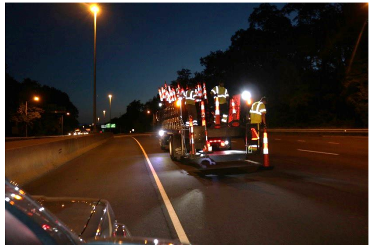
I-95 SB: The sign crew started the tangential to the pattern using traffic cones.
