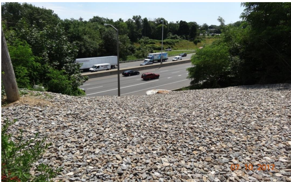
Photo 12: Showing the slope (in photo 11) down to the I-95 right of way.
