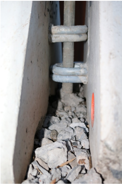
Some of the TPCBC sections had pins that were not fastened on the bottom.
