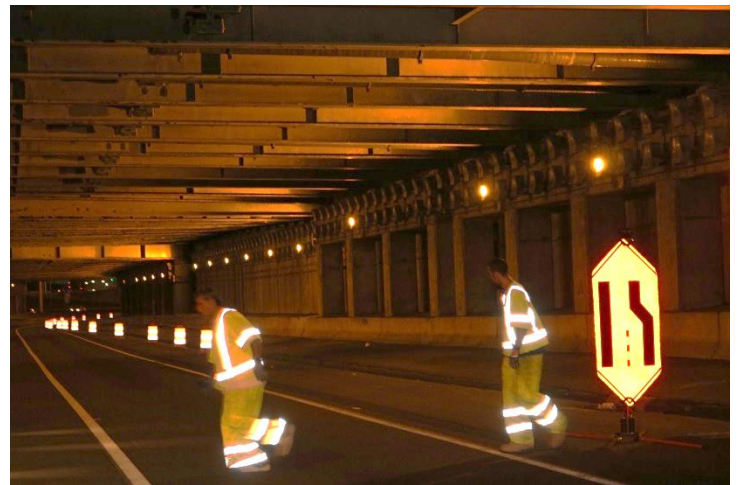
I-84 WB: A merge left sign is mounted within the tunnel. The sides are cut off to prevent it infringing into the lanes.
