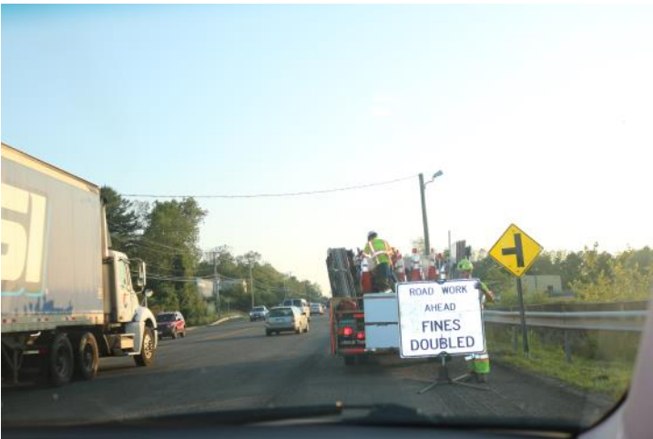
Route 6 WB: The first sign placed is the FINES DOUBLED sign. The traffic is still proceeding in their usual lanes.
