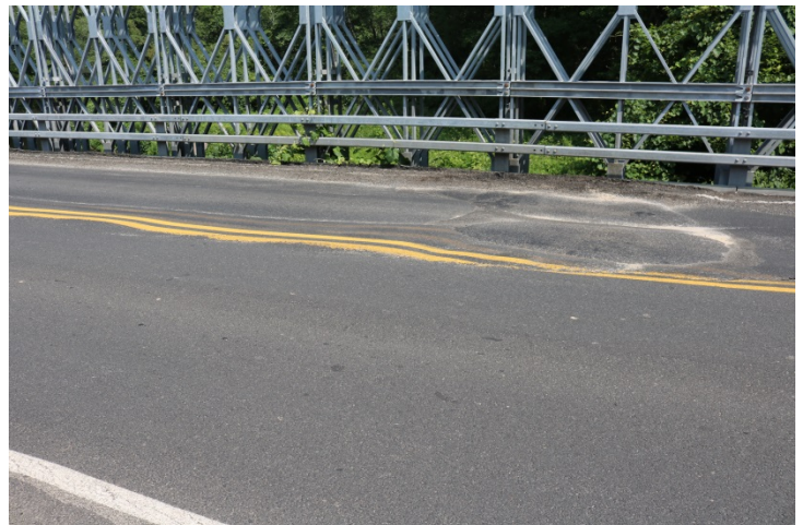
The shovelled pavement on the temporary bridge.
