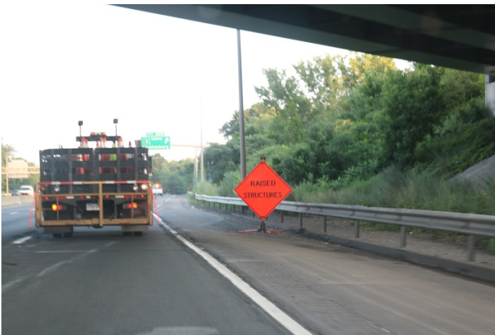
I-91 SB: Although this is a temporary construction sign, it stays in place through day to inform motorists of the roadway conditions that may be exposed from shift to shift like RAISED STRUCTURES.
