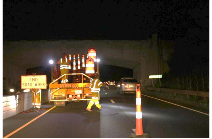
Route 15 SB: The END ROAD WORK sign installed.
