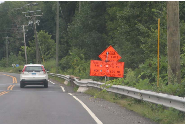
Route 7 NB: This sign states what dates the bridge on Route 7 will be closed and the detour in effect. However, the message is too long and lettering too small for motorists to read the message.
