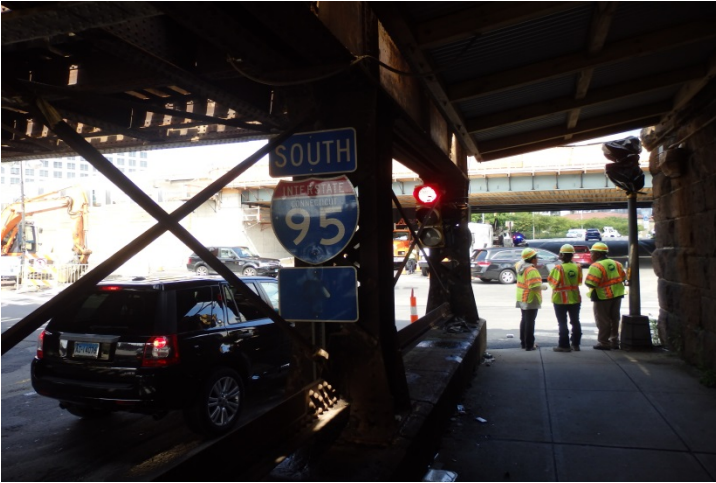
Atlantic Street: Here is the additional temporary signal that was installed to help with the poor sightline under the railroad bridge.
