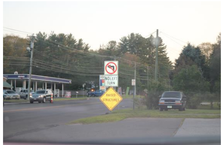
Route 6 WB: This sign (RAISED STRUCTURES) is mounted too low. It may be more convenient to mount on posts already placed but the height of the sign still needs to be high enough to catch a motorist's attention.
