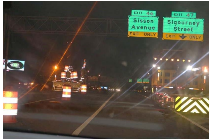
I-84 WB: Exit 47 to Sigourney Street is closed by a crash truck. It has a straight bar flashing arrow showing the lane is closed. The sign crew is installing traffic drums to close the off ramps.
