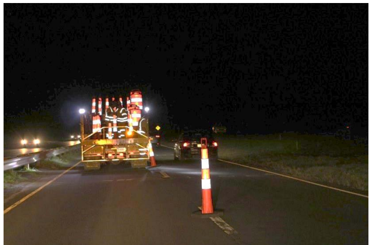
Route 15 SB: Traffic is let go after the Rolling Road Block.
