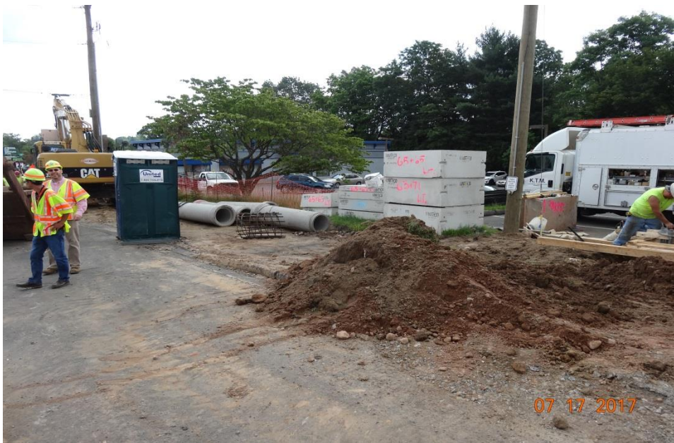
Photo 14: An example of construction equipment and materials being stored well outside of the roadway clear zone.
