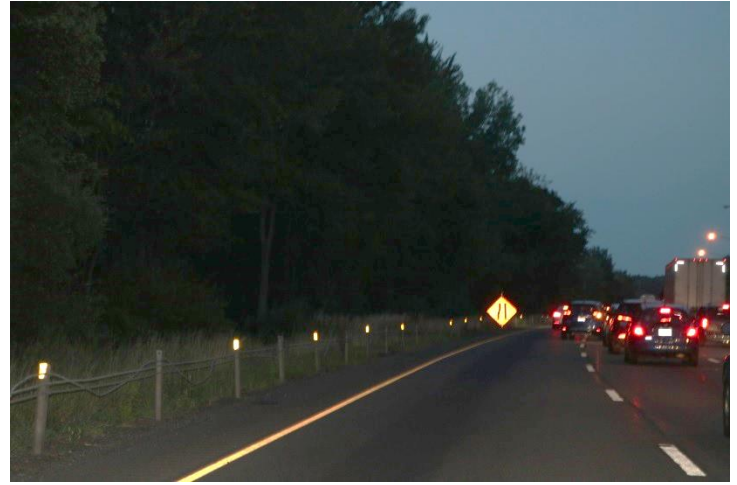
I-91 NB: A merge right depiction sign only on the left side of the road. None was placed on the right side of the roadway.
