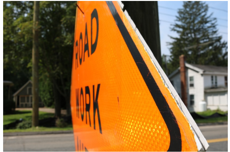
Route 74 WB: This ROAD WORK AHEAD sign is posted on waffle board which is not an acceptable material to use.
