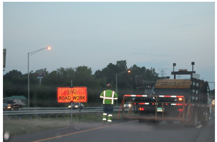
I-91 SB: The END ROAD WORK is installed around Exit 24.
