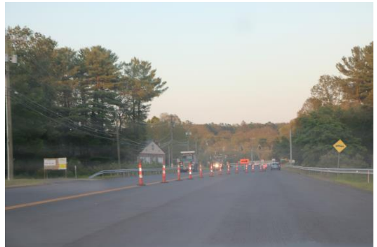
Route 6 WB: The other operation further down Route 6 in Chaplin, the traffic is shifted to the EB side as well. This pattern uses the taller 42-inch cones.
