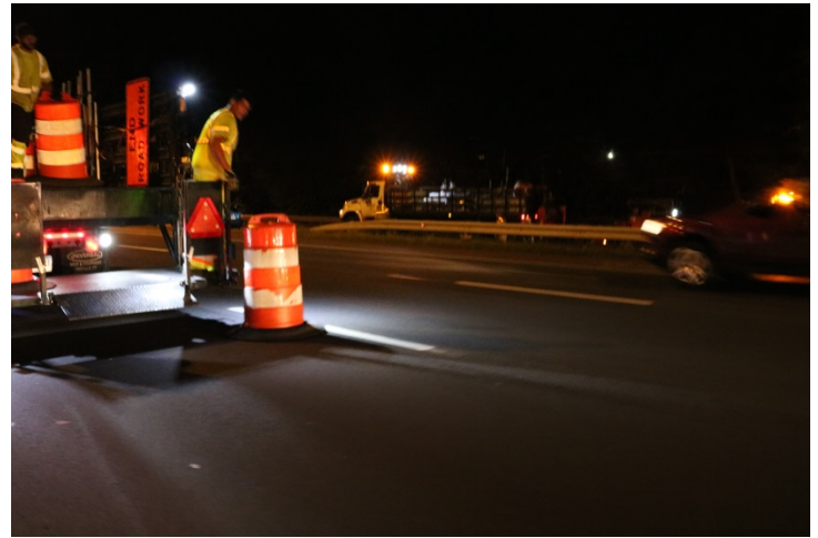
I-95 NB: This traffic drum is missing reflective tape and is marginally acceptable.
