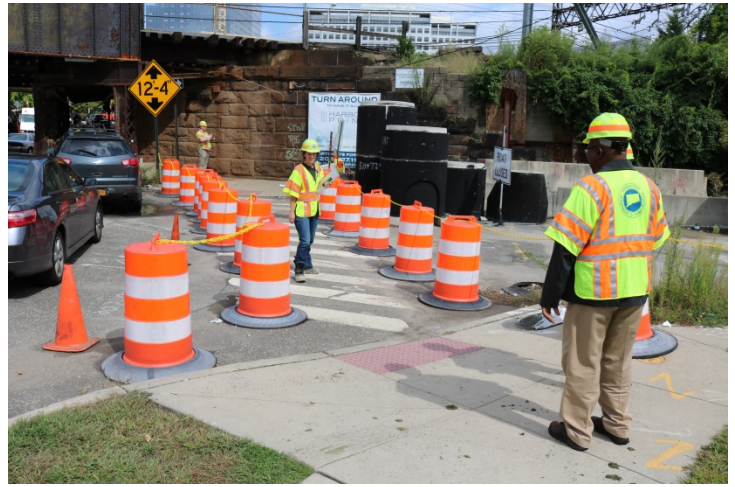
Atlantic Street: Traffic drums delineate the pedestrian cross walk on Manhattan Avenue since the road is closed.
