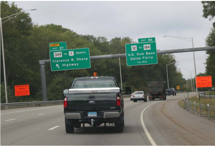
I-95 SB: The post-mounted construction roadway liability signs on both sides of the roadway
