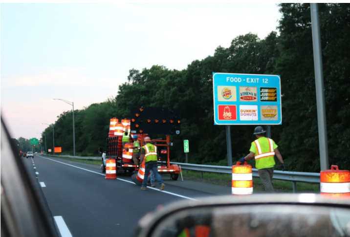
I-91 SB: A flashing arrow is installed in the taper.
