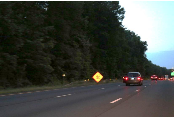
I-91 NB: The advance warning signs starting the northbound side.
