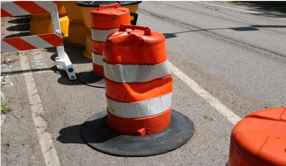
Photo 5: Any damage that may affect a traffic control device's ability to reflect light should be repaired or replaced.
