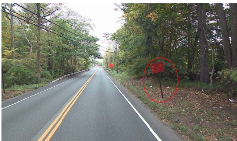
Signs left from a previous project that should be removed. See Finding #5.
