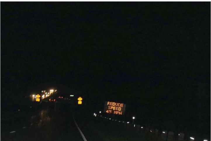
Route 15 SB: Before the pattern near Exit 40, a Changeable Message Sign displays two frames: LANES CLOSED AHEAD, REDUCE SPEED TO 45 MPH.
