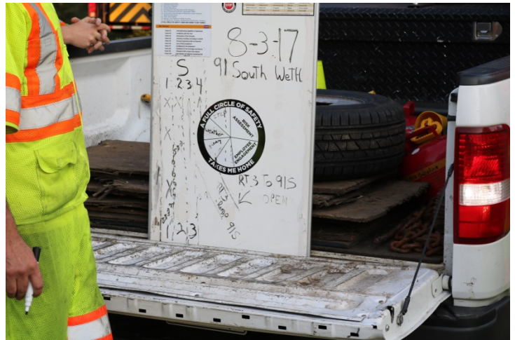
The Contractor's Supervisor draws out the traffic pattern to be installed that shift.
