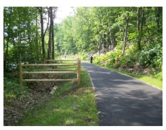
**Burlington – Project 20-107**. *(Constructed 2015)*. This project recently reconstructed a section of the Farmington River Greenway from Arch Street southerly for a distance of approximately 9,300 linear feet. The location is intended to be an example of a trail maintenance project that fully reconstructed the 15 year-old surface which was in poor condition because of tree root (Black Locust) damage. Construction was substantially completed in June 2015.
