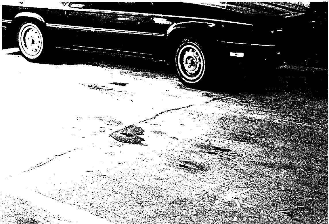
Typical crack location on floors. (Sealed with joint sealant and water tight)
