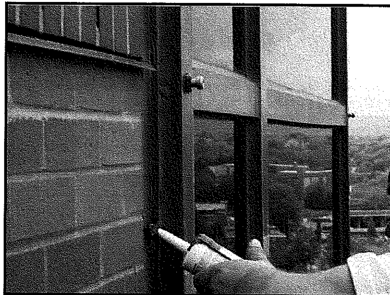
#9 Sealant repairs being performed at junction of curtain wall to masonry.
