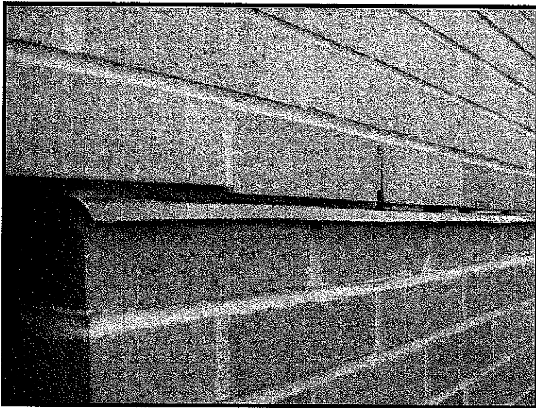
#8 New metal drip edge installed during recent masonry repair.
