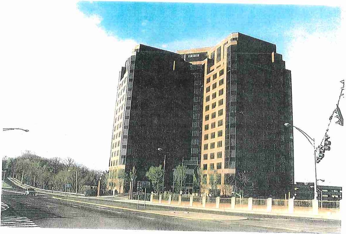
Photo No. 1 FRONT (NORTH/EAST) ELEVATION.
