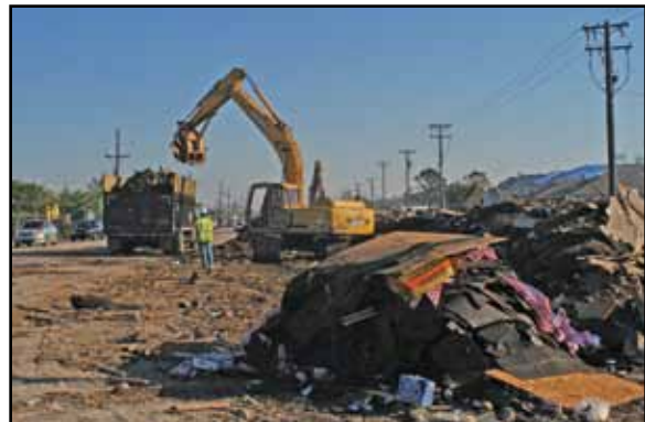
Figure 1: Contractor debris operation
