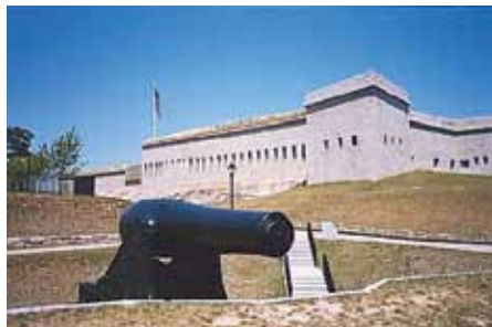
Opened in 2000, Fort Trumbull State Park today features the refurbished pre-Civil War granite-block fort, a world class, state-of-the-art visitor and interpretive center, and public-access saltwater fishing piers.
