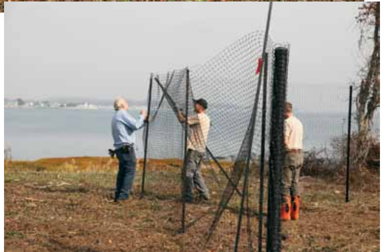
Deer-proof fencing was placed around planted areas on Charles Island.
