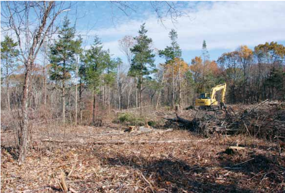
An excavator with a specialized mulching head (Denis Cimaf) also was used to clear trees from the site. Select trees, like apple trees, were retained to provide food and cover for wildlife.
