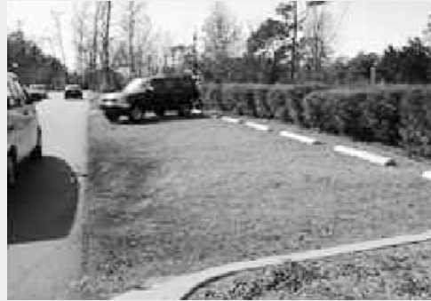
Parking Lot with Porous Surface
